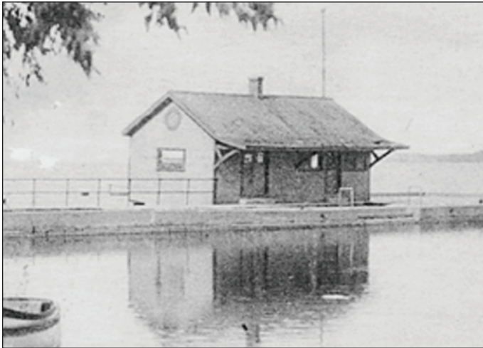
The dockhouse at the end of the Port Perry government wharf.
