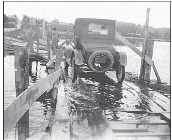
Temporary detour along a rickety floating bridge whil construction takes place along the causeway
