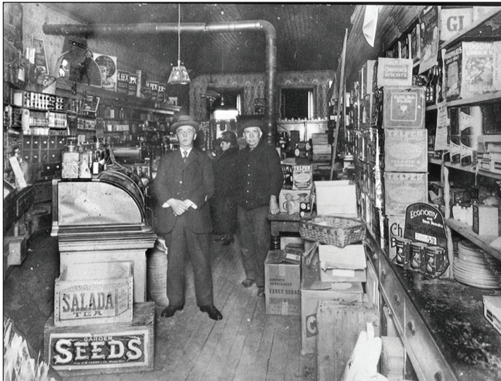
Interior of Thomas Widden's store, Queen St., Port Perry, 1922.
