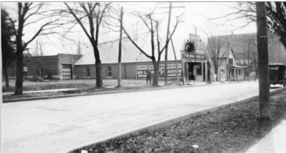
A section of the new Port Perry cement road, looking west towards the United Church, 1925.
