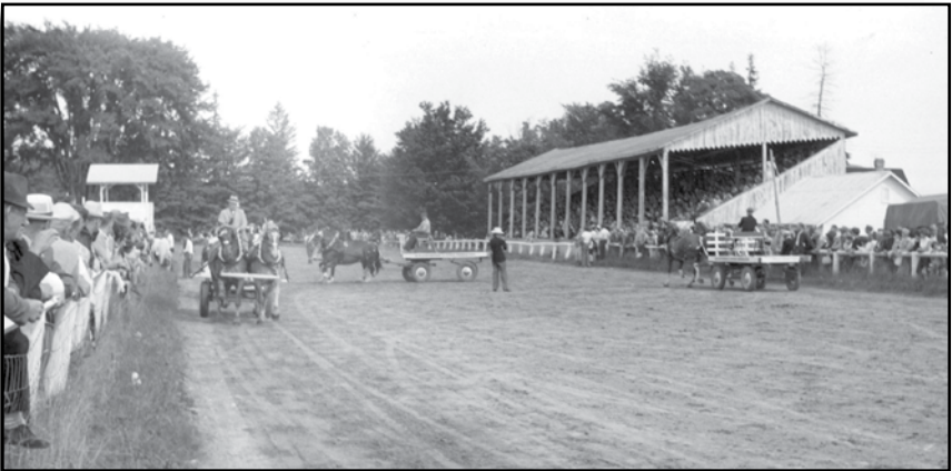
The last known picture taken of the former grandstand, which was destroyed in 1967
