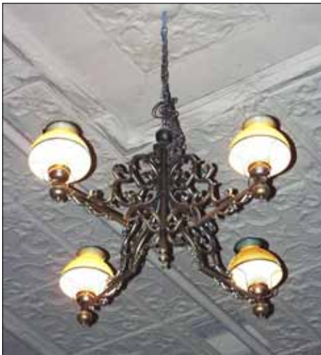
Period light fixtures upgraded with electricity.
