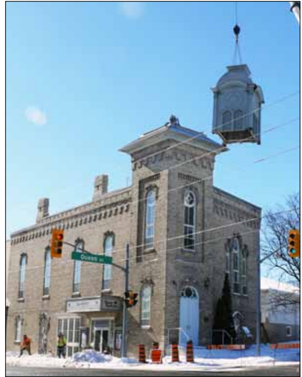
Up, up and away! Town Hall 1873 bell tower was detached and lowered to the ground for repairs on February 28, 2019.
