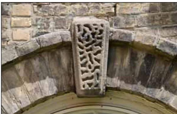
Decorative cement keystone over one of the windows.
