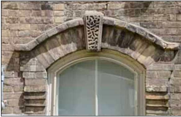
Decorative brick detailing around the windows.
