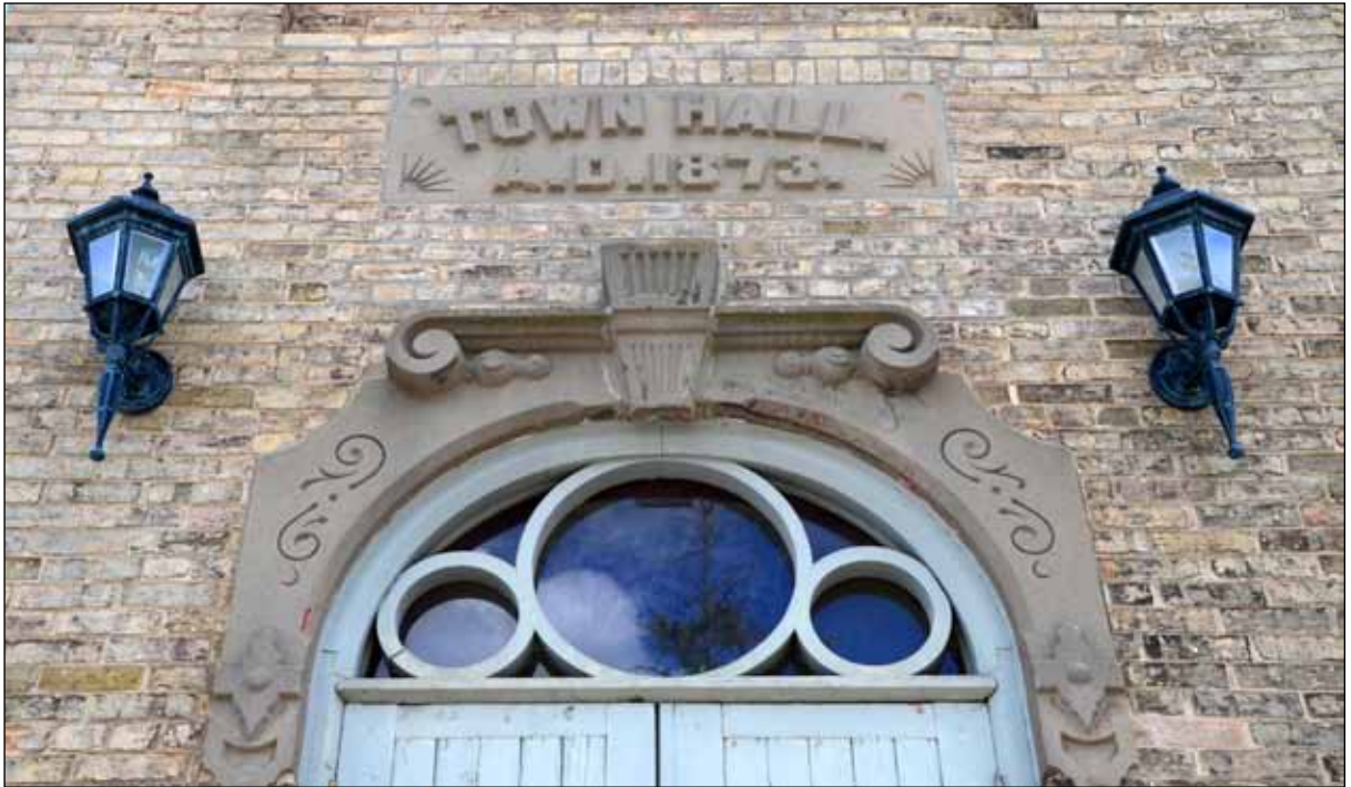
Decorative transom over front door of Town Hall 1873.
