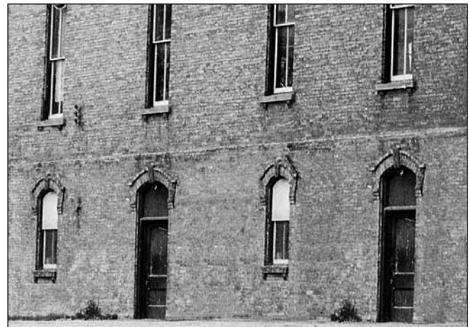
As near as can be determined, this picture shows what the lower east side of the Town Hall looked like before the large doors were cut into the brick to allow storage of the town's fire truck. Note: this is an illustrated picture, using photoshop to insert one window and one door where the two large openings were created.
