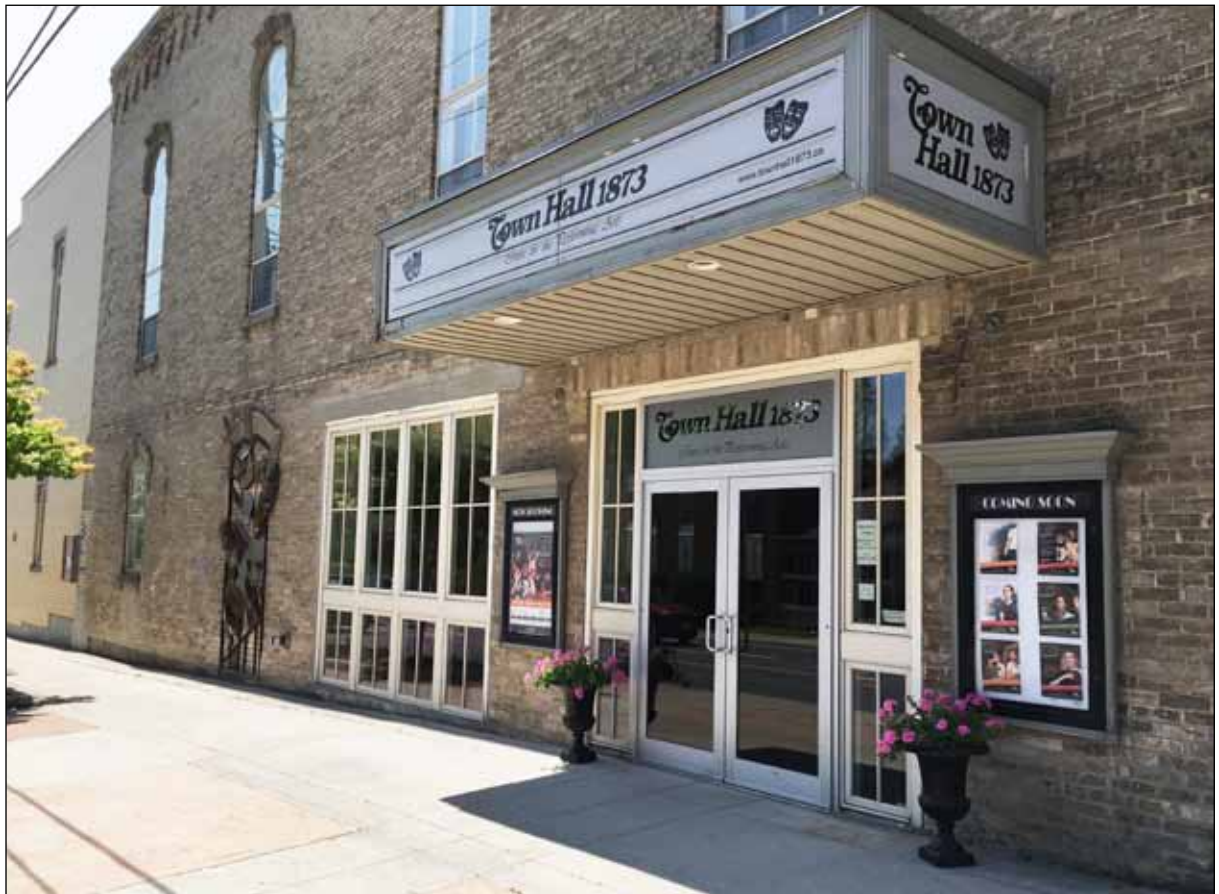
Above, the east side of Town Hall now has large windows and an attractive entrance to the hall, where there once was two large wood doors for the fire department.
