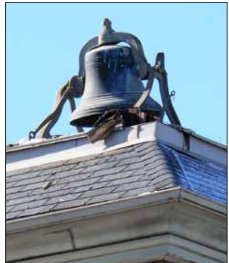
The Town Hall bell, installed about 1888, was visible for a short time after the tower was removed. It has since been put into storage.
