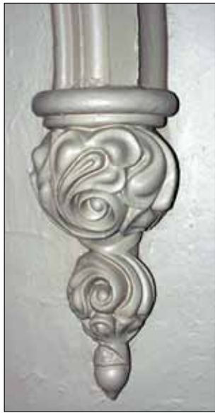
Ornate plaster mouldings.
