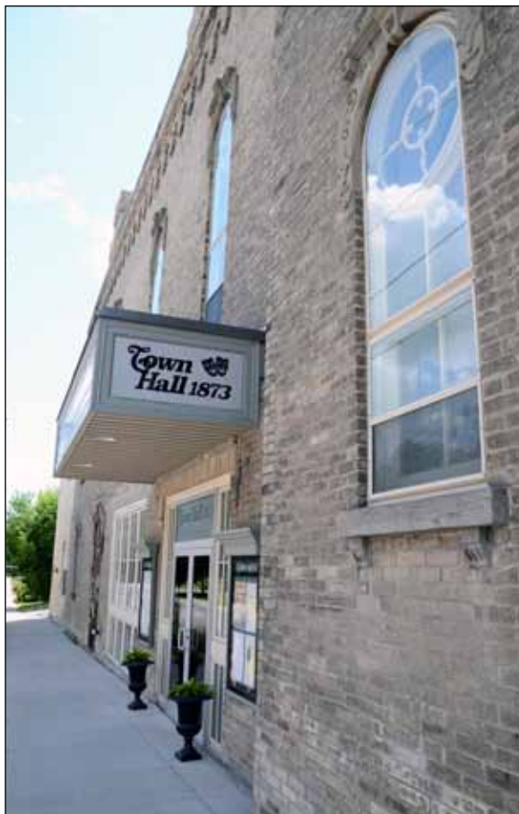
East side entrance to the theatre of Town Hall 1873.
