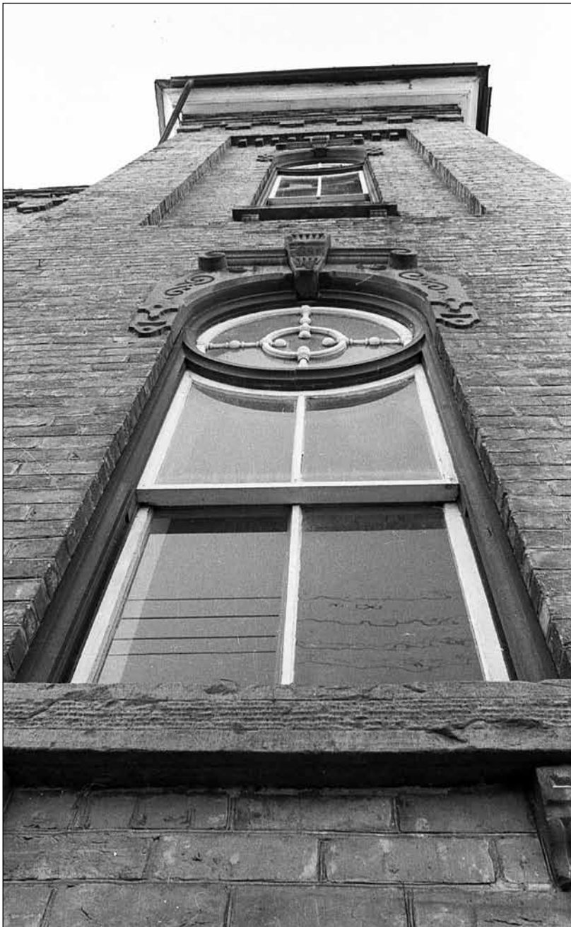
Decorative window at the bottom of the tower in March 1975.
