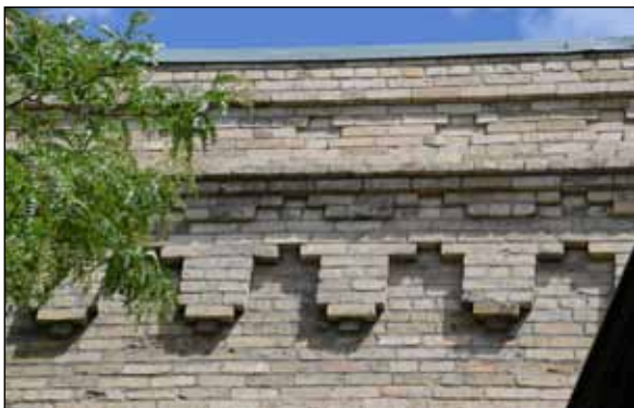
Intricate brickwork below the Town Hall parapet.
