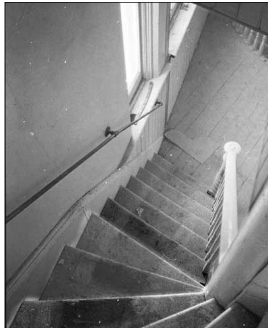
Staircase looking down from balcony.
