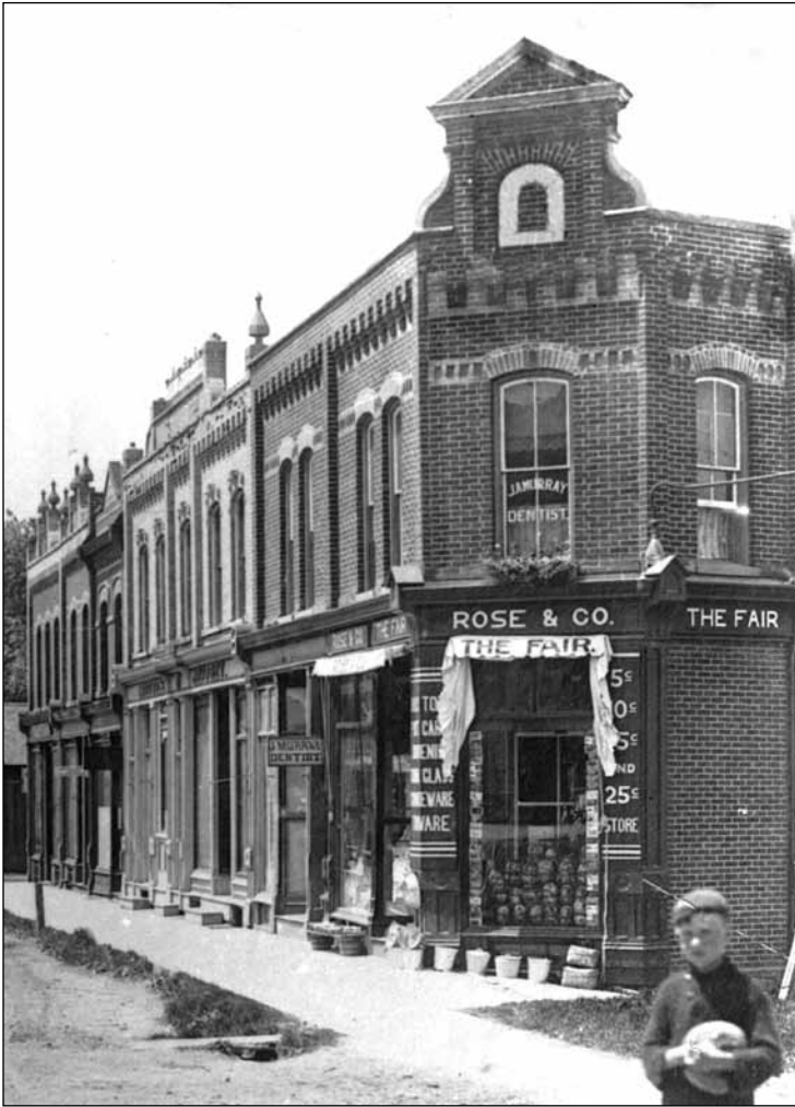
Buildings on the northwest corner of Queen and Perry Street.
