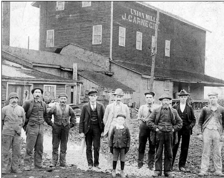
James Carnegie's Union Mills, near the waterfront, Port Perry.
