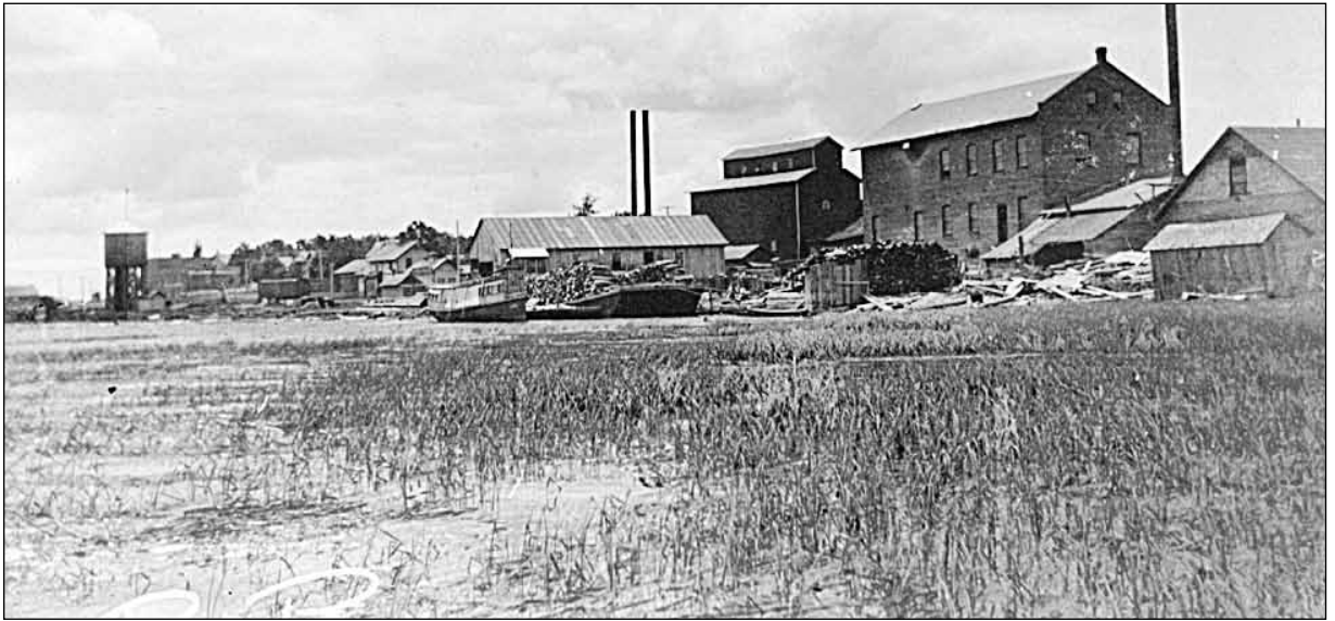
The lakefront of Port Perry, with its industrial buildings, were all being effected by the low water, as seen in this picture.
