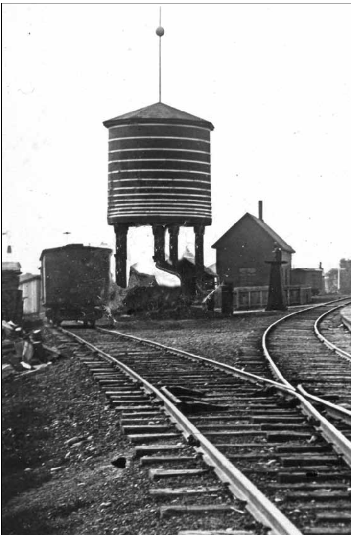
A new water tank was erected at the Port Perry railway station.
