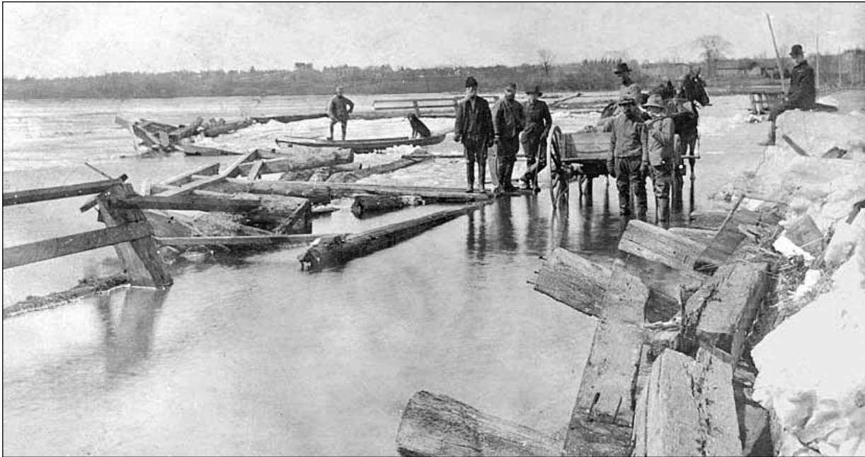
Ice damage was a common problem every spring for the Scugog Bridge, but especially bad in March 1908.
