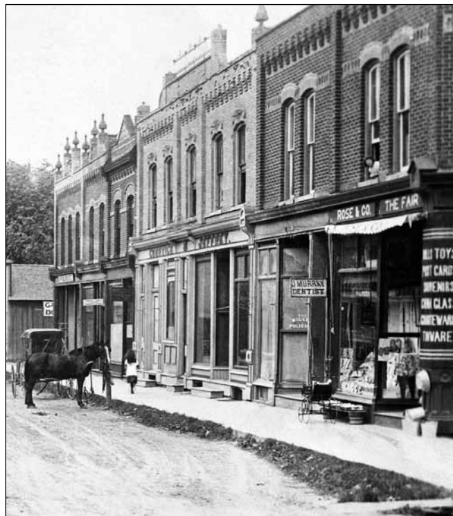
Buildings along this section of the western part of town, on Queen Street, were: Rose & Co. "The Fair"; J. Murray, Dentist (upper floor); Courtice and Jeffrey Harness Shop, and Monet's Grocery store
