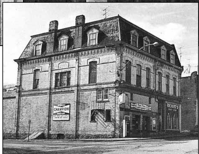
ST. CHARLES BUILDING 1976
