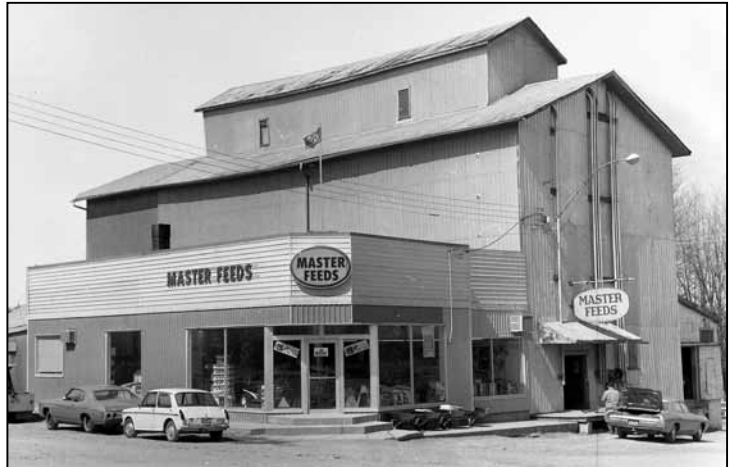
MASTER FEEDS ELEVATOR - circa 1971
