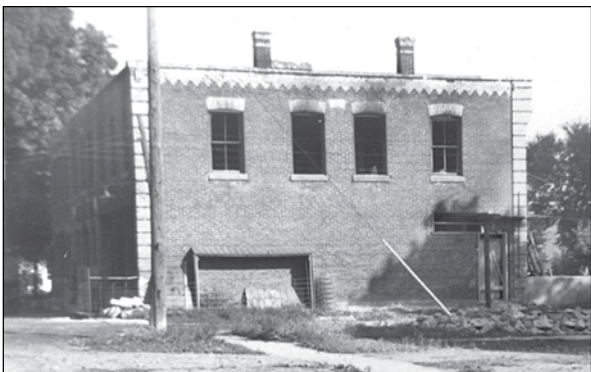
A fire in 1951 gutted the upper floor and damaged the building.
