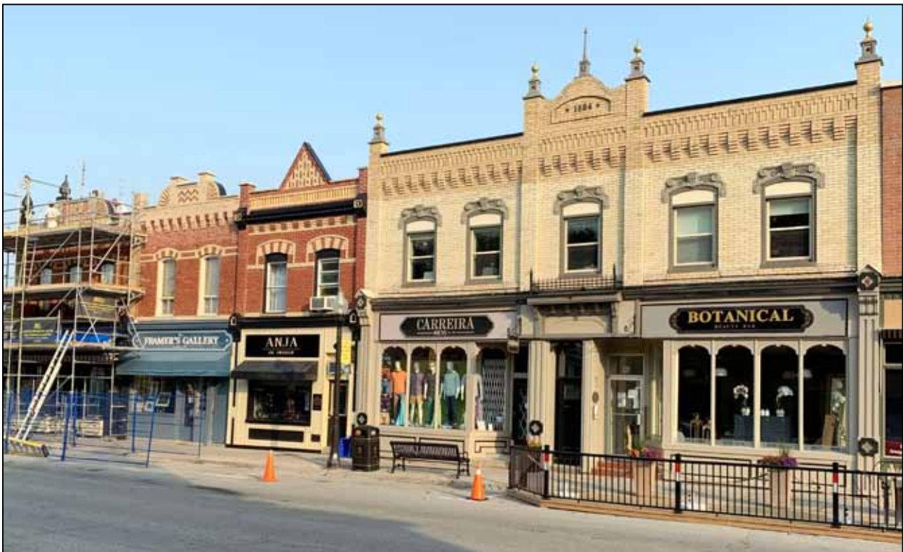
The west end block of Queen St., in 2021 with parapets being replaced on the three buildings to the left, and the Dan Stone family block of yellow brick with the redesigned parapet which was restored in 2010
