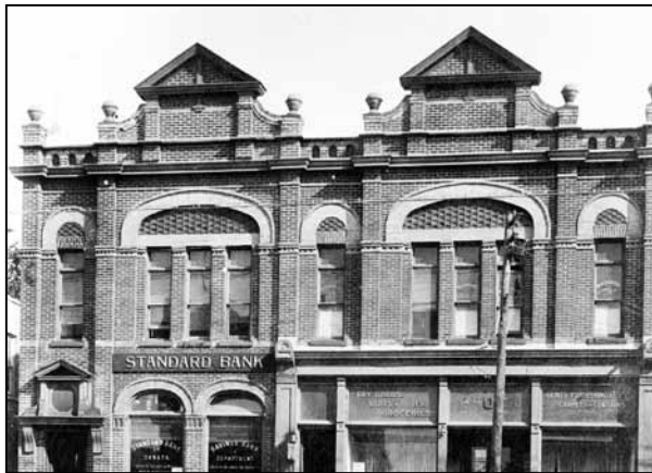
Original parapets on Brock's & Standard Bank, circa 1900.
