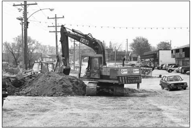
Twinning the sewer lines along Water St. in May 1989.
