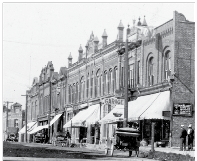
Buildings along Queen St., with their attractive parapets, circa 1900.
