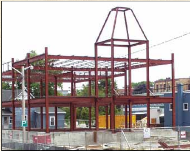
Steel frame of the new Scugog Township building in August 2003.
