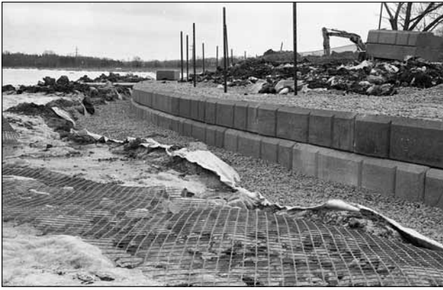
Developers construct a seawall around the project in March 1988.
