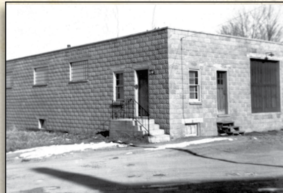
Norman Tease new Lakeshore Knitting Mill building on opened on Perry Street, about 1951.
