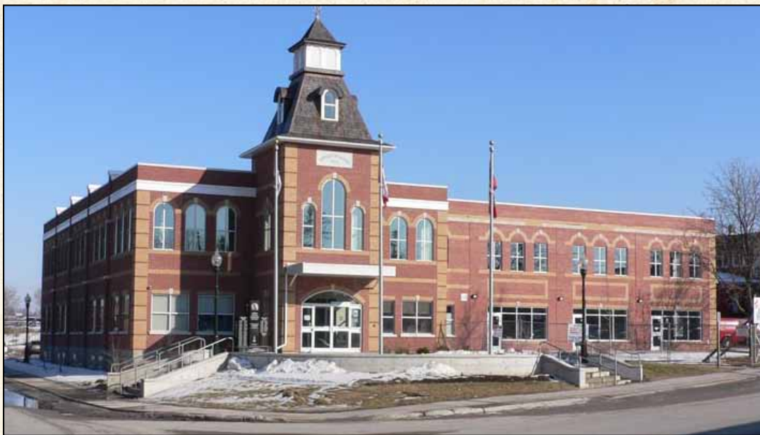
Scugog Township's new municipal office complex was opened for business in January 2004.
