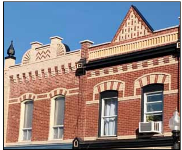
Framer's Gallery, left and Anja of Sweden had their parapets restore and rebuilt under the grant program in the summer of 2021.
