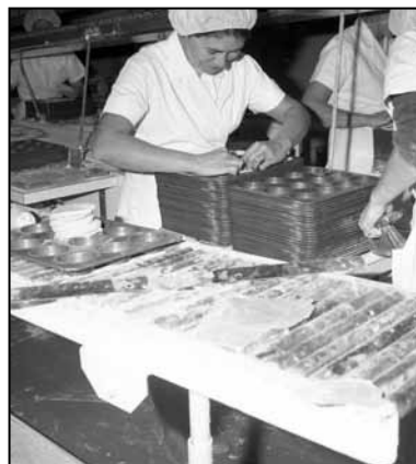
Production line at the new Flamingo Pastries plant on Simcoe St. (no Old Simcoe St.), in October 1968. Allan Rahm is seen with a fresh batch of dough, which will produce 500 dozen tarts. The stuffing of tart tins was still done manually, but the filling of the tart shells was done by machine.
