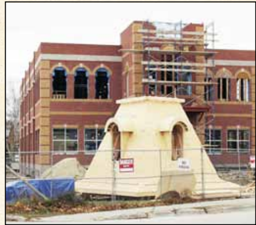
Top of tower waiting for cedar shingles.
