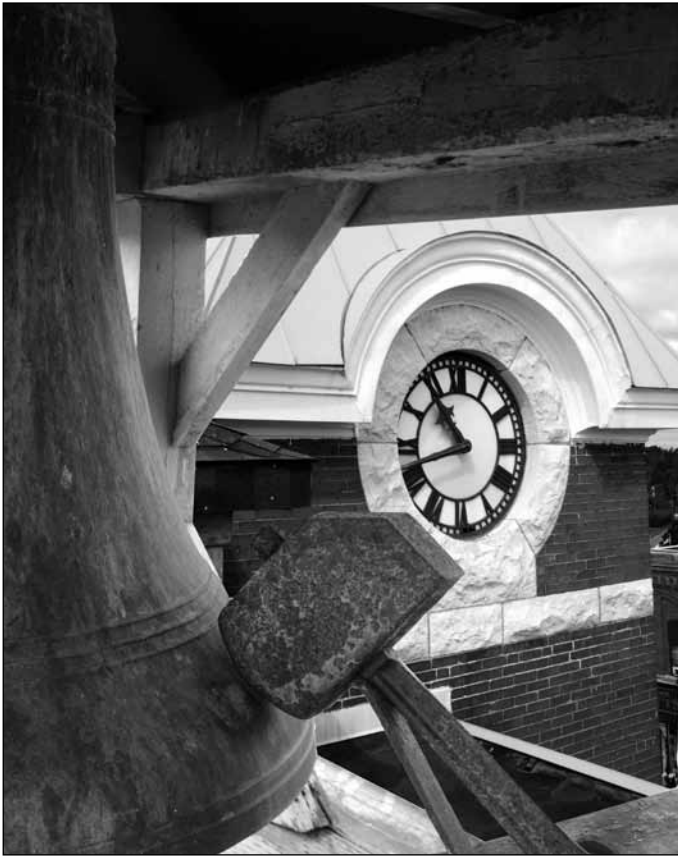
The bell and striker can be seen in this picture taken in 2013, with the clock and tower in the background.
