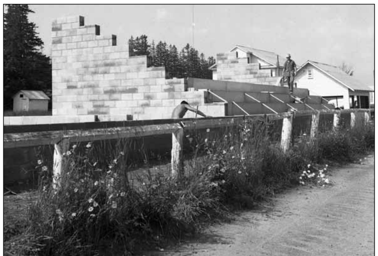
Construction got underway on a new grandstand in the summer of 1967.
