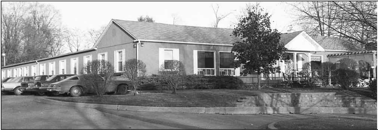
Port Perry Villa as it looked in November 1998.
