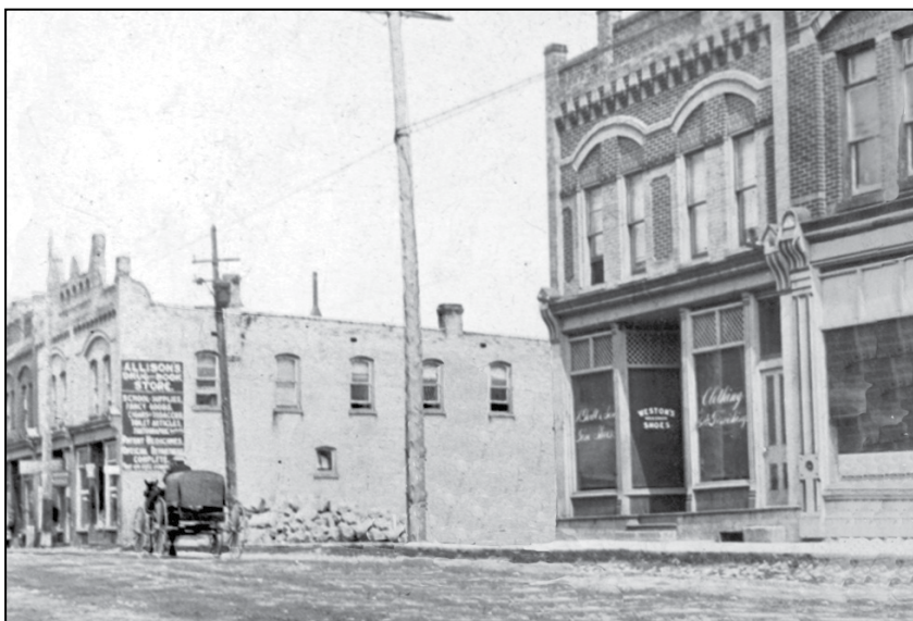
The Sinclair property, was chosen for the new post office. Picture shows the property after the fence was removed, and construction getting underway in the fall of 1911.
