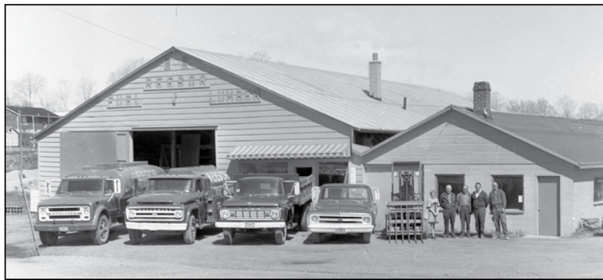
Reesor Fuel and Lumber, on Scugog St. (Hwy. 7A), at Water St., 1971.
