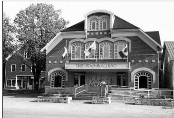
Port Perry Star building, 1991.
