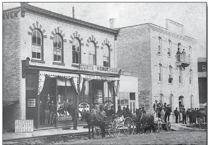
Curts & Henderson, Marshall's and Sebert House.
