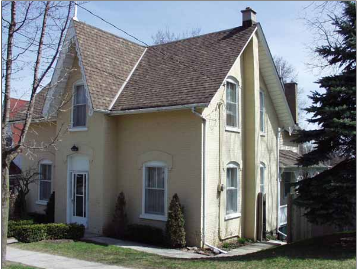
This substantial brick home, located on the south side of Queen St. was built about 1878.
