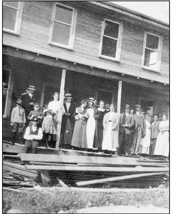
The new Delmont Cottage during construction by Albert C. Stinzel about 1914, with an unidentified group of people on the porch.
