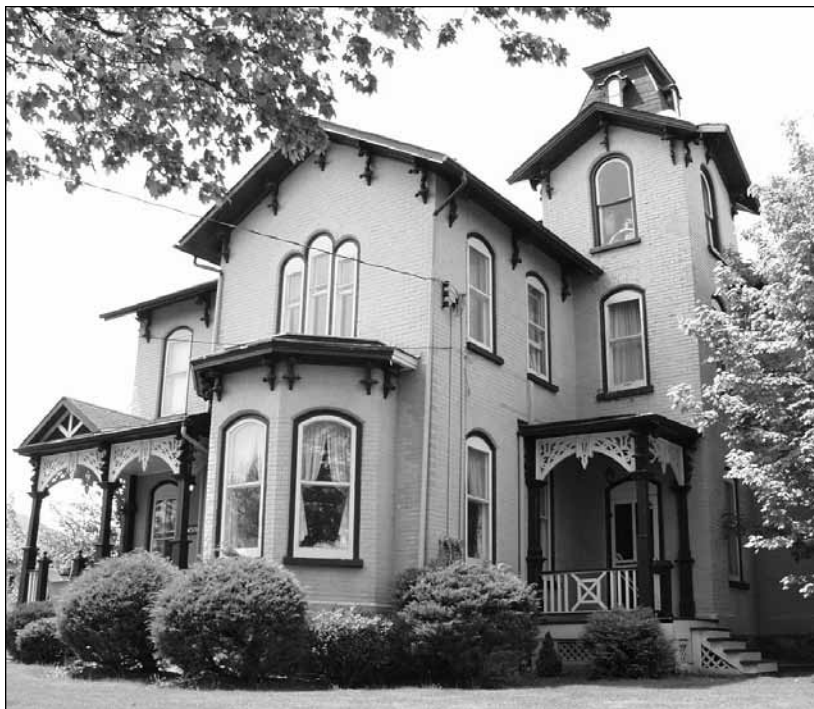
This photograph, taken in 2002, and the one below, taken about 1900, show the house from the same angle, although it is partially hidden by trees.
