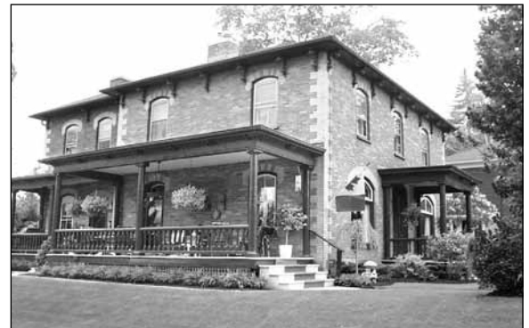
A view of the north-east corner of the Jackson house.
