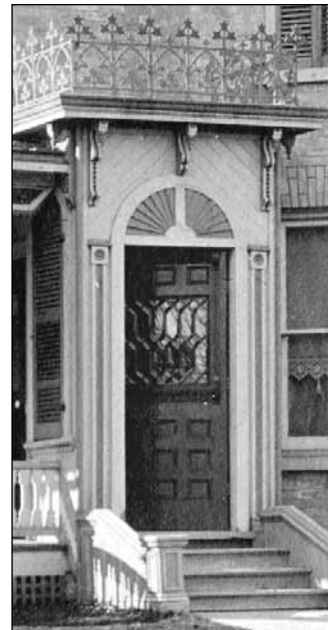
Ornate front porch was removed.
