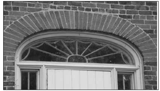
Elliptical fanlight window above front doorway as it looks from the exterior of the house.
