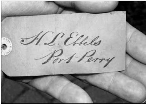
Tag found in winter of 2001 by Steve and Alice Carnegie while renovating the pantry on the main floor. The tag was in the wall still attached to an original 2x4 used in the construction of the home.
