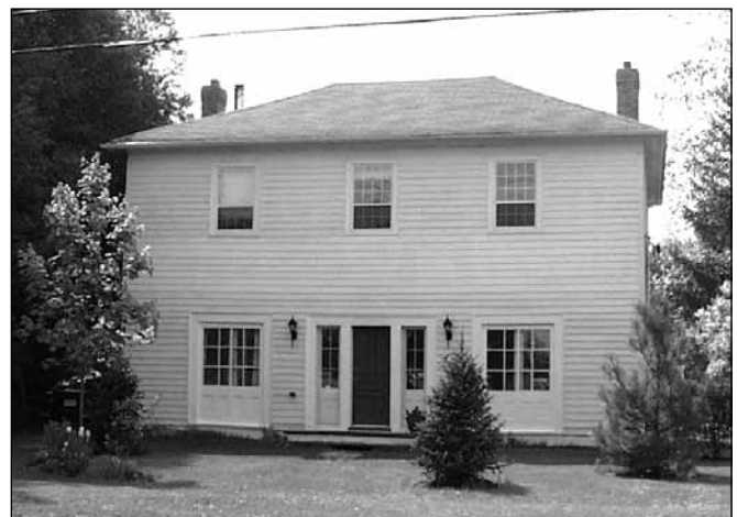
Rowan Tree Hall has changed little over the past 150 years, although the porch has been removed in this 2001 photograph.
