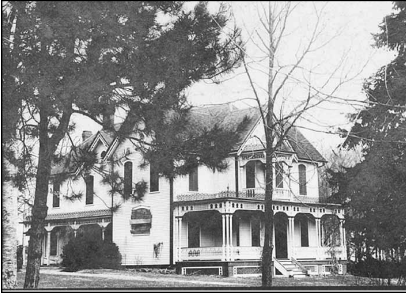
This large frame house was built by Johnathan Blong during the late 1800s, at his Beechcroft property, and later became the Kent family home.
