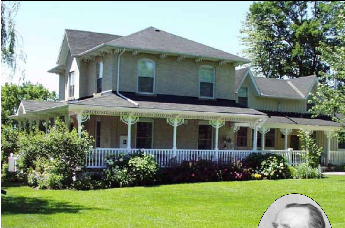
South west side of the Bateman home while under restoration in 2004.
