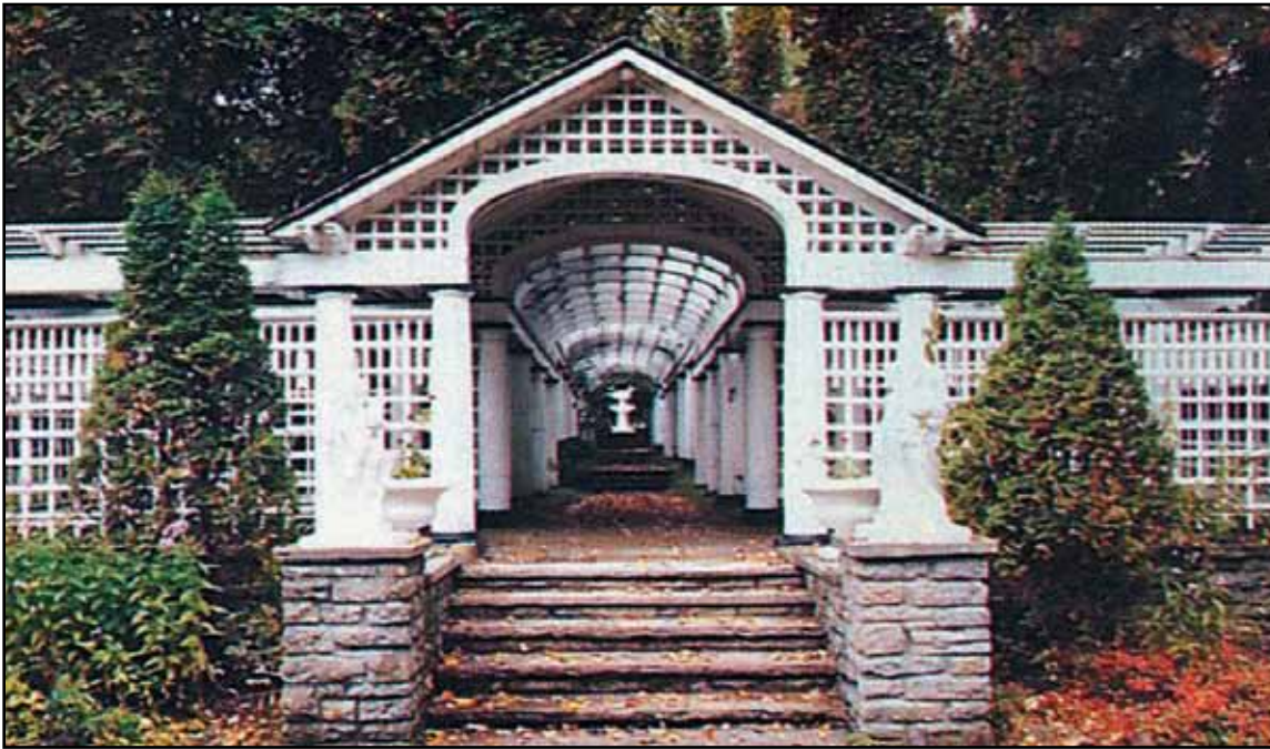
Entrance of the magnificent white lattice covered pergola which leads to a large fountain near the main residence.
