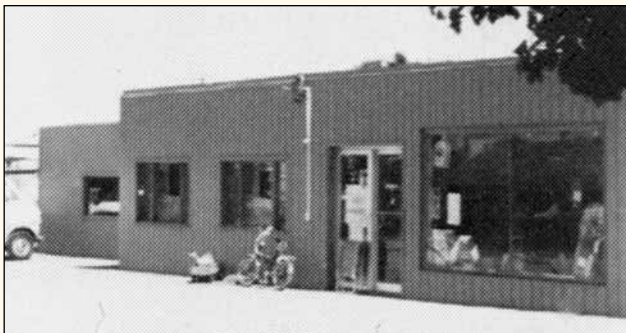
Construction on Frank Hoskin's store began in October 1950.
