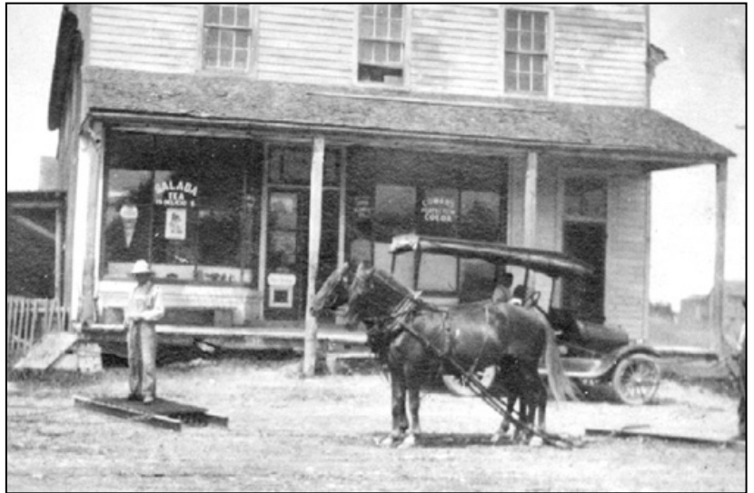
The former S.H. Christian and Deforest Hagerman store as it looked during circa 1918.
