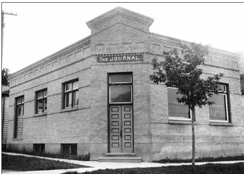
The new Uxbridge Journal Printing Office was constructed at the corner of Brock and Church St., just east of its old stand, which can partially be seen at the far right.
