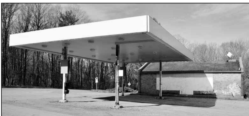
The former Ridgeview Gas Bar and Snack Bar building now vacated and in ruin. Exactly when it closed has yet to be determined, but it was abandoned for many years before this photograph was taken in May 2024.
