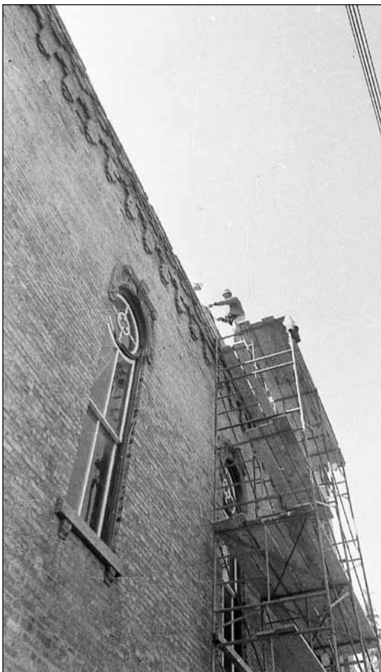
Construction inside the Town Hall had been steady all winter and now that spring has arrived repairs to the exterior got underway. Martens Masonry & Construction Ltd., commenced the work of repairing and replacing the brick parapet on top of the building. April 14, 1975,
