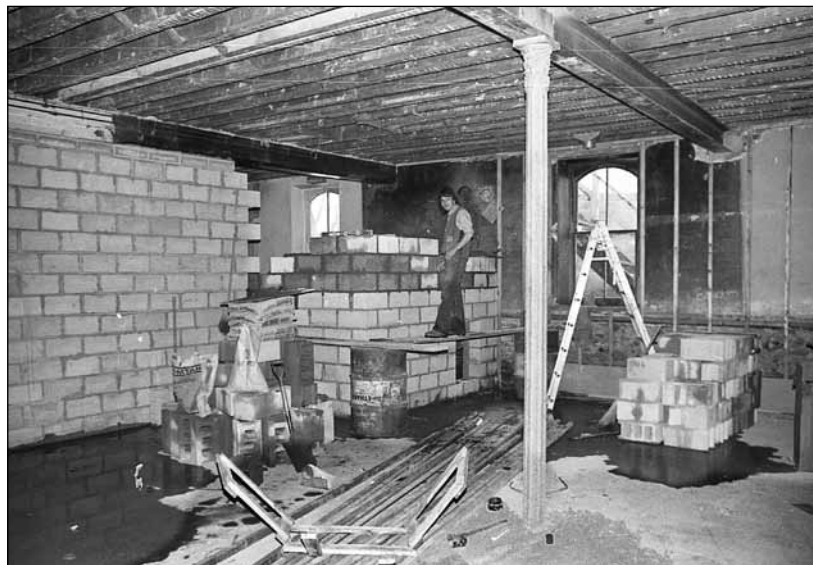
Work got underway restoring the basement of the Town Hall in February 1975, including a new floor, cement block walls and steel support beams under the floor.
