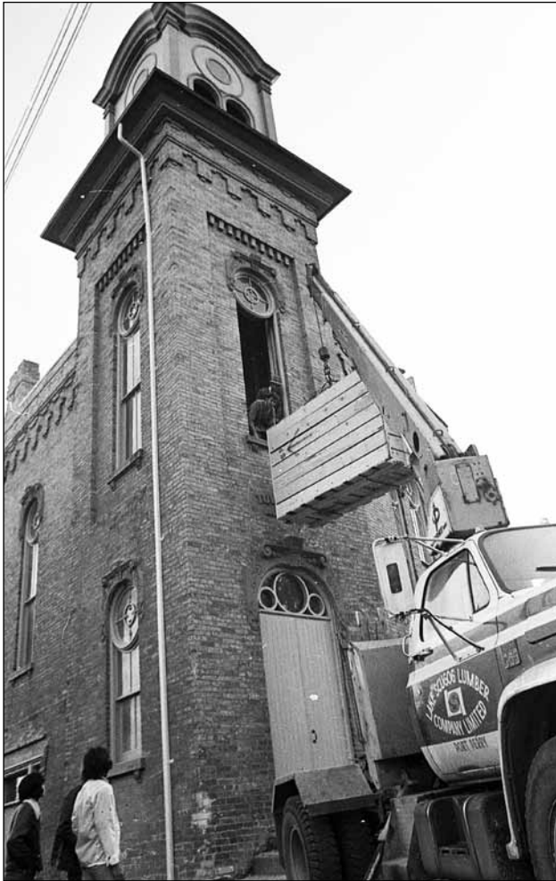
Almost 1,000 pounds of wiring, instruments, dials and electrical gadgetry was lifted through the tower window of Town Hall 1873 on November 20, 1975. The lighting panel has been long-awaited, and after installed in the upstairs of the hall will be used to light up stage productions. Cost of the equipment was about $7,000. Lake Scugog Lumber provided the truck to lift the equipment into place.
