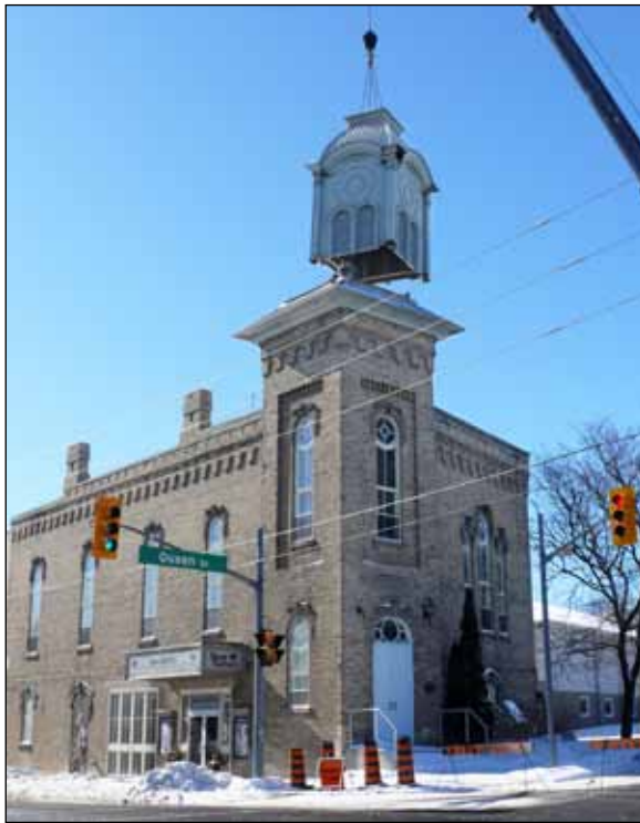
Up, up and away! Town Hall 1873 bell tower was detached and lowered to the ground for repairs on February 28, 2019.
