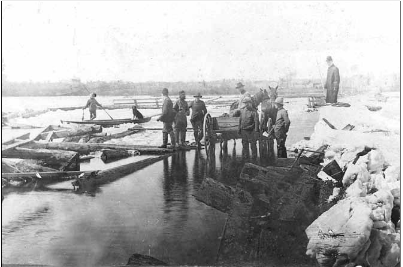
The Scugog Bridge following extensive damage in the spring of 1908.
