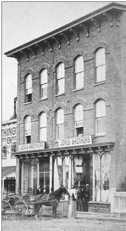
Jones Brothers open their new brick building located on Queen St., Port Perry, in October 1872.
