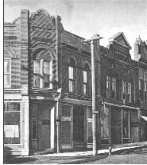
The Currie block, on the corner of Queen and Perry Streets, after being rebuilt in 1884. The new building was damaged on May 24, 1887, when a fire destroyed stores of Brown and Currie. Note difference in brickwork on upper structure and details in the bricks around windows.
