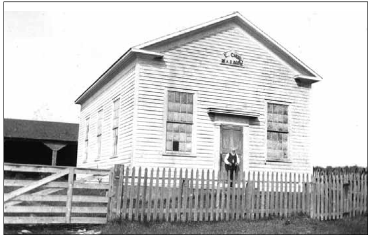
Bethel Methodist Episcopal Church, was built in 1860, on the north east corner of Simcoe St. and Clements Rd. (Conc. 11).
