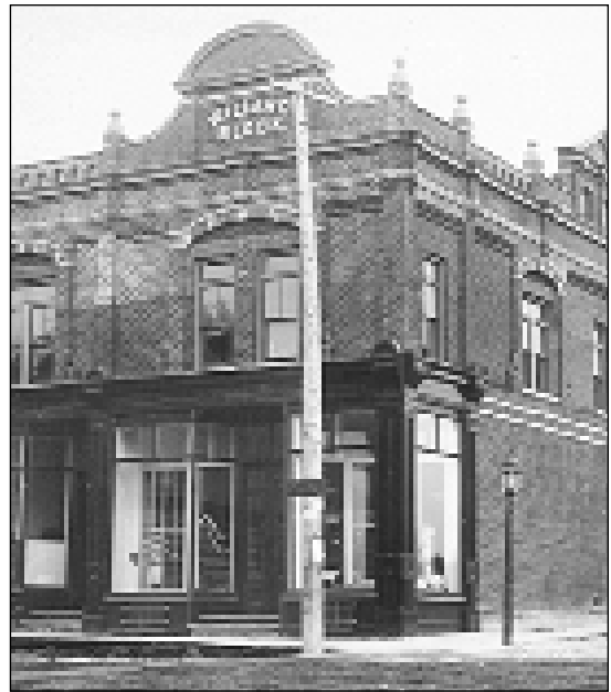
Willard's store in the Willard Block gutted by fire.
