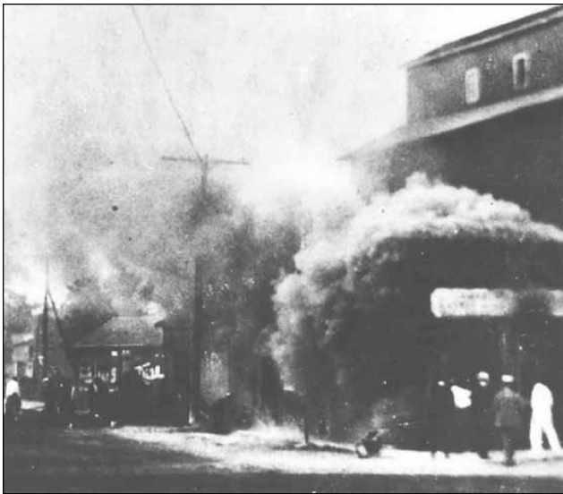
Fire destroyed the offices of Hogg & Lytle in August 1920, but the flames were prevented from spreading to the elevator.
