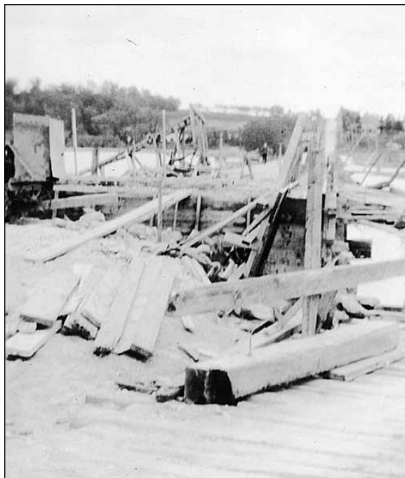
A section of the Scugog Bridge , or Causeway while under construction during the summer of 1928.
