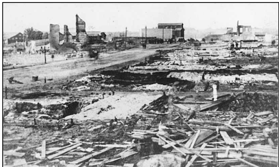
View of the damage caused by the July 4, 1884, a few days after the disaster.
