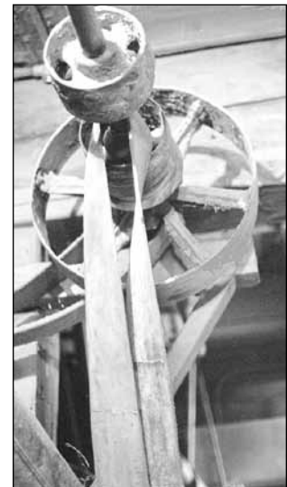
Pulleys and belts hang unused in the mill in 1979.
