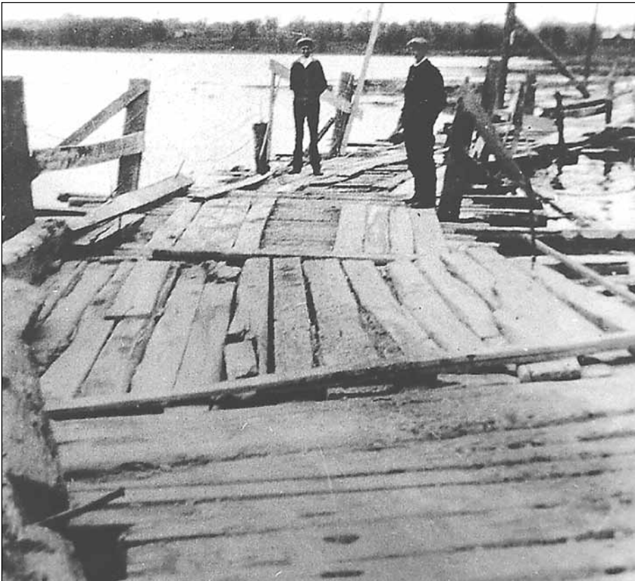
The original floating Scugog Bridge, built in 1856, as it looked prior to it becoming a permanent road.
