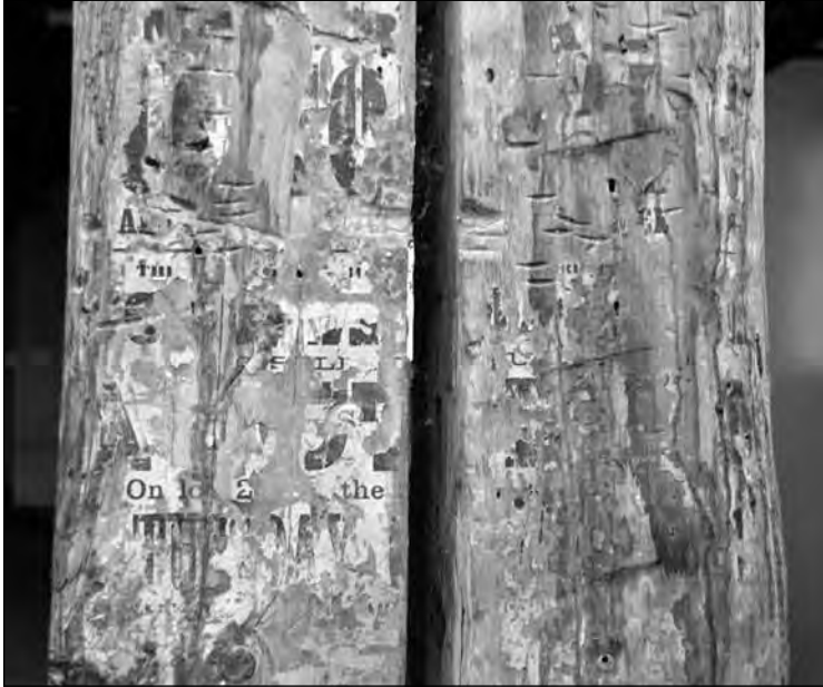
Large hand hewn posts were often assembled into groups of two or four to create one massive support column.
