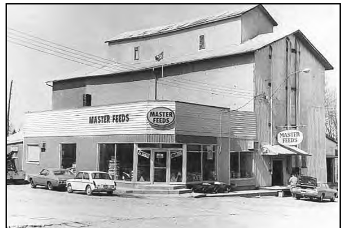
Master Feed's grain elevator July 1971
