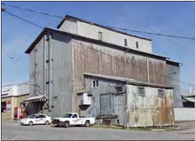
Elevator looking northwest from Palmer Park.
