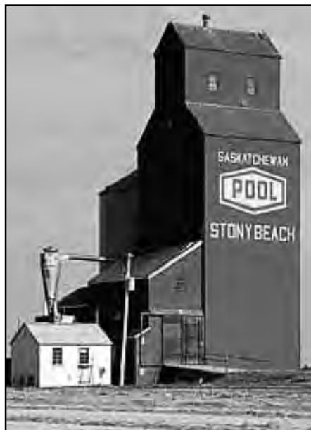
The Western Grain Elevator was more square in shape.
