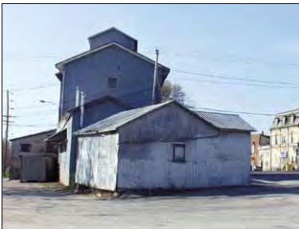
The elevator looking south from North St.
