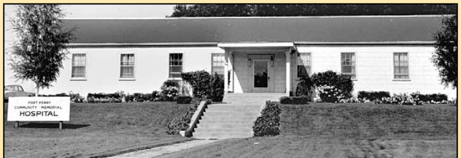
Community Memorial Hospital, Port Perry opened in 1953
