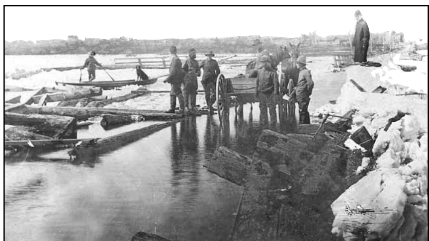
Ice damage to the Scugog Bridge during the early 1900s.
