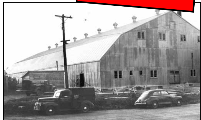
Construction nears completion on the new Port Perry Memorial Arena and Recreation Centre in the fall of 1950.
