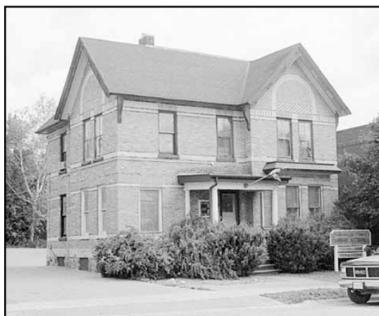
This turn of the century home located on Queen St. is occupied by the offices of Powell, Shepherd Accounting.
