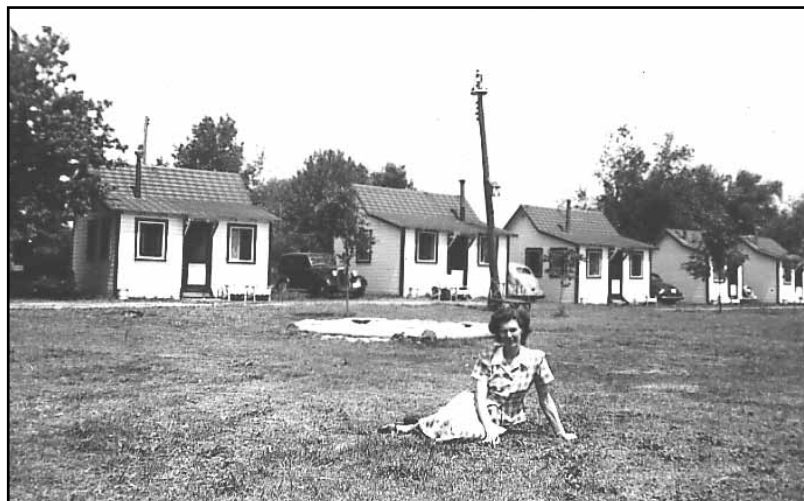
BIRDSEYE CENTRE CABINS
