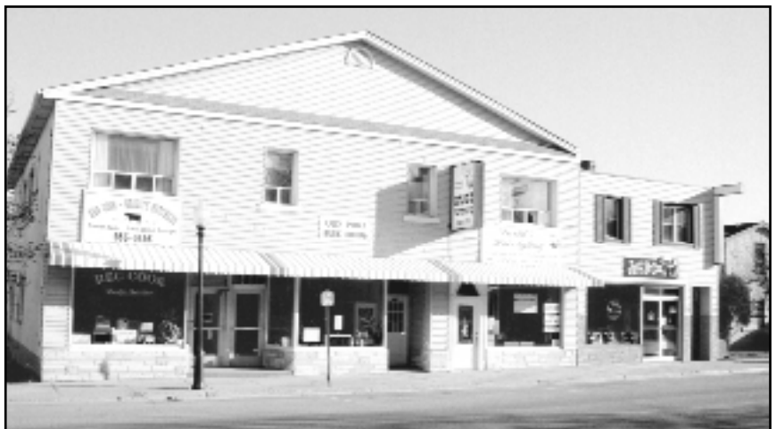
This block of stores at the west end of Queen St. was originally built by James Carnegie. It is currently owned by David Menzies who operates David's Hairstyling in the building.
