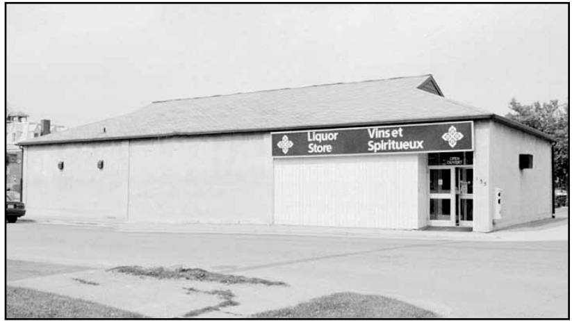
The LCBO Liquor Store as it looks in 1998, formerly the Ontario Carriage Works.
