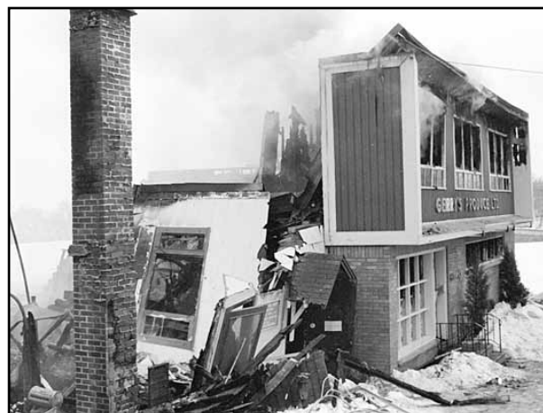
FIRE AT GERRY'S PRODUCE Fire ravaged the warehouses and office of Gerry's Produce, Port Perry causing an estimated $1.5 million damage and loss in March 1982.
