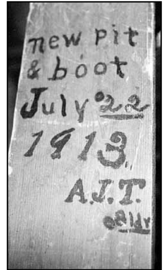
Graffiti on one of the massive wooden beams tells of the mills history.
