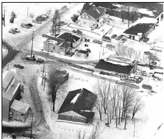
Aerial view of the old Lake Scugog Lumber site. The Latcham Centre is seen at bottom of photo and the old mill at left. The Griffen house, at top, was taken down and is now the location of the Scugog Memorial Library.
