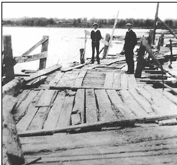
A floating bridge was built to link Port Perry with Scugog Island in 1854.
