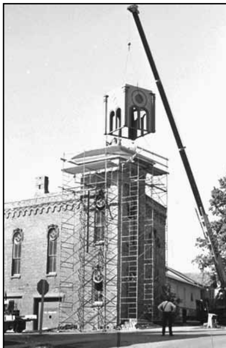
Town Hall 1873 with tower being replaced.
