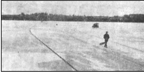
In March, Bell Telephone crews cut a large slit in Lake Scugog's ice surface to lay new telephone cable to Scugog Island.
