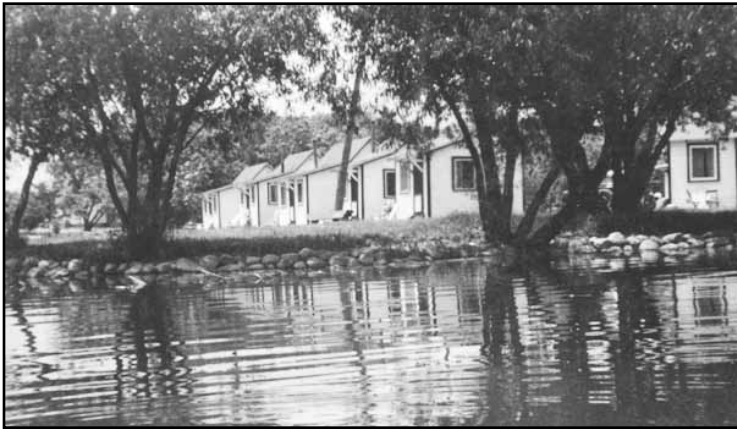
Above: Photo of some of the nine Birdseye Centre Park cabins as they looked from the lake during the 1950s.
