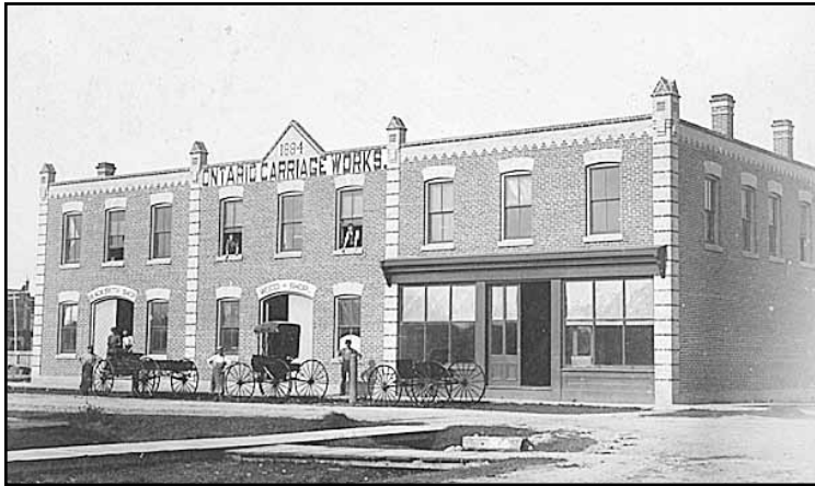
ONTARIO CARRIAGE WORKS
