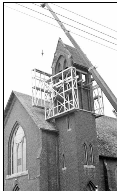
UNITED CHURCH REPAIRS
