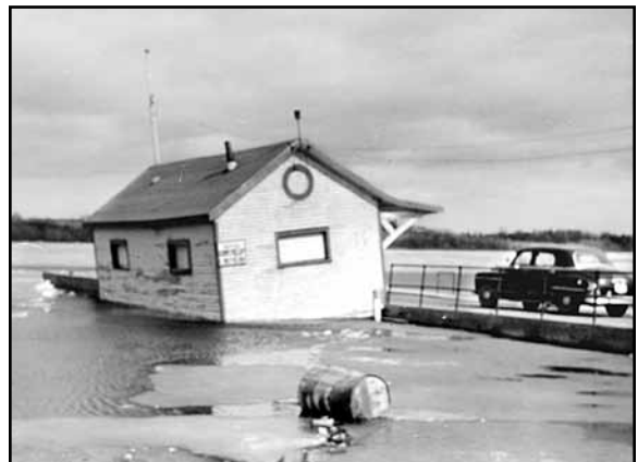
Pilings under the dockhouse, which was built in 1915, were damaged when the ice went out in spring of 1958.
