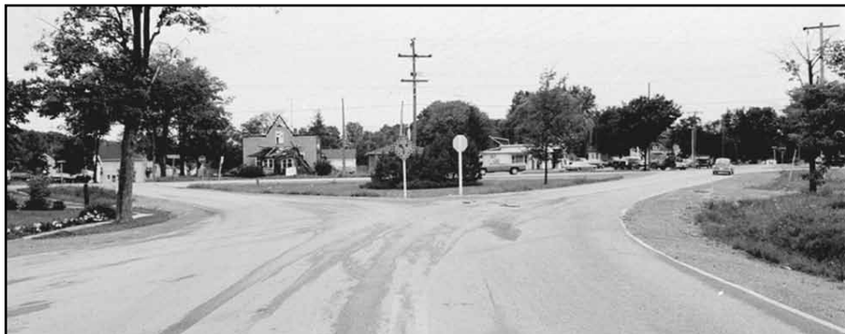
Work began in September on the intersection of the Oshawa Rd. and Scugog St. (7A). The island in the 'Y' of the road was removed, the road widened and signal lights installed.
