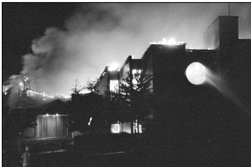
Fire rips through the roof of the Immaculate Conception Church before dawn on Sunday, May 31, 1998.
