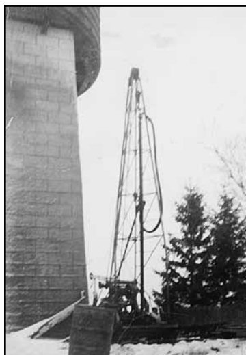
NEW WATER TOWER
