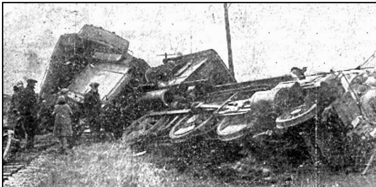
TRAIN WRECK Heavy rains washes out tracks near Manchester, derailing train.
