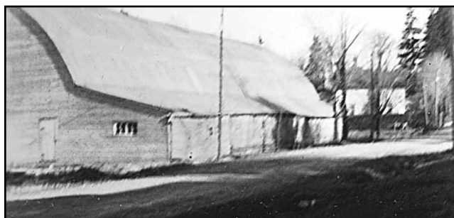
The Port Perry Rink on Lilla St. (built in 1922) as it looked about 1940.
