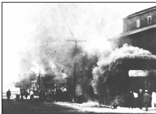
FIRE AT HOGG & LYTLE Fire guts offices and front end of elevator building in Aug. 1919.
