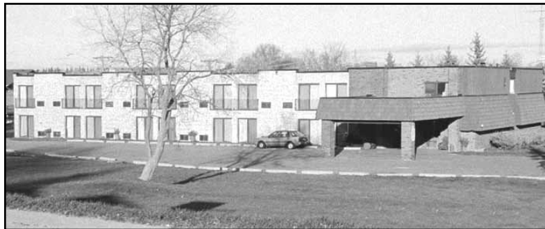
RAILROAD HOUSE MOTOR HOTEL Located on Scugog St., Port Perry.
