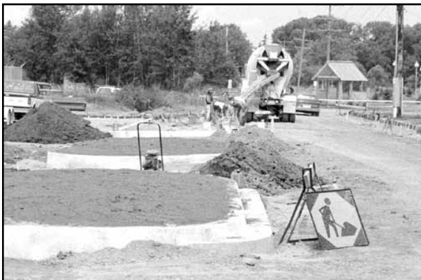
Work begins on enlarging and repairing township boat launch.
