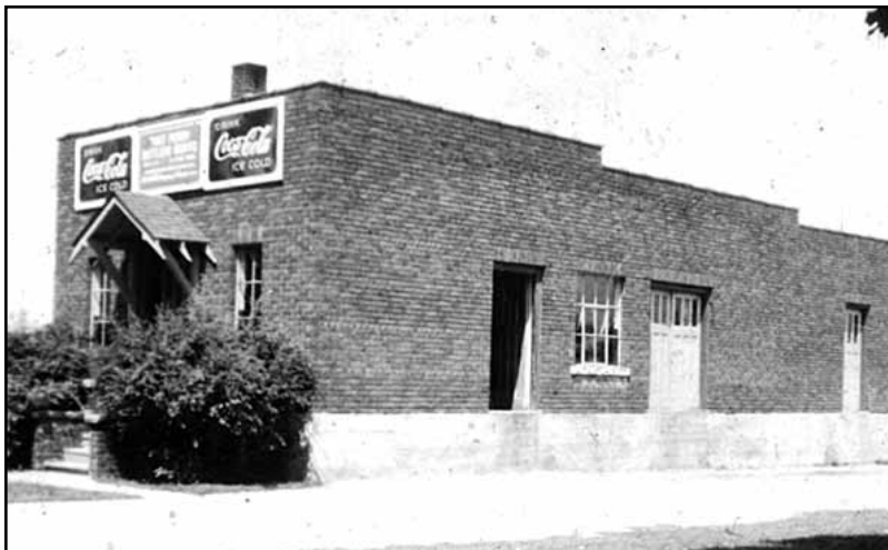
PORT PERRY BOTTLING WORKS
