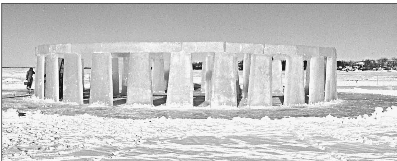
Bill Lishman, with a group of volunteers, constructed "Icehenge" just off the wharf at the end of Queen St. Unfortunately it collapsed due to the weight of the structure.
