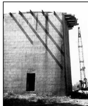
Port Perry's old water tower was taken down in August 1962.
