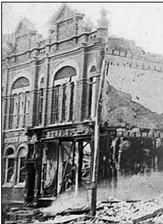
This enlargement of the upper photo shows the badly damaged and charred exteriors of A. Ross & Sons store and the Western Bank. This is the building occupied by Brock's store today.
