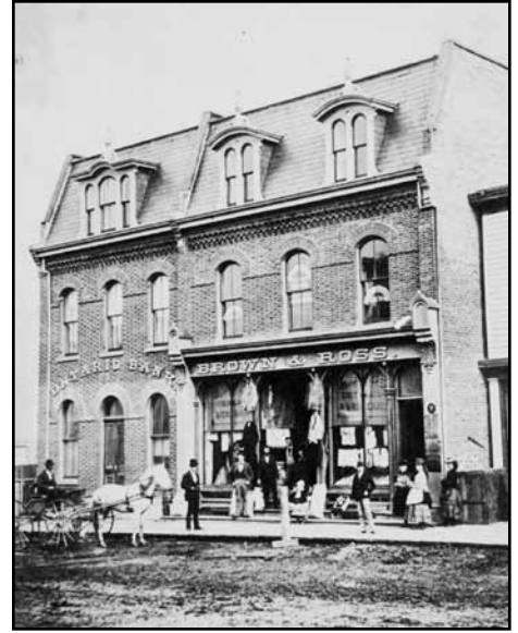
The attractive Ontario Bank and Brown & Ross building as they looked before fire destroyed them in 1884.
