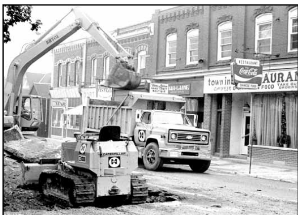
QUEEN STREET CONSTRUCTION
