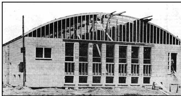
Construction on new Port Perry Curling Rink well underway.
