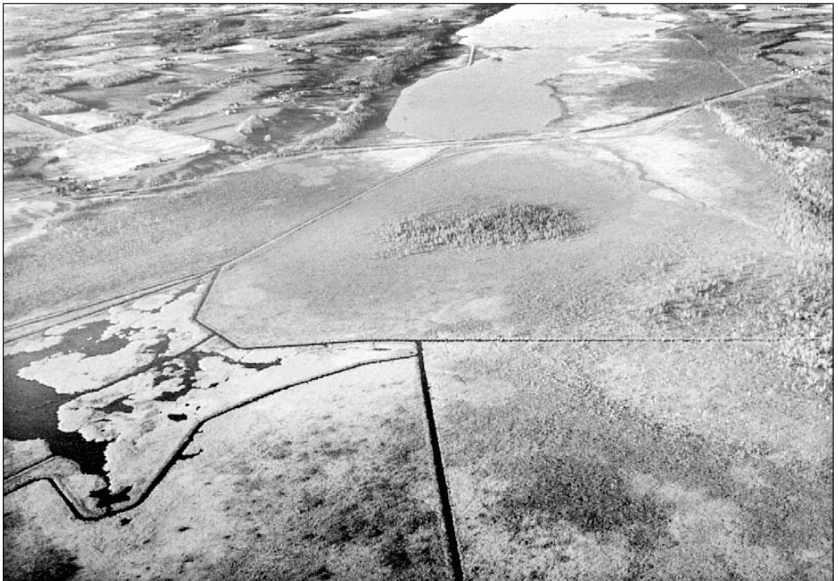
View of the marshlands and canals, looking north across the Cartwright Causeway. Land on both sides of the causeway belong to the Osler family and some of the 20 miles of canals can be seen cutting through the property.
