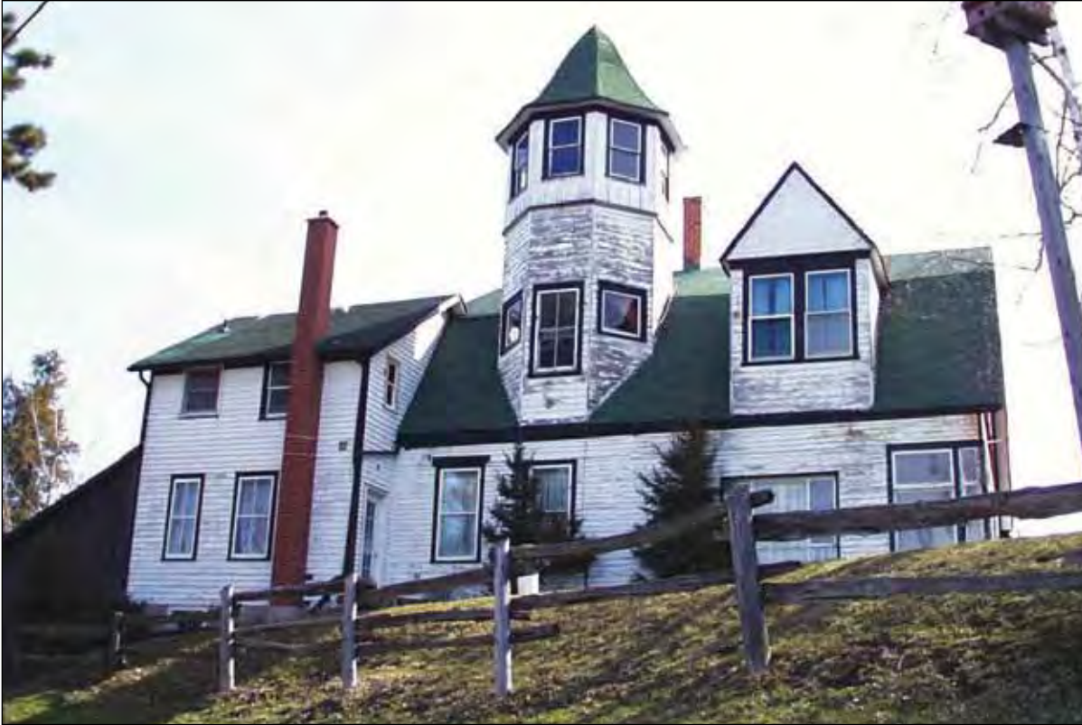
The Osler's clubhouse, right with tower, and the caretaker/gamekeeper residence, at the left, about 2000.
