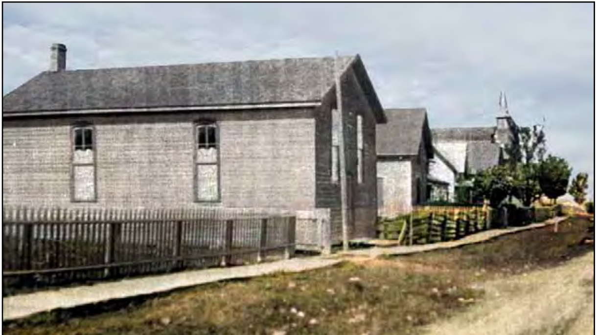
These buildings located on the north side of Cragg Road, Greenbank, show the Temperance Hall and a few other building before the steeple of the Presbyterian Church comes into view.
