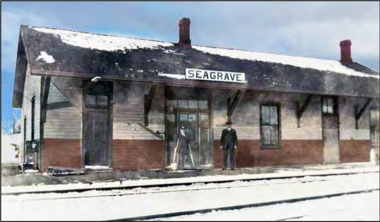
The Seagrave railway station was built about 1873, when the line was extended from Port Perry to Lindsay.
