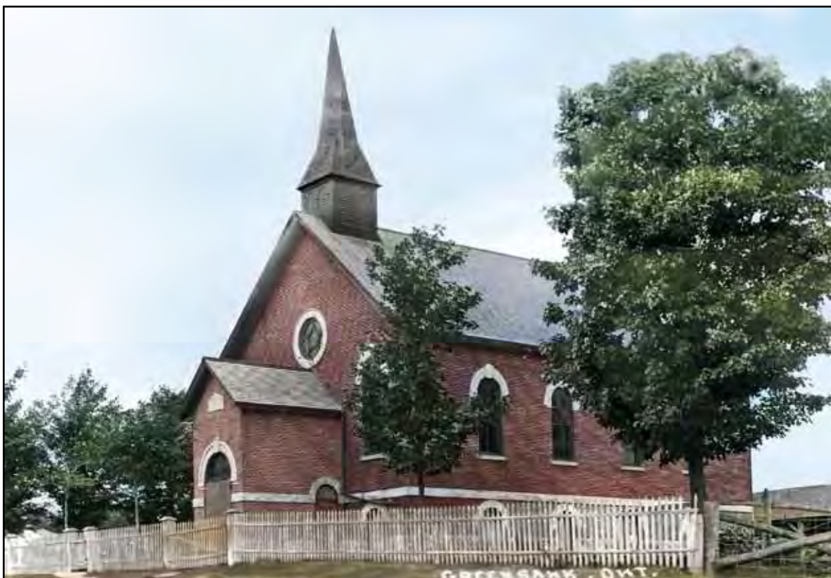
The Greenbank Presbyterians constructed this Presbyterian Church just east of the intersection, on Cragg Road. The congregation held a Dedication Day, and the church was officially opened Sunday, November 10, 1878.
