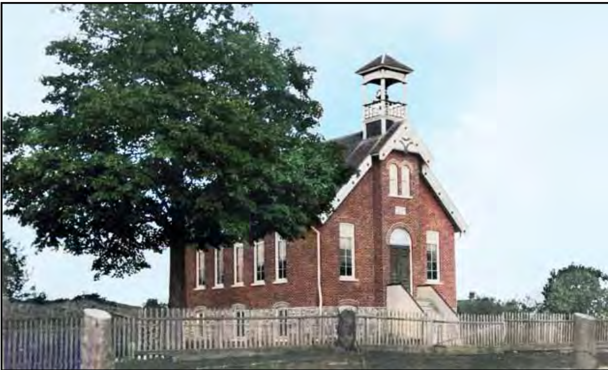
This classic red-brick building is the Blackstock Public School, which was opened in 1896.
