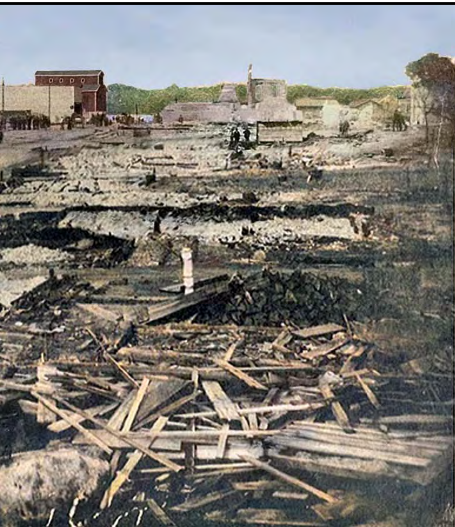
Only the large Grain Elevator near the lakefront, and the partially rebuilt Curts and Henderson block escaped total destruction from the devastating fire.
