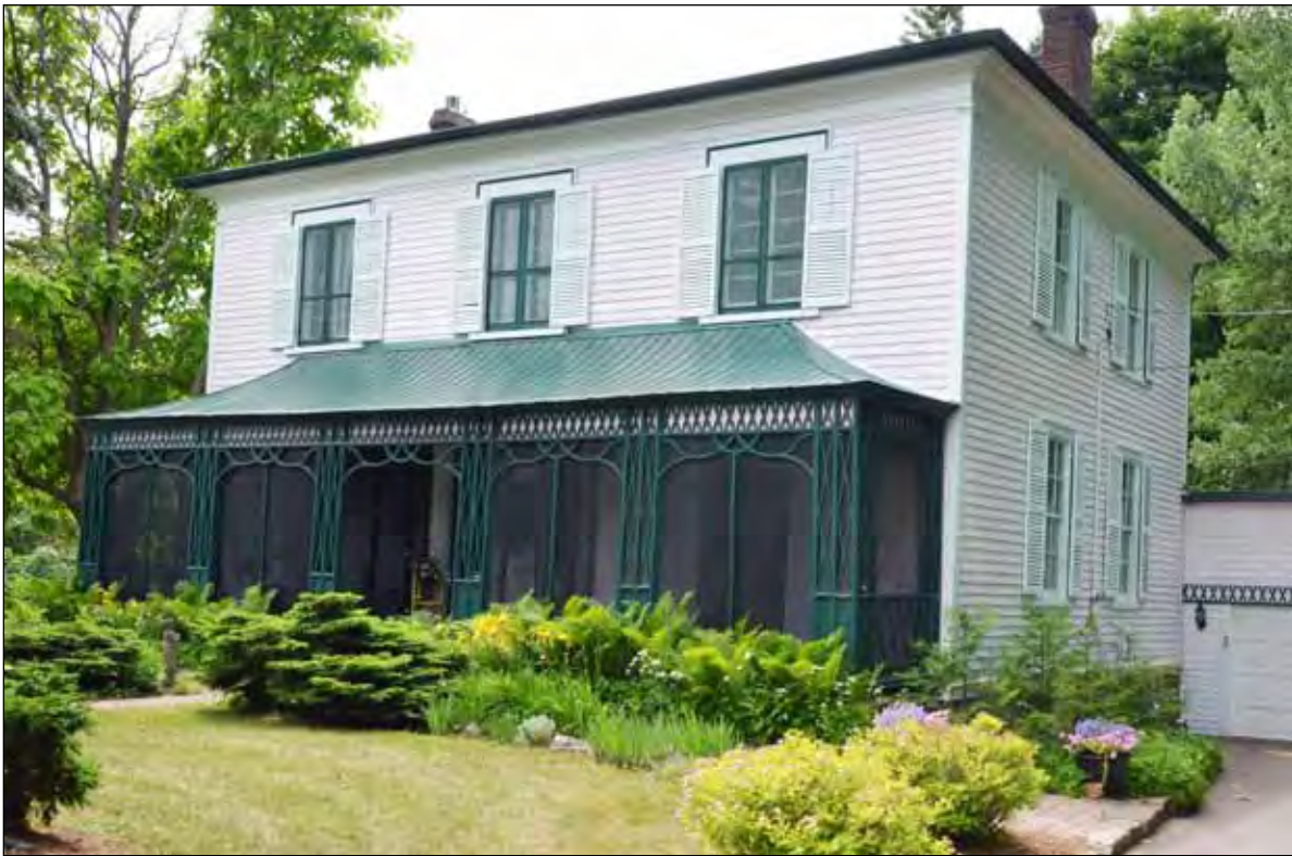
This substantial two-storey home was built by Aaron Ross during the 1850s.
