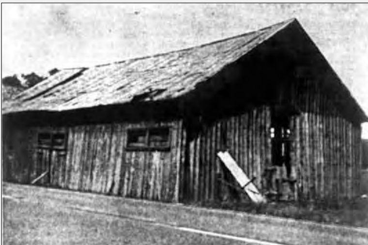
This "Drill Shed" from near Ottawa, would be similar to the one built in Prince Albert.
