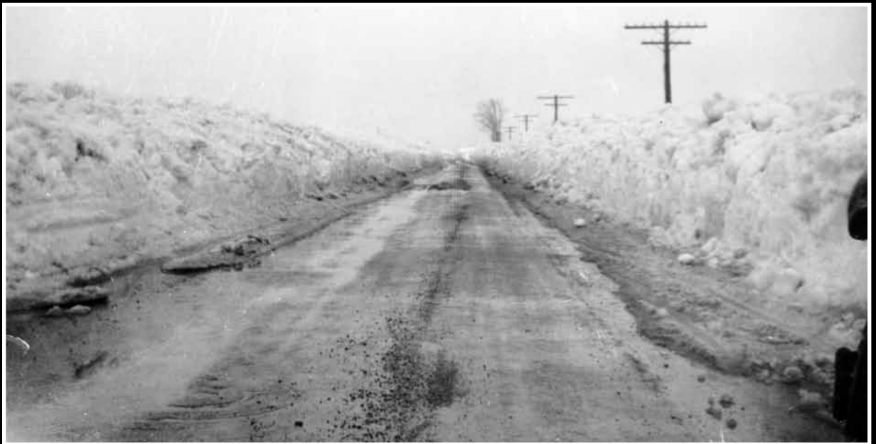
Highway 7A, looking west towards Manchester following a storm in January 1941.
