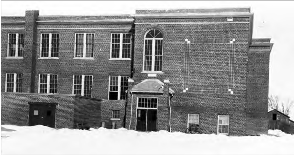
West side (rear) of the Port Perry High School about 1944.
