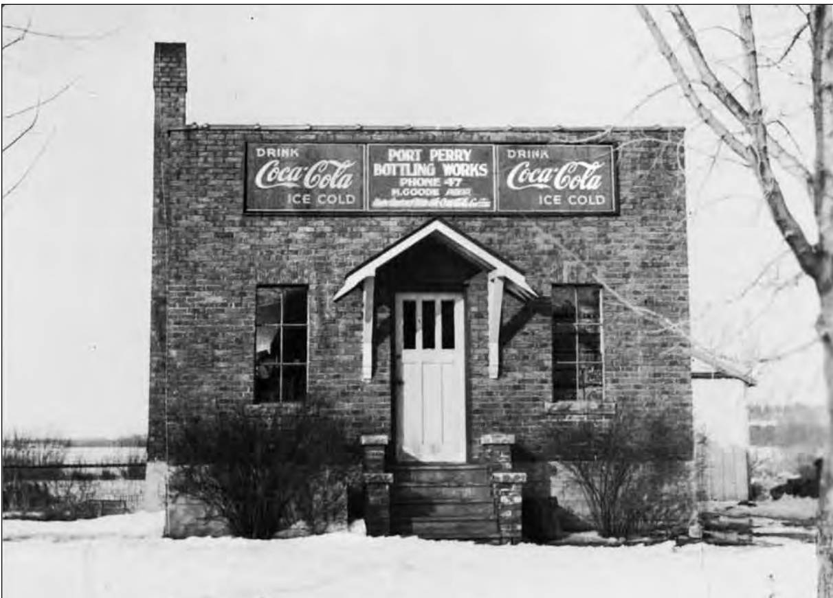
Port Perry Bottling Works, bottlers of Coca-Cola, announced in March 1940 that deposits on bottles of Coca Cola will be reduced from 3¢ per bottle to 2¢ per bottle. The bottling plant is located at the north end of Perry Street, in Port Perry.
