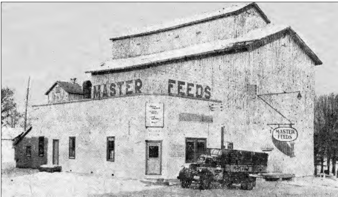
Toronto Elevators Ltd., purchased the Hogg & Lytle grain elevator in 1949 and operated under the name Master Feeds.
