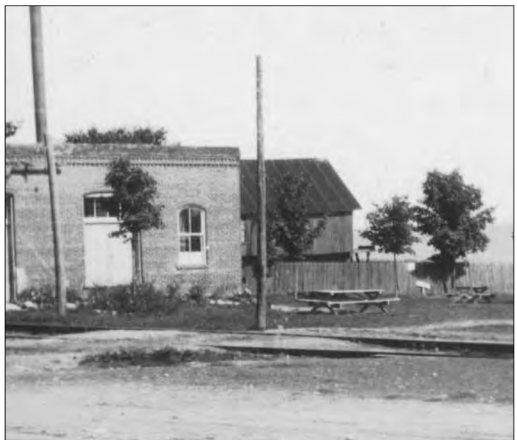
Port Perry's Hydro Sub-station at the east end of Queen St., at the lakefront.
