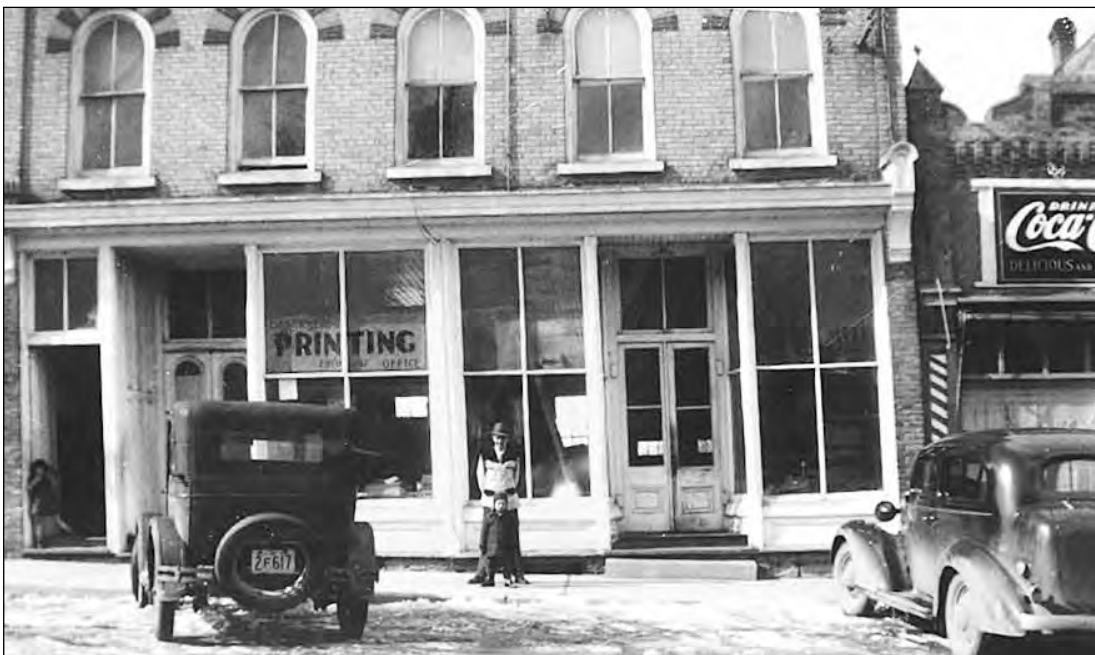
The Observer Printing Office operated from this building until it was purchased in the spring of 1945 by Ivan Haugen, who remodelled and opened the Delicataria "Del" Restaurant. Years later, during the 1950s, Mr. Haugen opened up the well-known "Haugen's Chicken Barbecue" resaurant on Hwy. #12, at Manchester.
