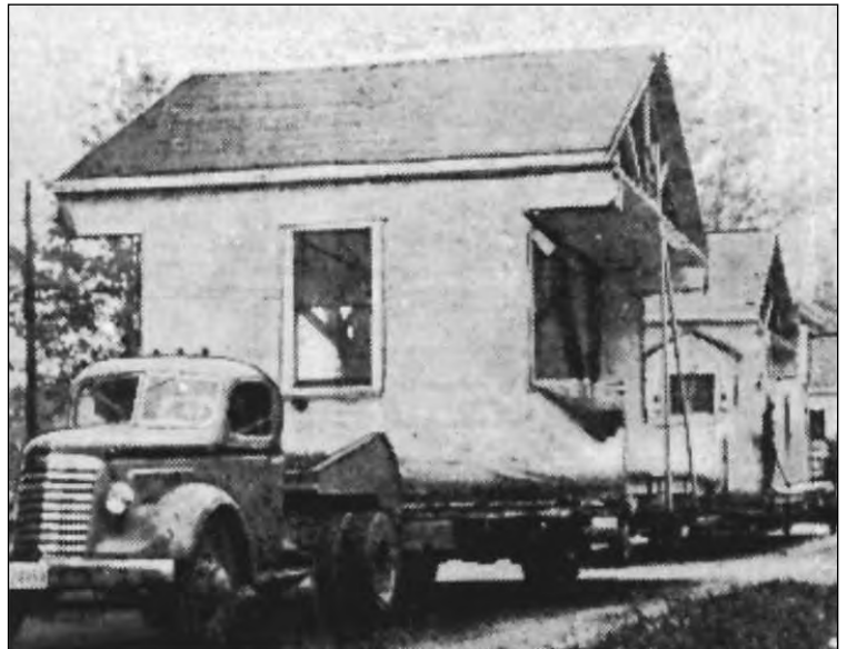
Sections of an old munitions factory from Ajax are seen here being moved by truck to Port Perry in October 1949 and were assembled on the new hospital site.
