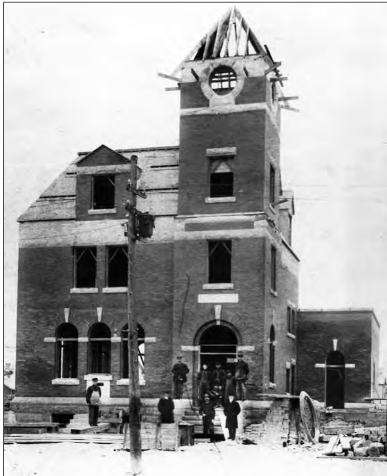
Construction of the Port Perry post office, in early 1912.
