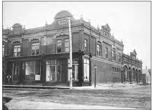
William Willard's store was located in the west unit of this beautiful block, the Willard Block, which he built after the fire of 1884.
