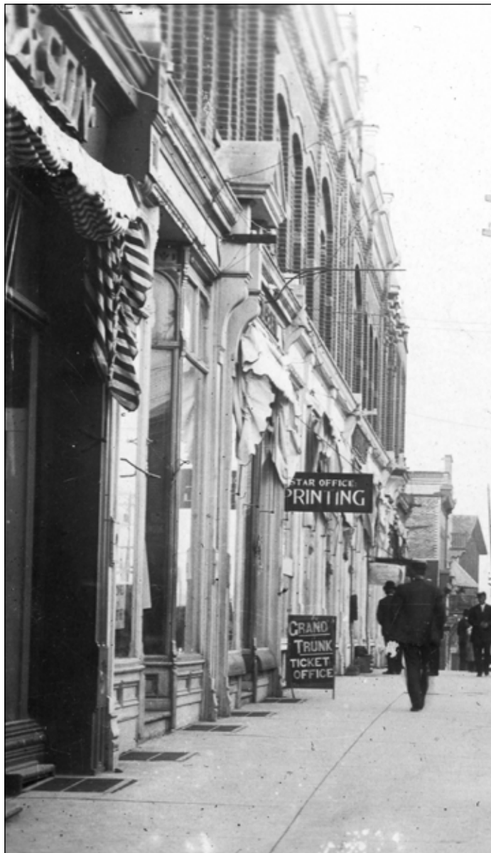
North side of Queen Street looking east with Jones & Sons store, left and the Star Office Printing halfway along the street.
