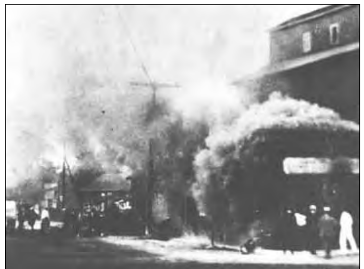
Fire broke out in the engine room of the James Lucas Grain Elevator, in March 1916, but damage was slight.
