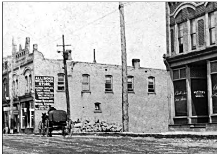
The merry-go-round was set up on the Sinclair lot, which was this empty lot on Queen St. The new post office was constructed on it a few years later.
