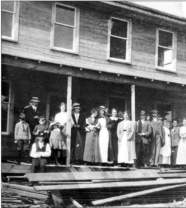
Gathering on the porch of the unfinished Delmont Cottage, 1912.
