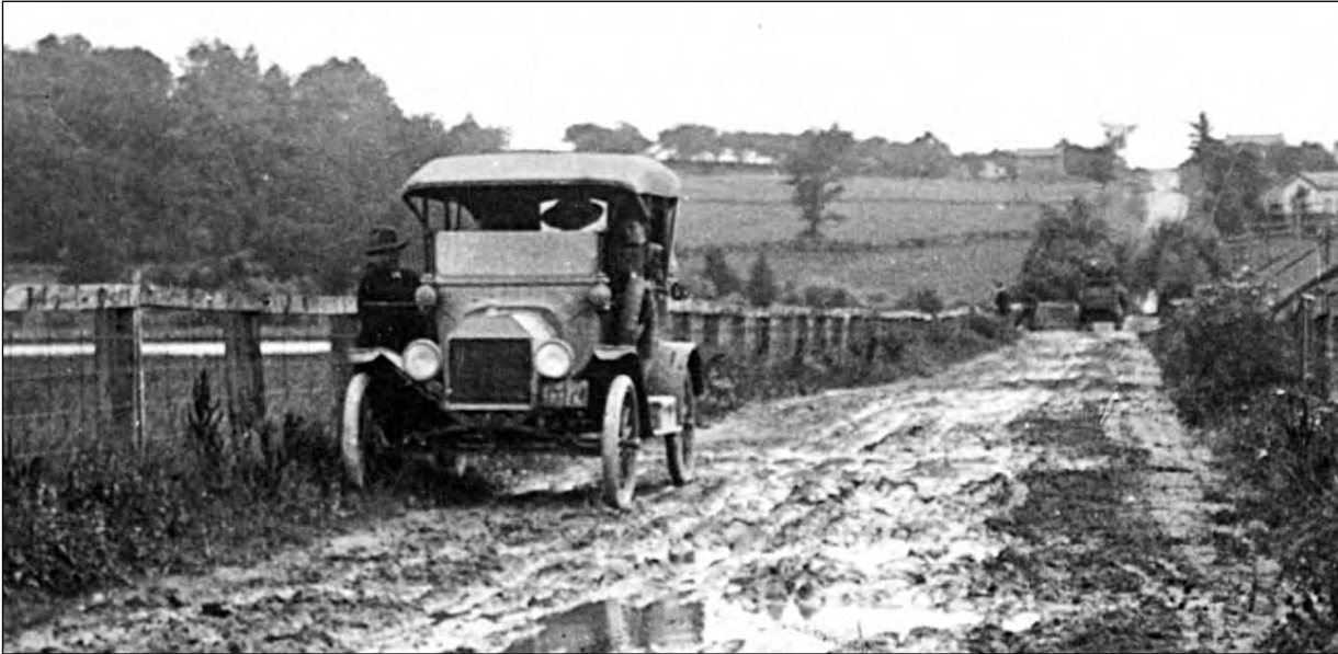
In August 1916, the Scugog Bridge was to be repaired with $800 spent on improvements, including 500 loads of crushed stone.
