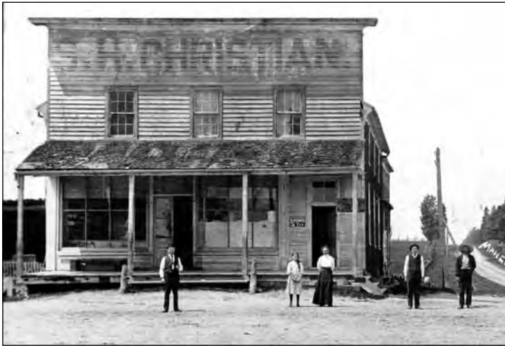
The former general store of Samuel H. Christian, at Manchester.
