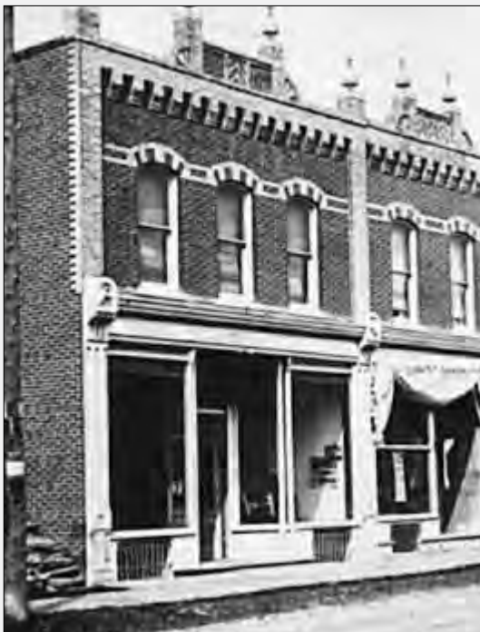
Royal Theatre located in Jessop Block, 235 Queen St.
