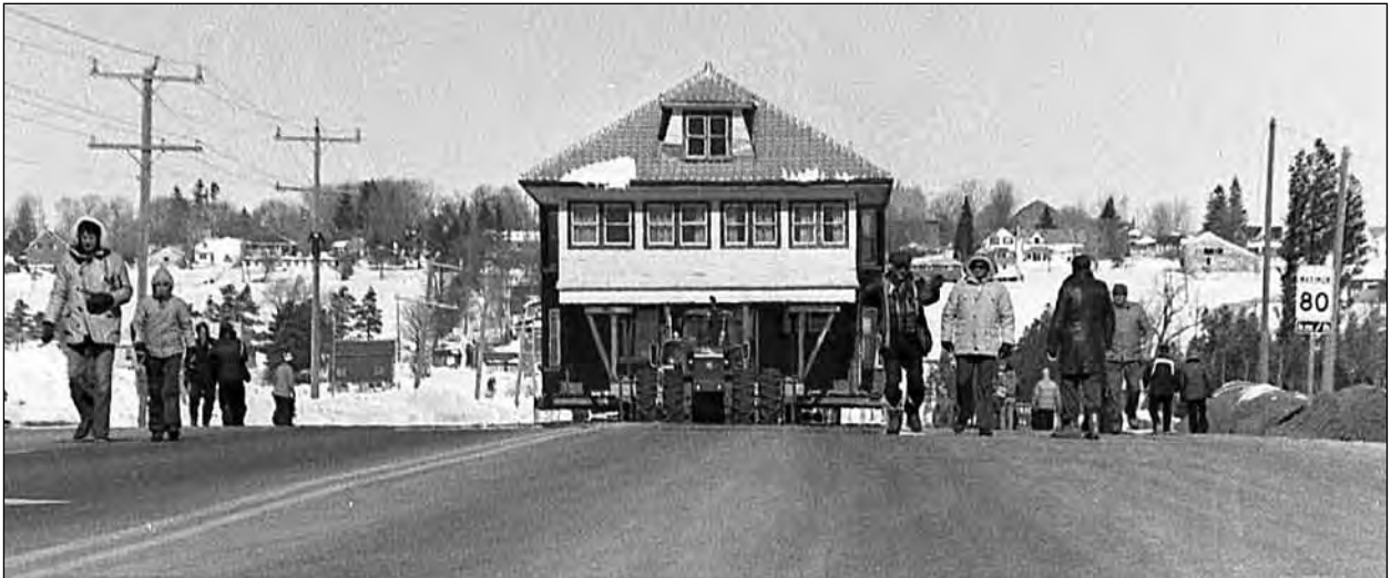
This was the scene on March 25, 1982 as a two-storey house owned by Dr. Morley Pitts, was moved from Greenbank, three miles south of the village to a new lot on Concession 9. The move took five hours to complete and cost about $100,000.
