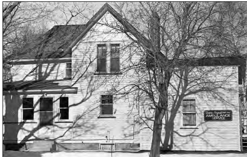
The Charles Brignall Ambulance Service was located in this building just east of the municipal office before being purchased by the township.
