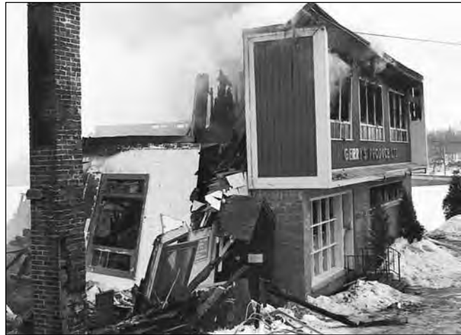
Burnt out remains of Gerry's Produce following the fire.
