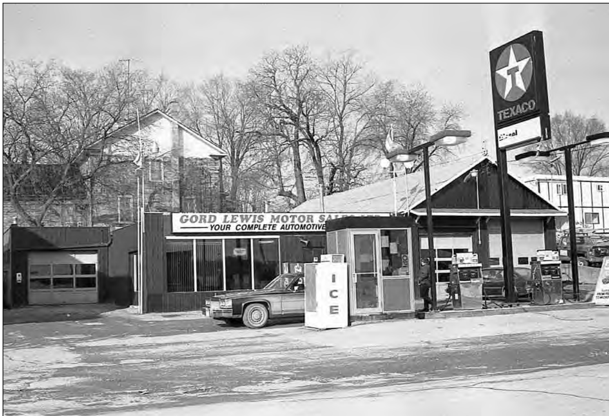
Gord Lewis Motors Sales was located in this Water Street garage, at the corner of Casimir Street, in March 1989. The building still remains today, one of the few original buildings along this stretch of Water Street.
