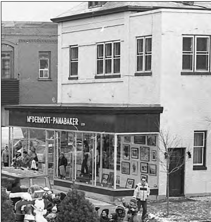
McDermott-Panabaker Funeral Home at the corner of Queen and Perry Street featured a glassed-in furniture showroom facing onto the street until December 1981 when new owner, Harold Wagg, opened The Wagg Gallery in the space, featuring the work of local artists.
