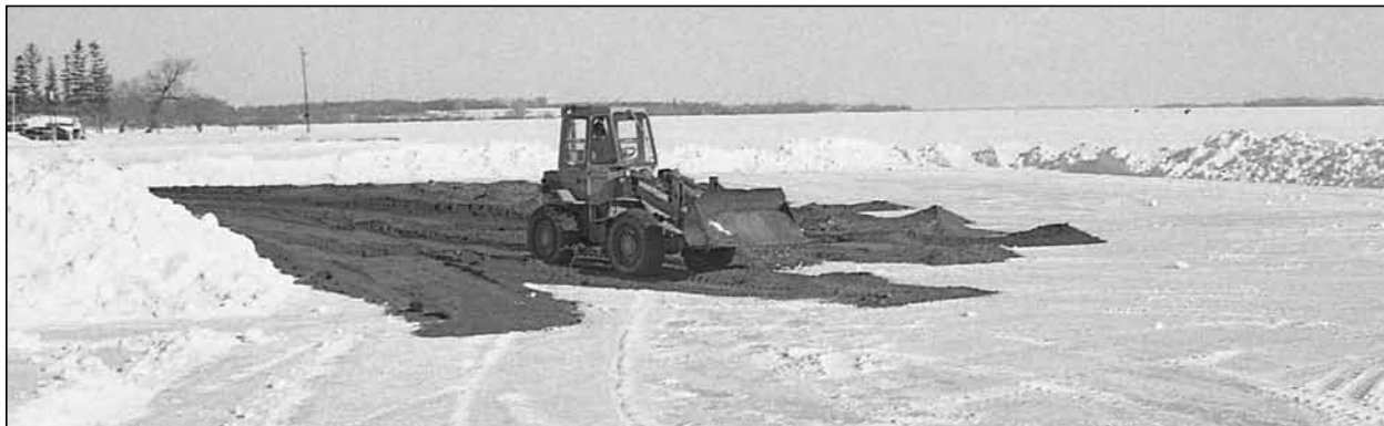
Scugog Township works department had a grader out on the Lake Scugog ice in early March 1982, clearing an area around the lakefront beach. After removing the snow, tons and tons of sand were dumped along the beach and spread over the ice. This new sand will sink to the bottom when spring thaw comes, making the bottom of the "old swimming hole" cleaner. Above, the sand is being spread over the ice by one of the township workers.
