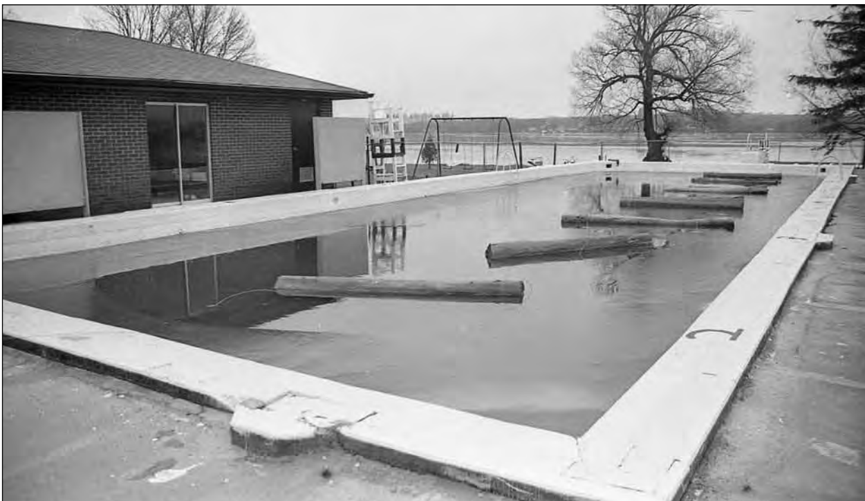
The original Birdseye Pool, seen here winterized in December 1982, was in serious condition and in need of repairs. Scugog council gave authorization to go ahead with $14,000 in repairs to the pool if the Regional Health Department agrees it will bring it back to standards. The main work will include raising the concrete deck around the pool to bring it level with the lip of the pool. If all goes according to plan, the township hopes the pool will be open again next summer.
