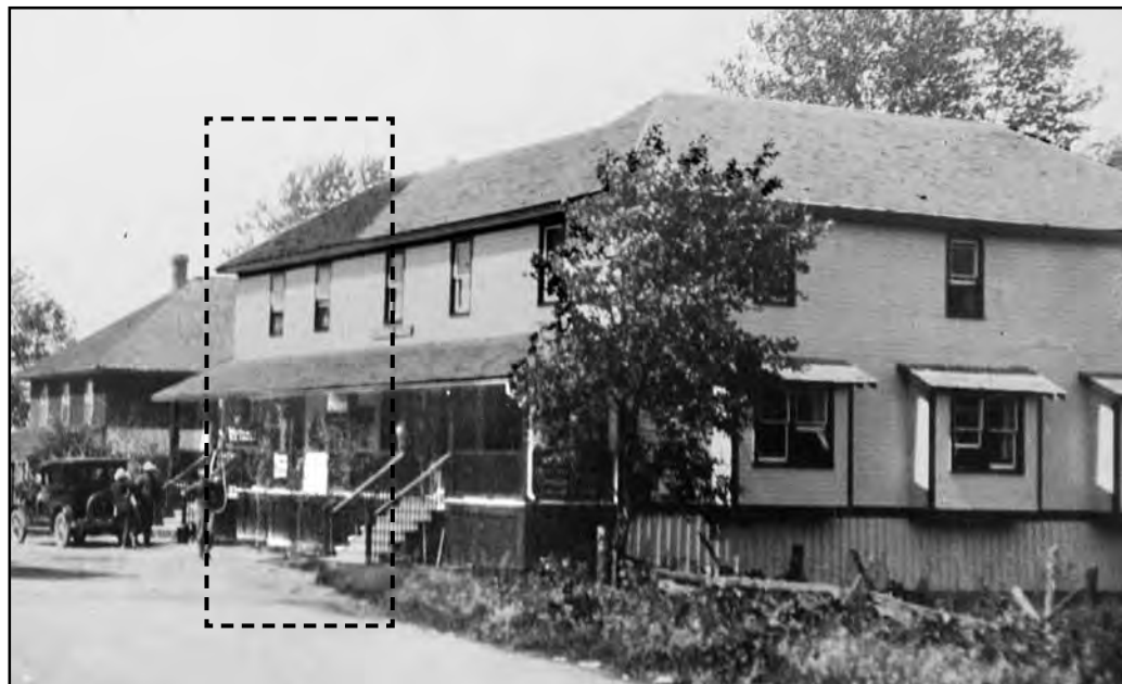
Lakeview House, far left, with the post office (above) combined into the new large building, area outlined.
