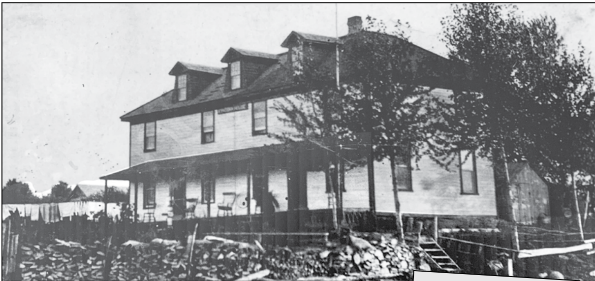
This photo of the Kenosha (Kynosha) House Annex was taken about 1908.
