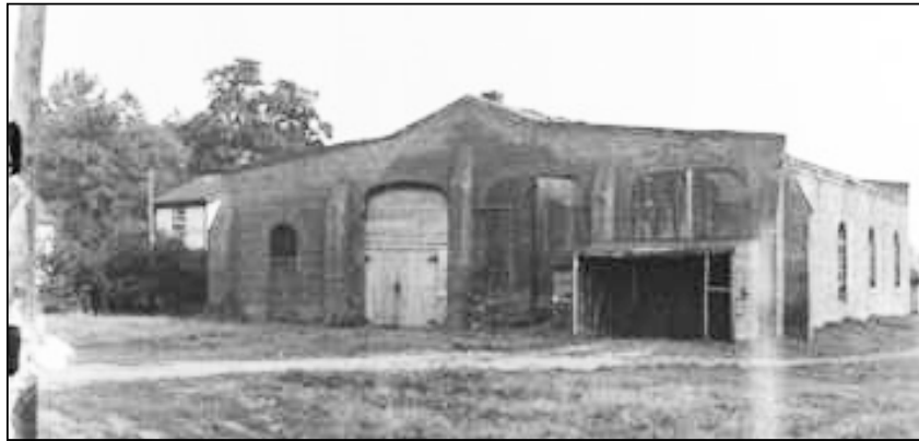
The PW&PPR Engine House, northeast of Uptown Station, above.
