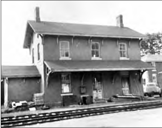
Whitby station prior to demolition.
