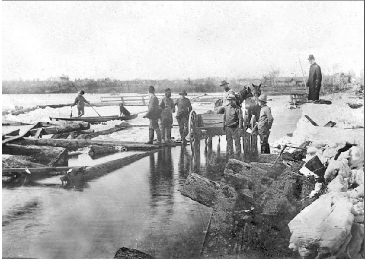
Men begin repairs to the Lake Scugog floating bridge following extensive damage from ice during a spring breakup, circa 1876.
