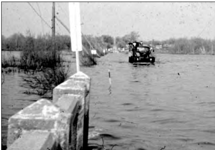
A cement pier, bottom left, of the concrete bridge constructed in 1928, which replaced a part the old wooden bridge.
