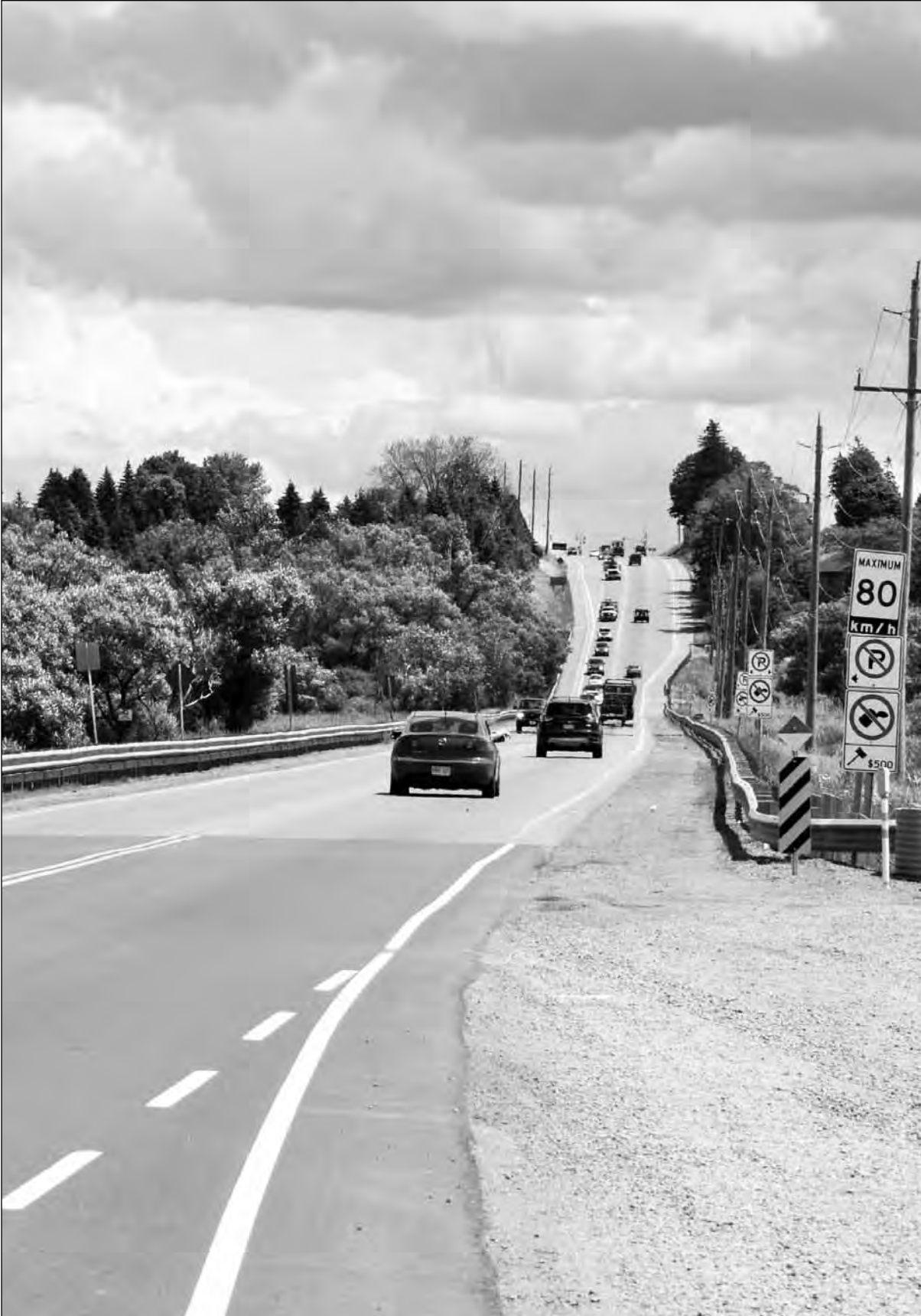
The west causeway linking Port Perry with Scugog Island - June 2017.
