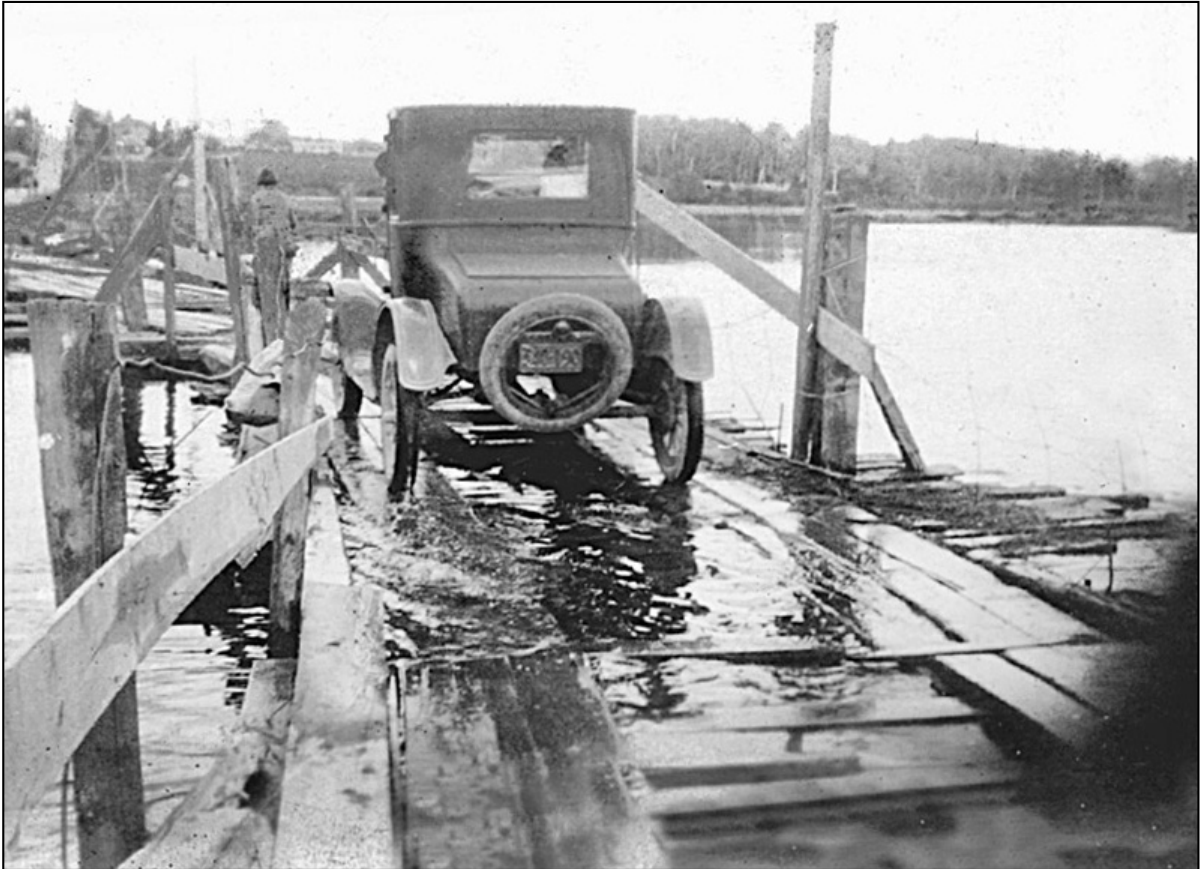
A car carefully makes its way across the floating detour, during construction on the bridge in 1928.
