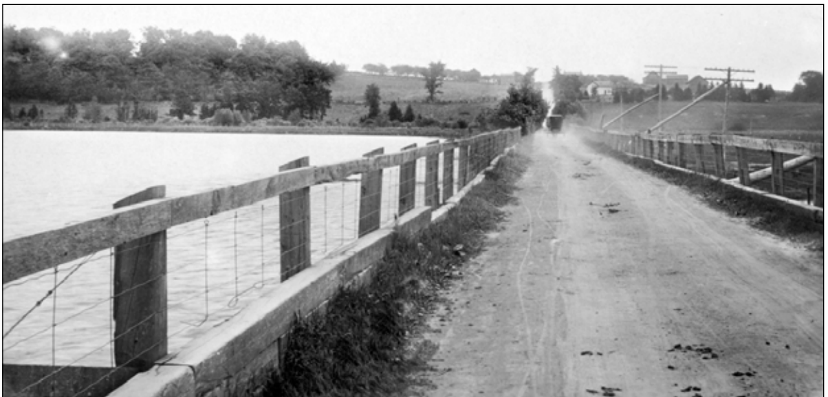
The Scugog Bridge, lined with a protective fence, as it looked during the summer in the early 1920s.
