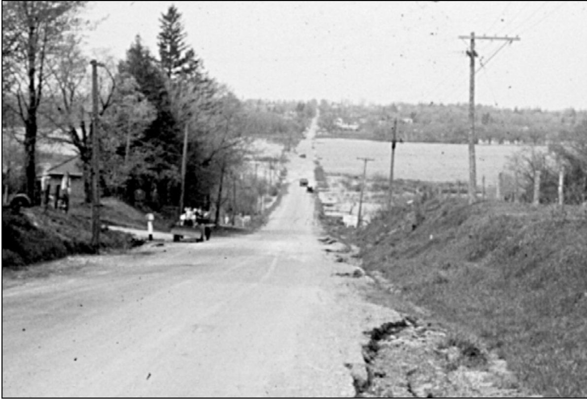
This view from the top of Scugog Island hill, shows the washed-out condition of road on the hill and construction under-way on widening and raising the roadbed, further west on the causeway, near Port Perry.
