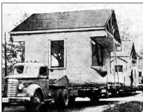
Sections of the munitions plant from Ajax being moved by trucks to Port Perry in 1949.
