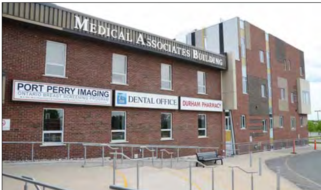
North side of Medical Associates Building, looking west towards parking lot.
