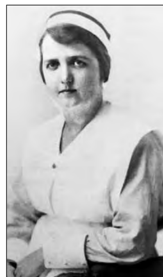
Nellie Whitmore took over the hospital in 1930 and operated from here until 1946.
