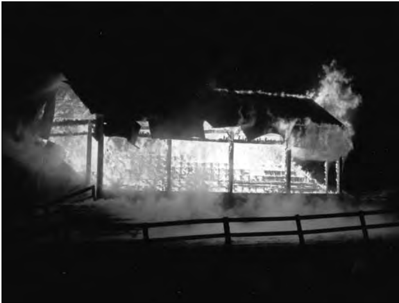
The grandstand at Blackstock fairgrounds erupts in waves of flames on a Saturday night December 14, 1996. It is believed arson is the cause of the fire, which totally destroyed the structure, which was built on the property in the mid-1930s. The grandstand had suffered many times over the years at the hands of vandals. The picture was taken by Blackstock resident Fred Ford.
