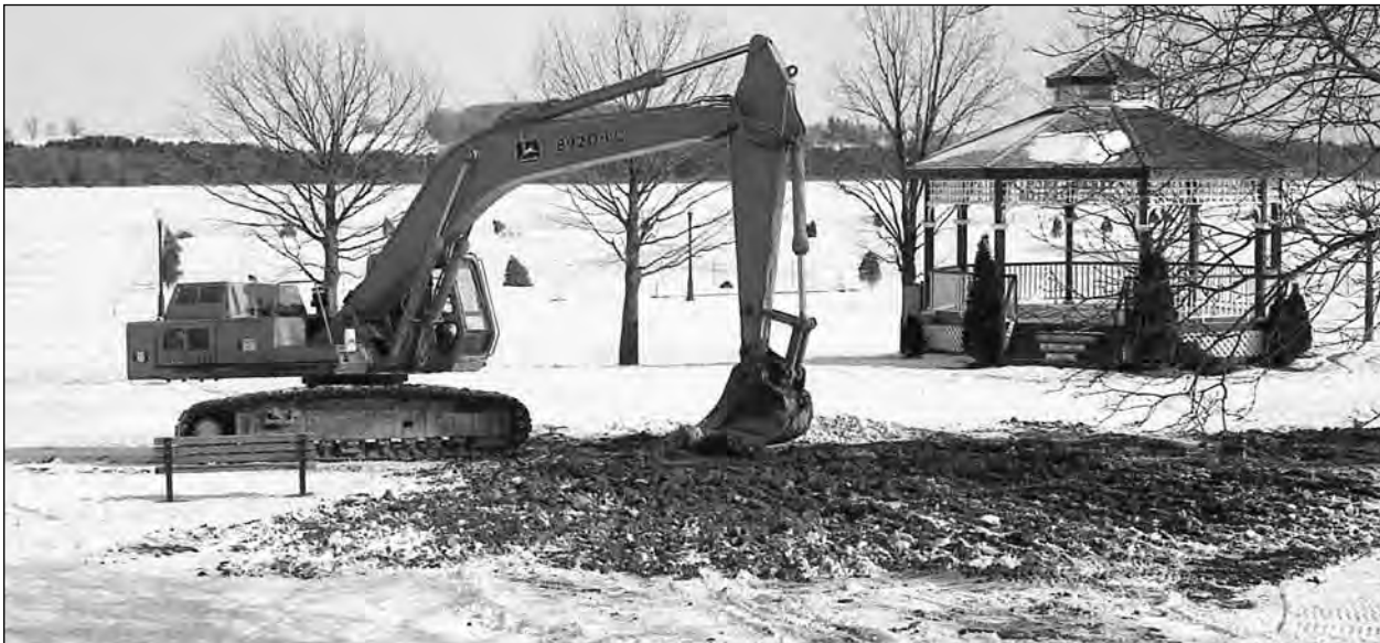
Township workers tried unsuccessfully to remove a concrete slab from the ground in Palmer Park in February 1993. The large slab had been used as a base for a water tower beside the railway station which was located in the park. Parks committee chairman Marilyn Pearce said it was being removed for cosmetic reasons. During the summer, the grass turns brown over the pad, due to the small amount of topsoil over it.
