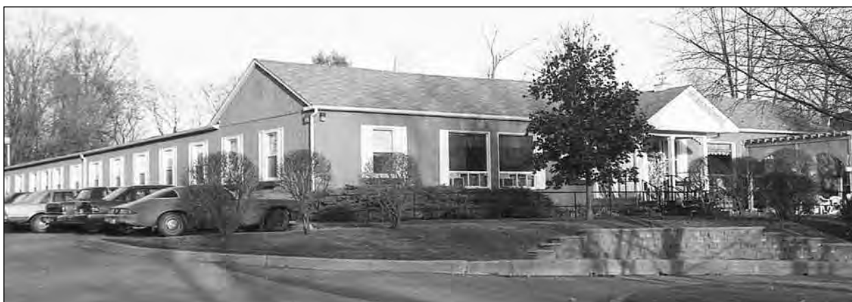
The Port Perry Villa, located beside the Port Perry Nursing Home, on Simcoe Street, November 1998.
