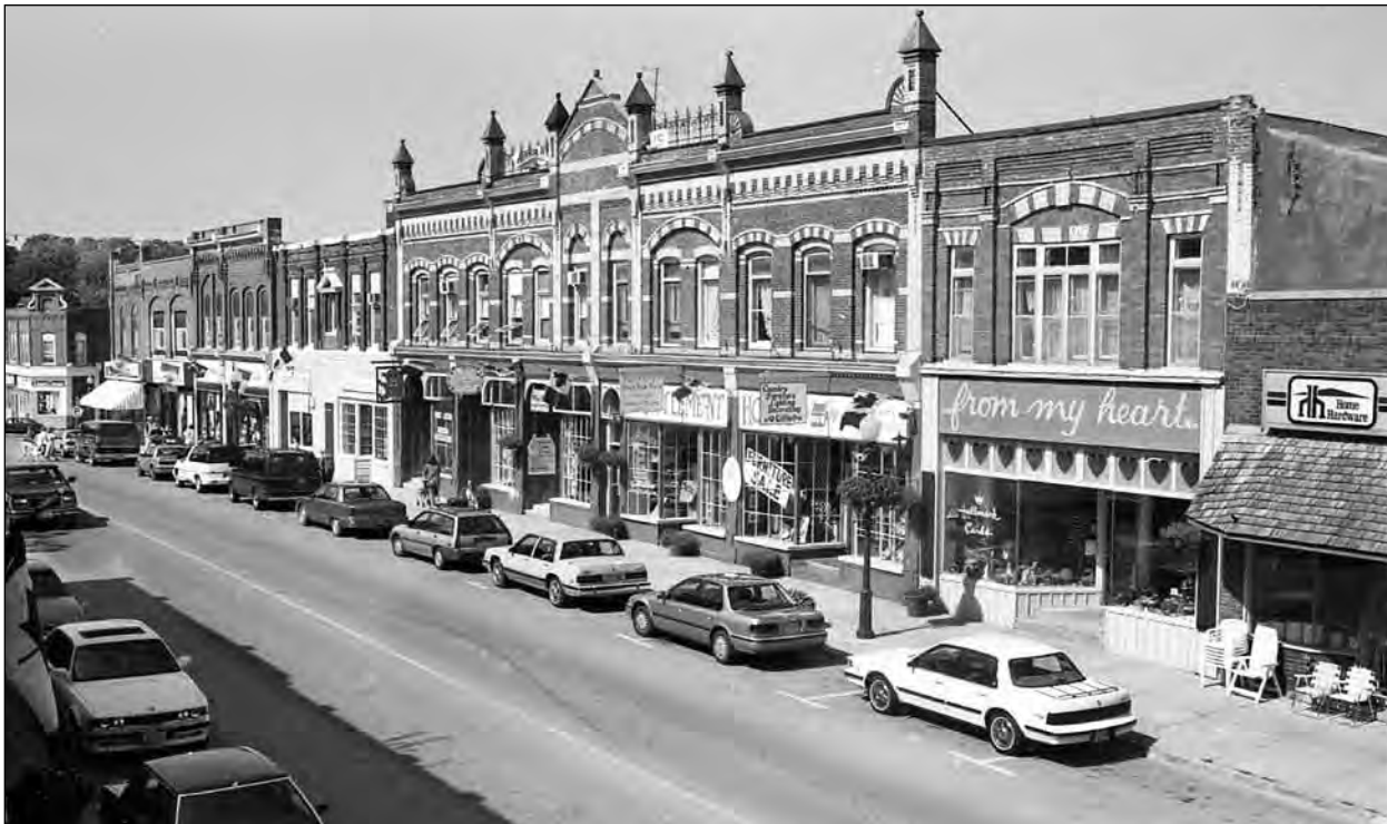
The north side of Queen Street in July 1993 with the attractive and ornate Settlement House block with its many stores.
