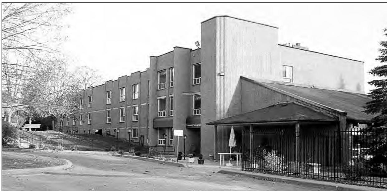
Port Perry Community Nursing Home, north entrance, November 1998.
