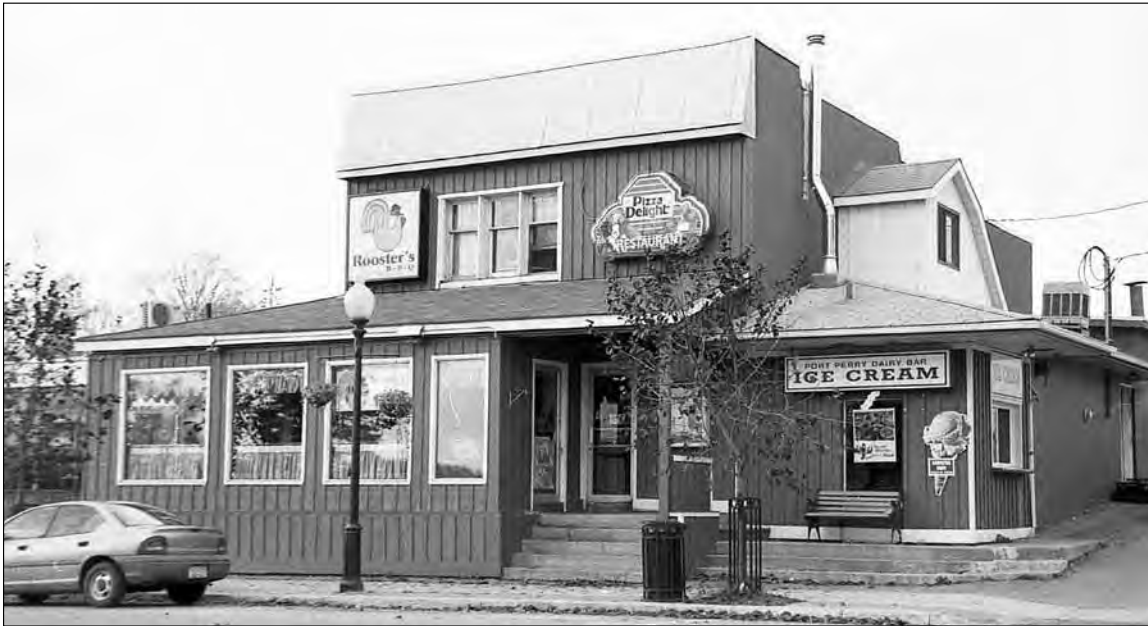
The former Port Perry Dairy building was the location of Pizza Delight in this 1998 photograph.
