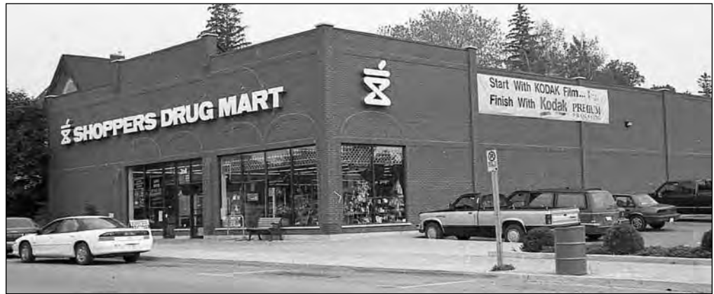
This Queen Street property was originally the location of a Chevrolet-Oldsmobile dealership. After closing, the old building was torn down and Big V Drug Store opened in the new building. It was later taken over by Shopper's Drug Mart, as seen in this 1998 picture.
