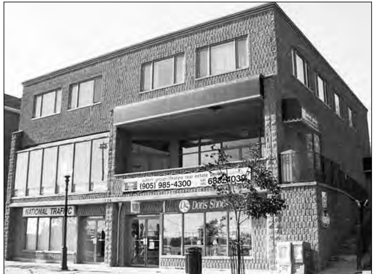
Three-storey building on Water Street was the location of National Traffic, Doris Shoes and Sutton Group Lifestyle Real Estate in this fall 1998 picture.
