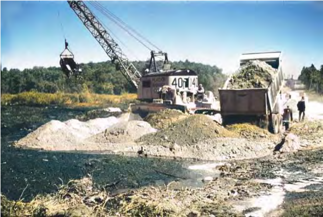
Construction finally got underway in August 1960. The existing causeways were both closed as the adjacent marsh was excavated up to 20 feet deep in order to insure a proper foundation for the permanent roadway.
