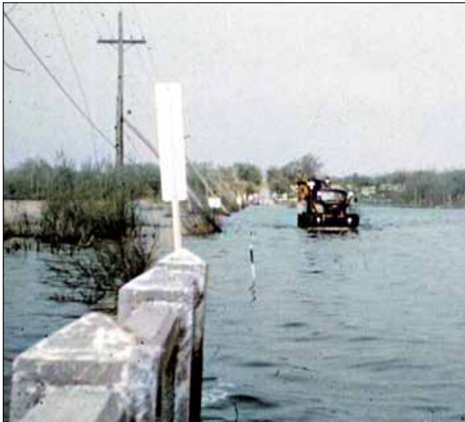
A cement pier, bottom left, of the concrete bridge constructed in 1928, which replaced a part the old wooden bridge.
