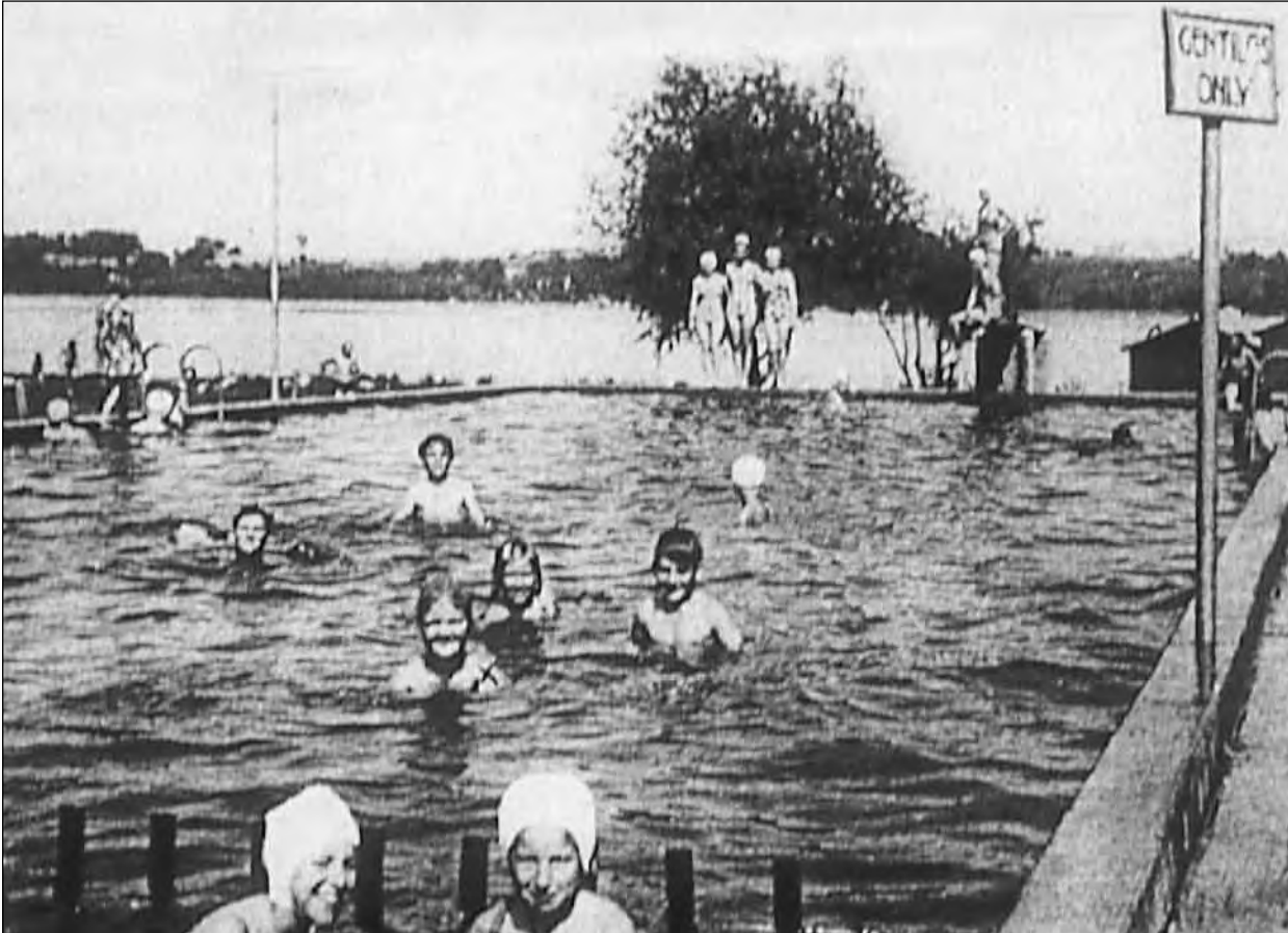
This picture of the Birdeye Pool must have taken in early 1940, before the bath house was built at the end of the pool nearest the lake. What is interesting about this picture is the sign posted on the pole with "Gentiles Only" thus restricting anyone who was Jewish. This sign does not appear at any other time.
