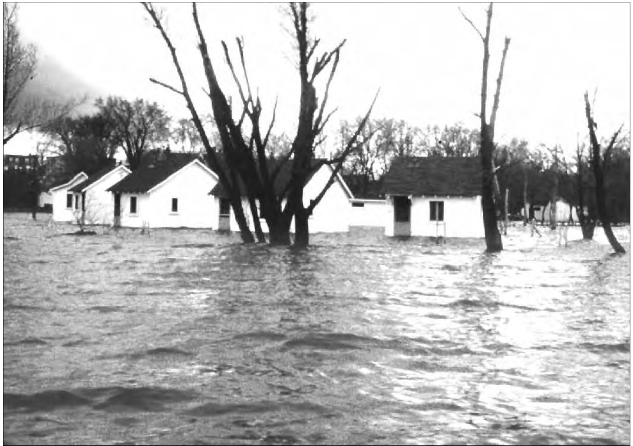
The property on which Birdseye Centre is not much above the level of Lake Scugog, so is prone to flooding in the spring. This picture, about 1945, shows the cabins flooded during one of those high water seasons.
