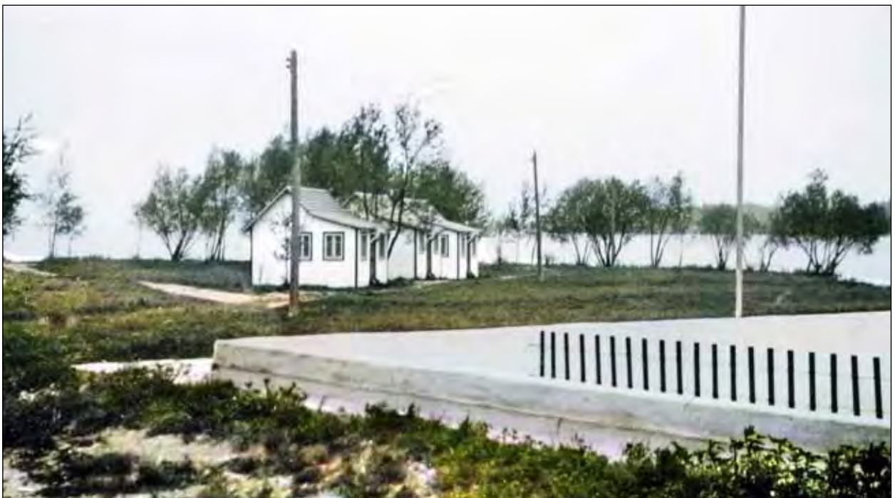
Work got underway on Birdseye Centre Cabin Park in the fall of 1939. This picture shows a corner of the pool with three of the cabins behind. Eddie Michell purchased his first three cabins from another park and had them moved to his site.
