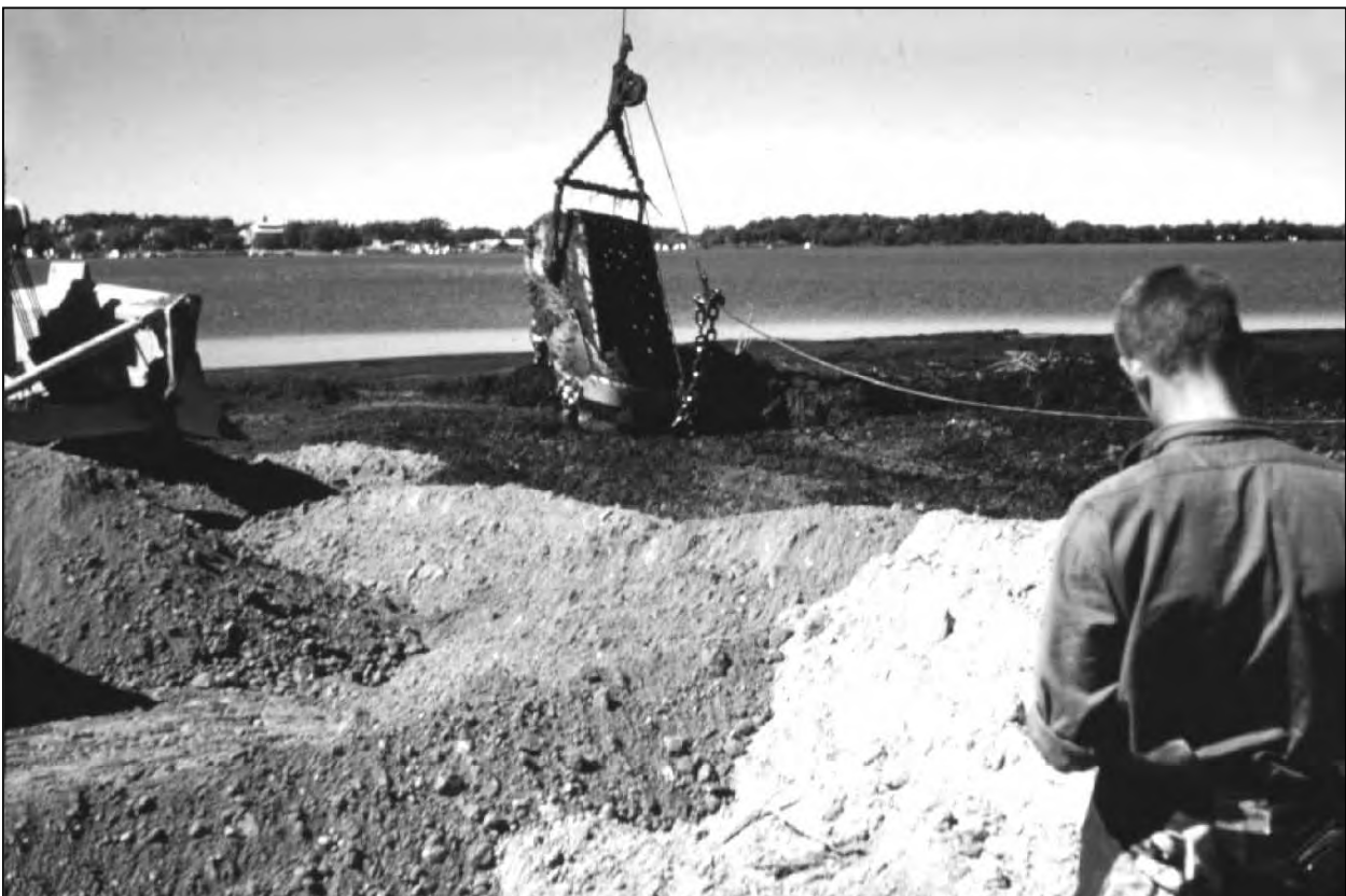
Construction finally got underway in August 1960. The existing causeways were both closed as the adjacent marsh was excavated up to 20 feet deep in order to insure a proper foundation for the permanent roadway.
