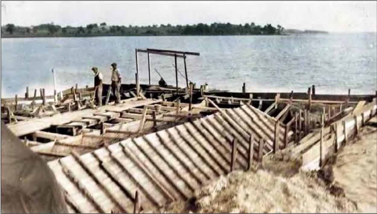
These pictures, taken in 1925, show the framing and construction of the cement dock and entrance to the boathouse at Seven Mile Island.
