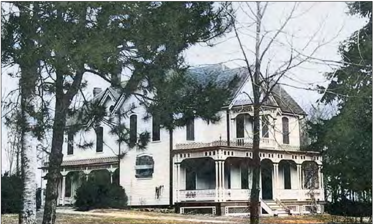
This large frame house was built by Jonathan Blong during the late 1800s, at his Beechcroft property, and later became the Kent family home. It still stands today on 434 Lakeshore Drive, Port Perry.
