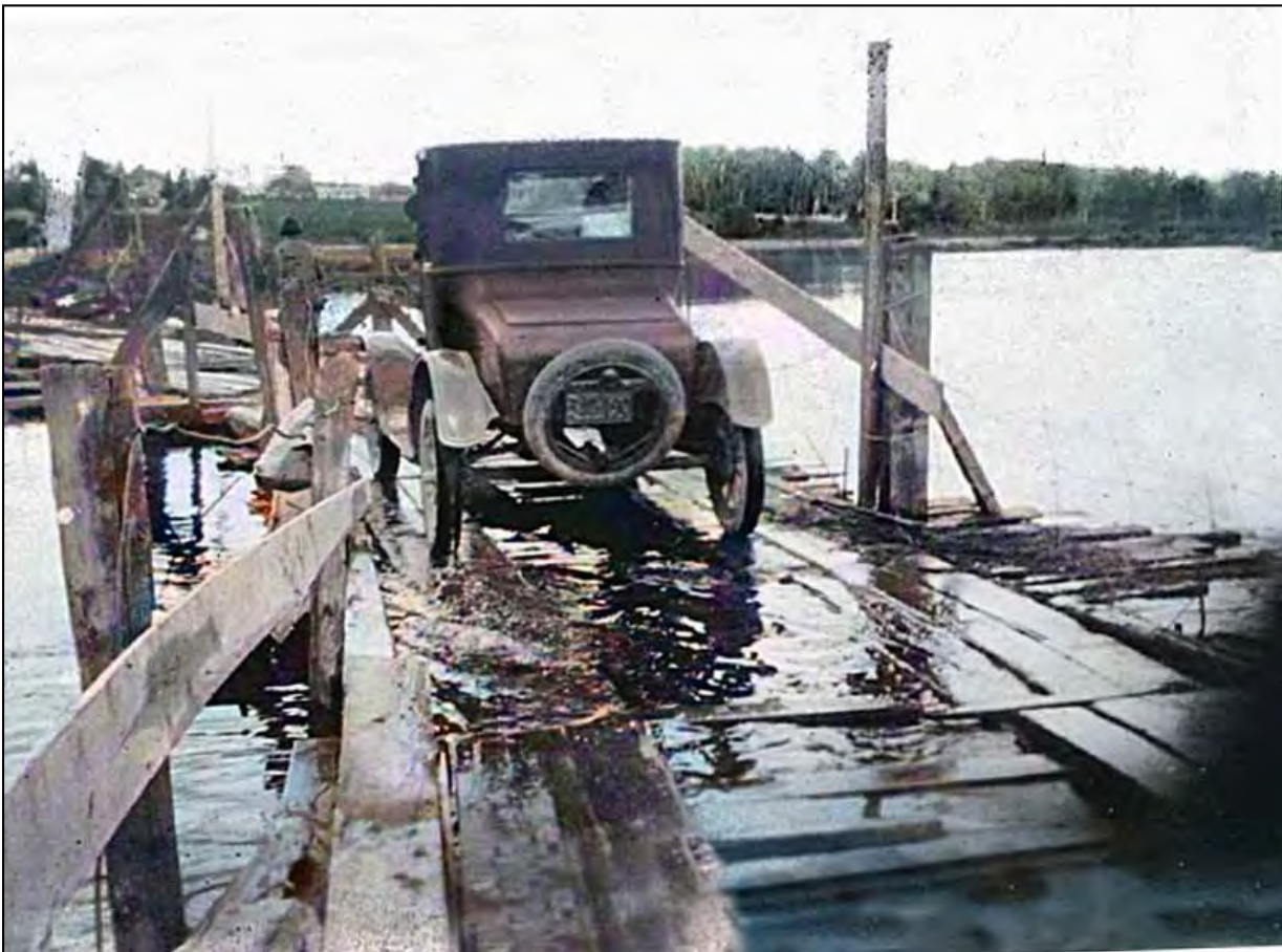
A car carefully makes its way across the floating detour, during construction on the bridge in 1928.
