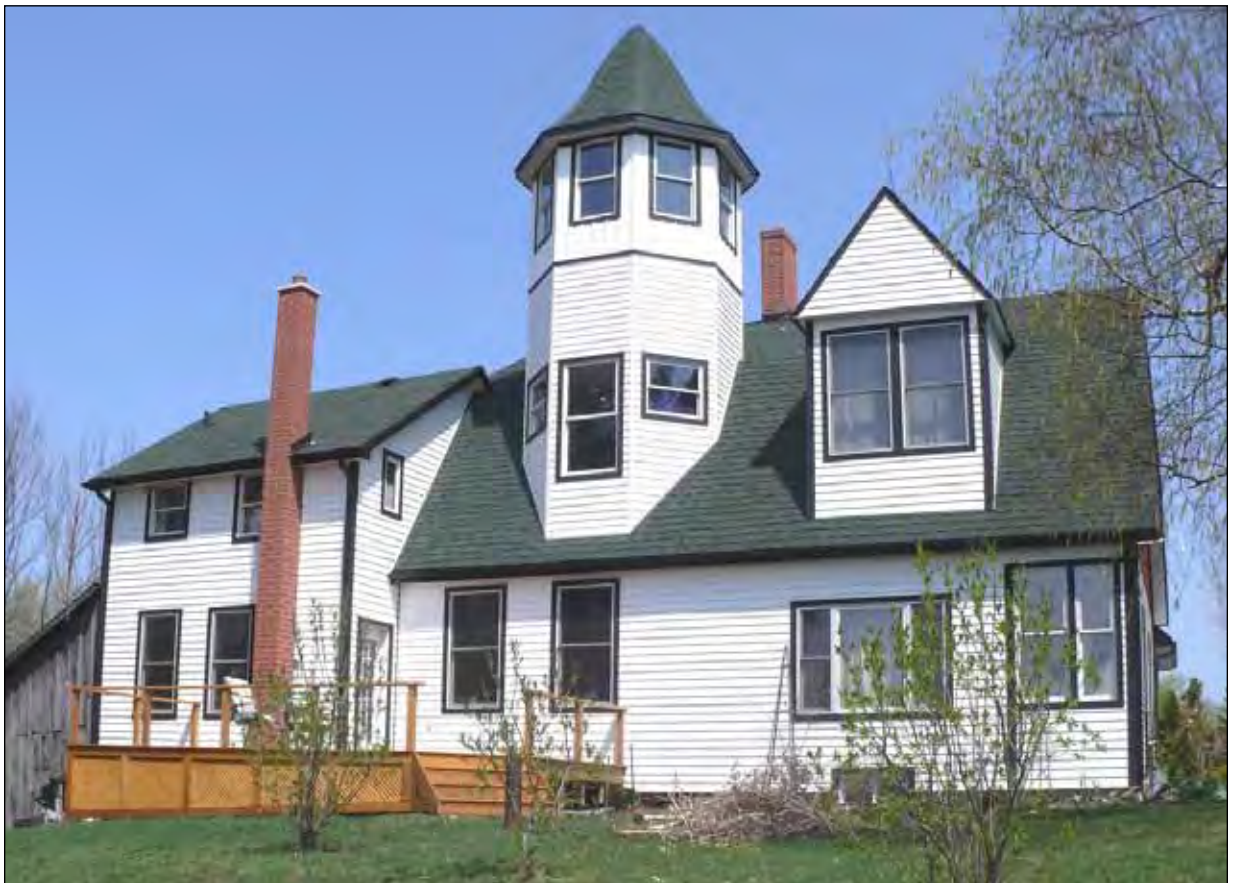
The Osler's clubhouse and caretakers residence after renovations in 2008.
