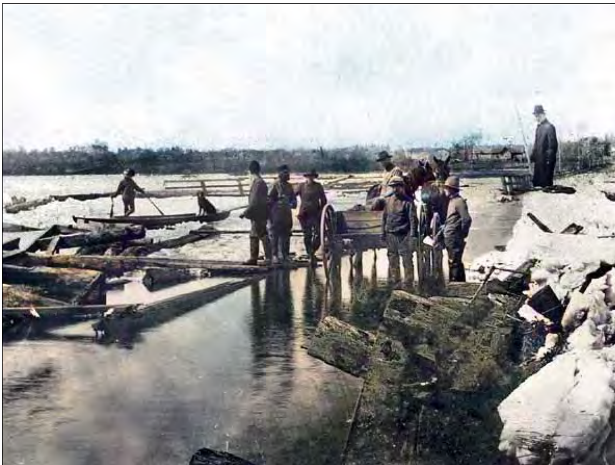
Men begin repairs to the Lake Scugog floating bridge following extensive damage from ice during a spring breakup, circa 1876.
