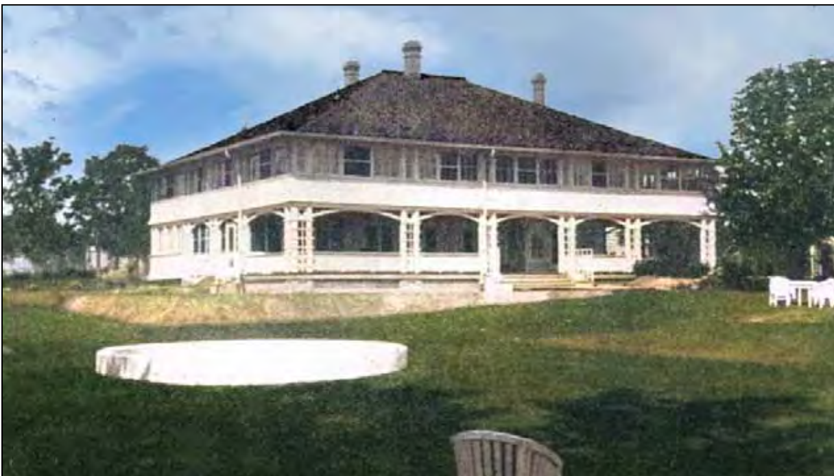
The Wilson's main residential building was impressively set on a large manicured lawn. The 5,200 sq. ft. two storey house, enlarged from Delmont Cottage (page 4) had four fireplaces, eight bedrooms, a den, large kitchen and livingroom.
