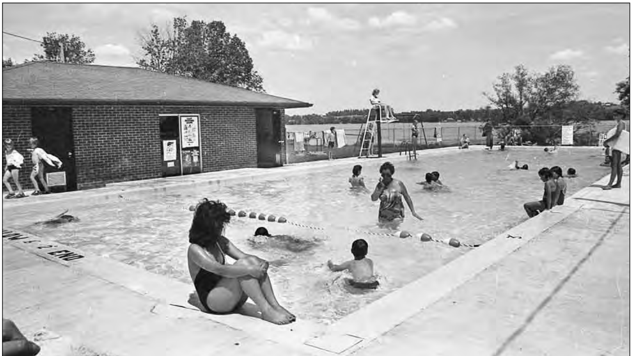
Birdseye Pool as it looked in 1985, after the change rooms had been re-located to the north side of the pool. This picture was taken about 19 years before it was removed in 1999.
