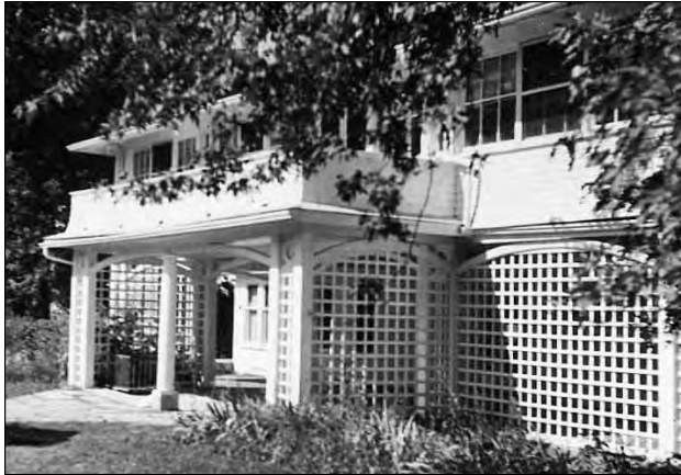
The south entrance to the main residence, about 1948.
