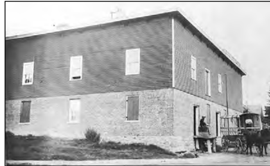
Port Perry Creamery, on Perry Street, Port Perry.
