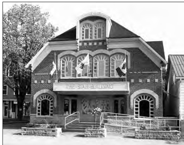
The new Star Building at 188 Mary St., 1991.
