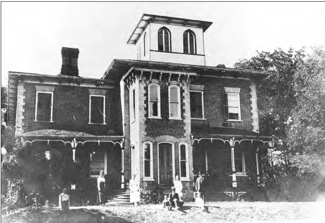
Beuna Vista, the home of William and Lurana McGill, located in north Port Perry near Lake Scugog.
