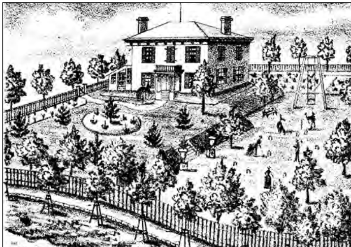
Residence of Hubert L. Ebbels, Cochrane St., Port Perry.
