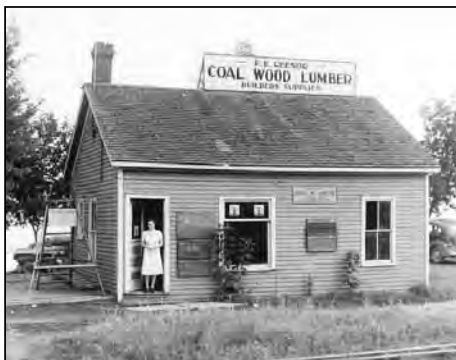
Fred E. Reesor, Coal, Wood & Lumber office 1930s.
