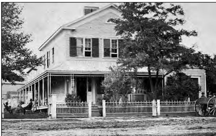
William Sexton's home on Water St., across from the Currie Grain Elevator.
