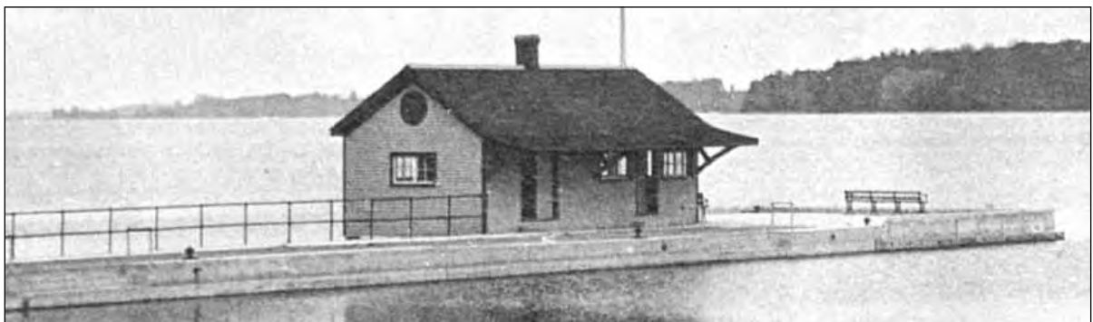
Charles Vickery constructed the lakefront wharf in 1914-15. The dockhouse was added about 1918.
