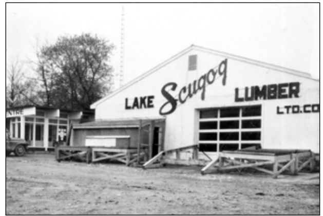
Lake Scugog Lumber was located at the north end of Water Street, beside the lake and Birdseye Centre Park.
