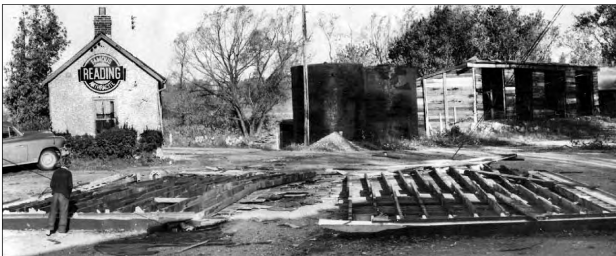
The roof of the home of Mr. and Mrs. Philip Orde can be seen laying on the ground, removed by winds of Hurricane Hazel.
