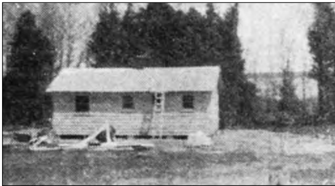
One of the cottages under construction.
