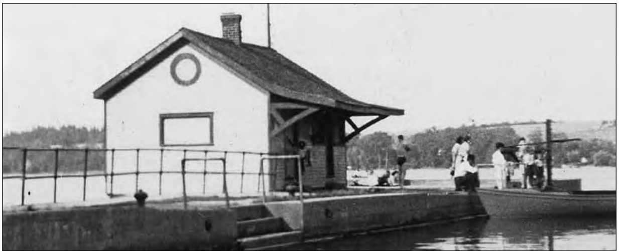
The dock house, or wharf house, located at the end of the government wharf, before it deteriorated.
