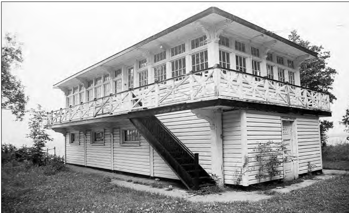
The two-storey boathouse was located at the south end of the island on the shoreline of Lake Scugog. The second floor was surrounded by 35 large windows lighting the spacious room, below, which featured a dance floor.
