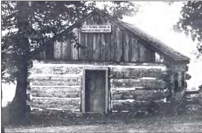
* Example of the type of primitive log school houses built in Ontario during the early 1800s.
