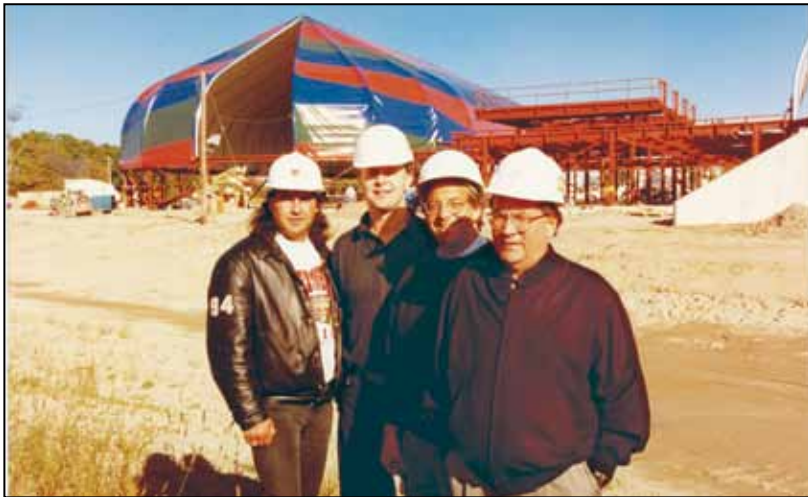
Work was progressing quickly on the Great Blue Heron Casino and Bingo complex in October 1996 when Chief Gary Edgar, right, toured the site. With him are, from left, Sean Eade, Thomas Kelineer and Ron Steiner.
