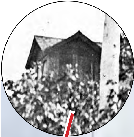
A portion of the roofline of the fire hose tower, at the rear of the Town Hall.
