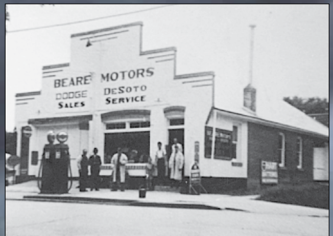
The upper structure of the Beare Motors building, at the corner of Queen and John Streets, was toppled to the ground, during a storm in December 1919, killing one and injuring two others.
