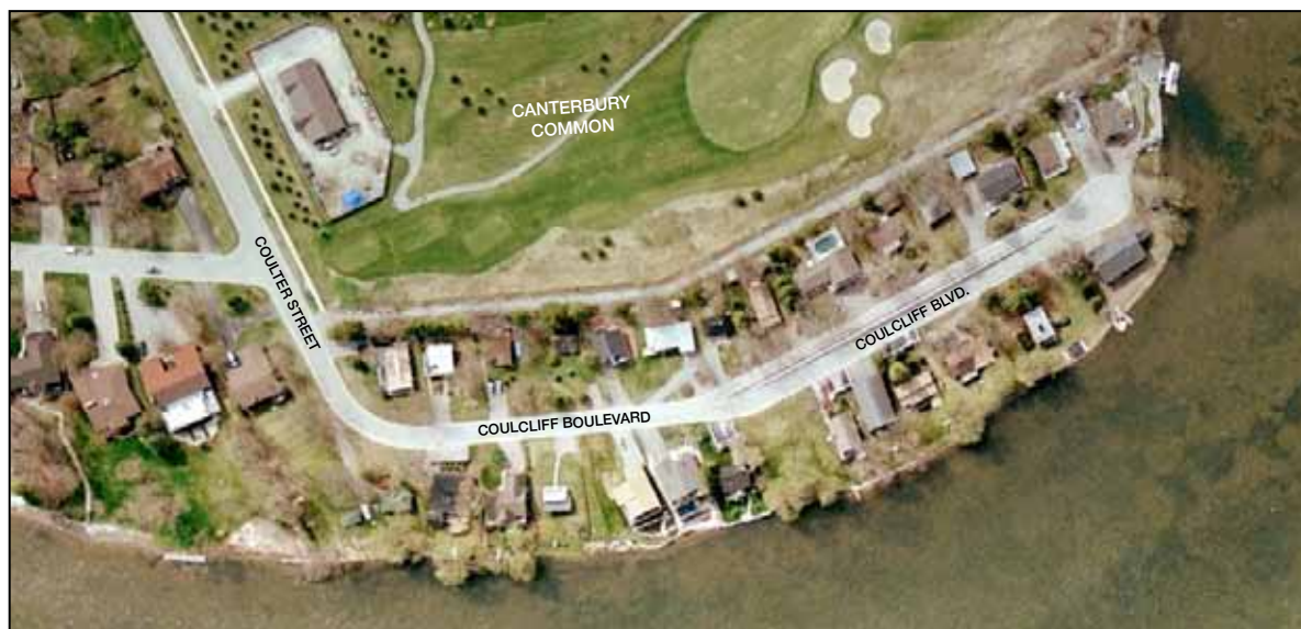
Aerial view of Highland Beach, from Google Earth, shows the homes and cottages along Coulcliff Boulevard.
