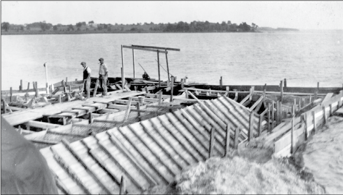
These pictures, taken in 1925, show the framing and construction of the cement dock and entrance to the boathouse at Seven Mile Island.
