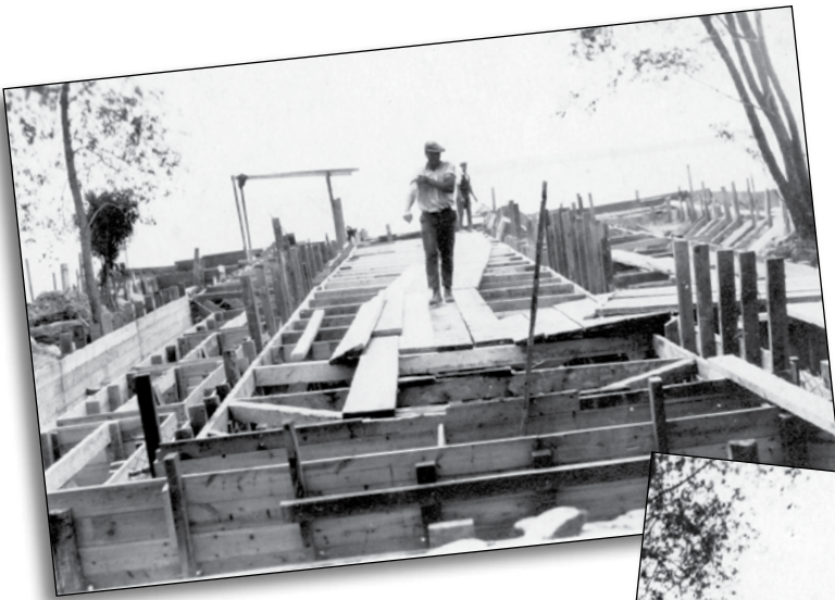
These pictures, taken in 1925, show the framing and construction of the cement dock and entrance to the boathouse at Seven Mile Island.
