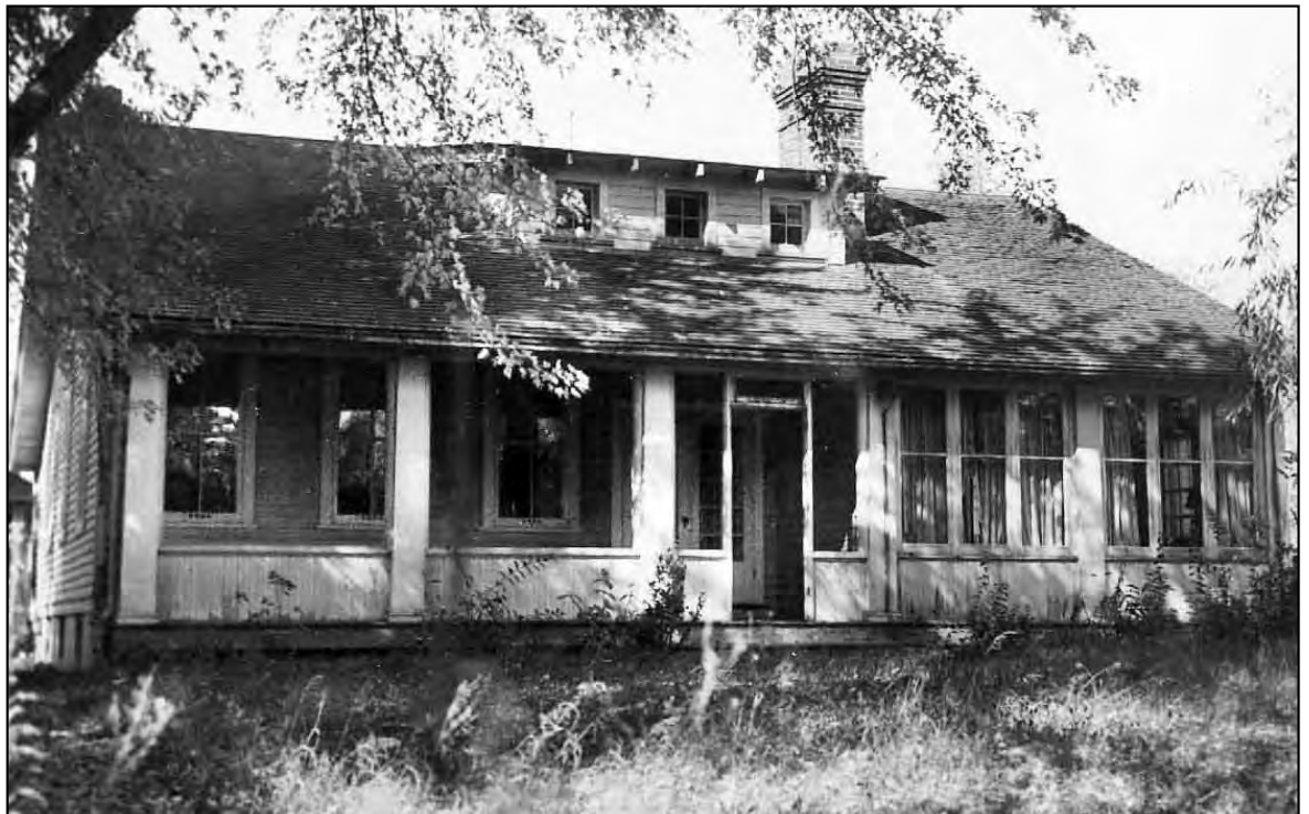
This building photographed in 1948, became the summer residence of Harry and Freda Ely.
