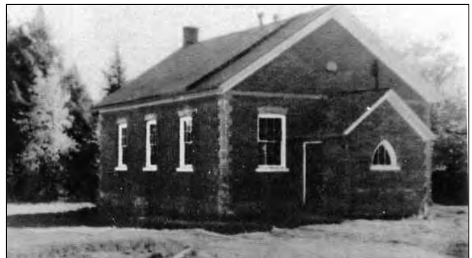
A view of the front and entrance of the Bethesda SS #1 school.
