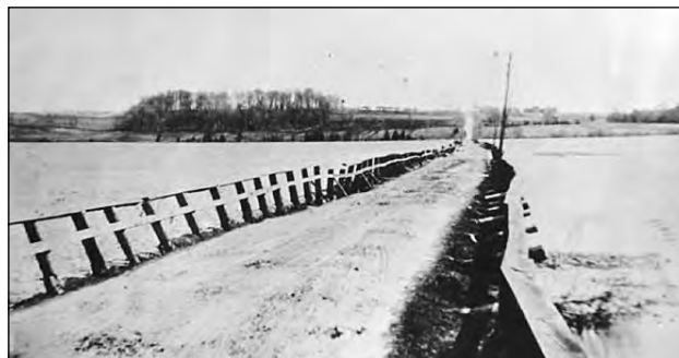
The Scugog Bridge after being made permanent.
