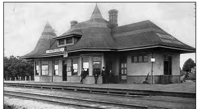
The Grand Trunk Railway's Whitby Junction Station.
