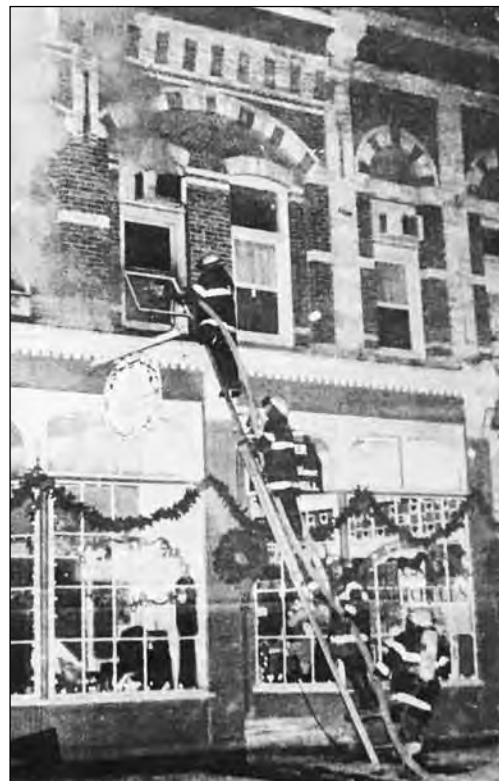
Fireman scale a ladder to get at a fire which started in an apartment above Settlement House, in downtown Port Perry. The fire threatened to destroy one of Port Perry's landmark buildings, constructed in 1885.
