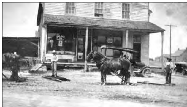
Haggerman's store at corner in Manchester.
