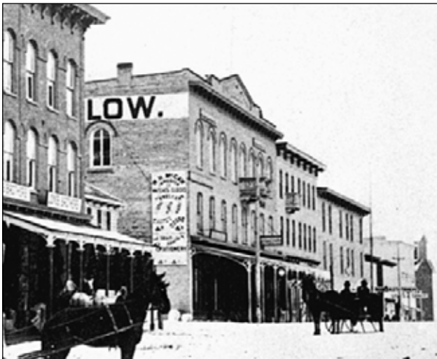
Section of Port Perry destroyed by fire in November 1883.
