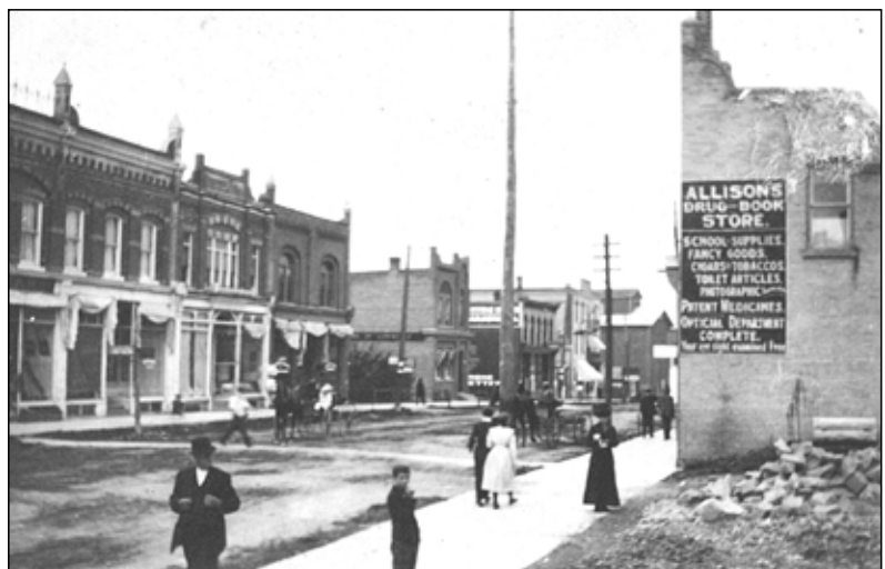
Allison's Drug Store building destroyed in 1897 fire.
