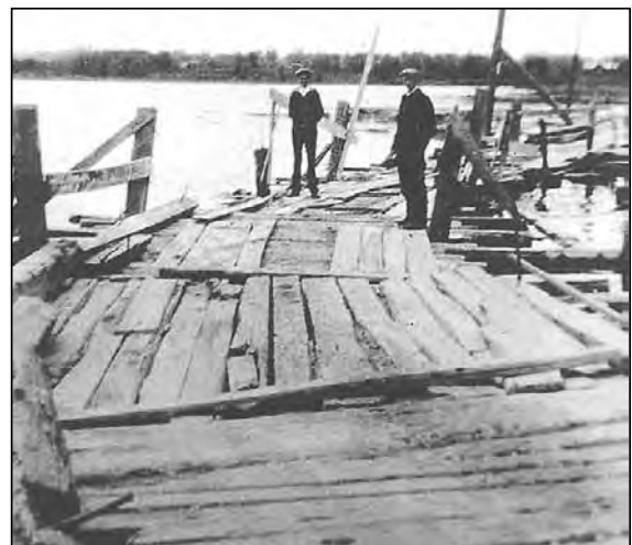
Scugog Floating Bridge.
