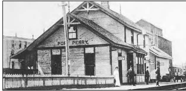
The new Port Perry Railway Station.
