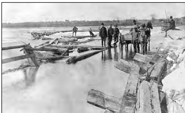
Scugog Bridge ice damage.
