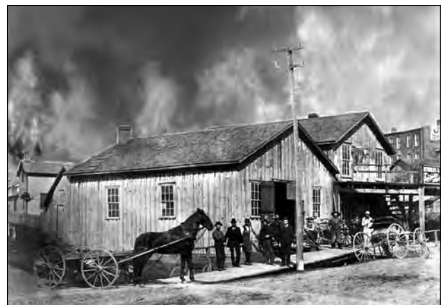
Carriage Works buildings on Perry Street.
