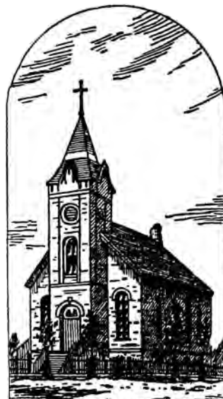
Catholic Church, John St., Port Perry.
