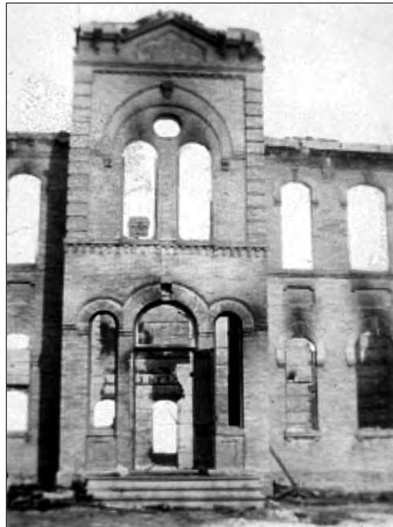
The entrance and tower of the Public & High School.
