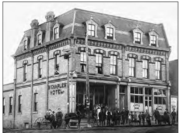
St. Charles Hotel, Queen Street, Port Perry.
