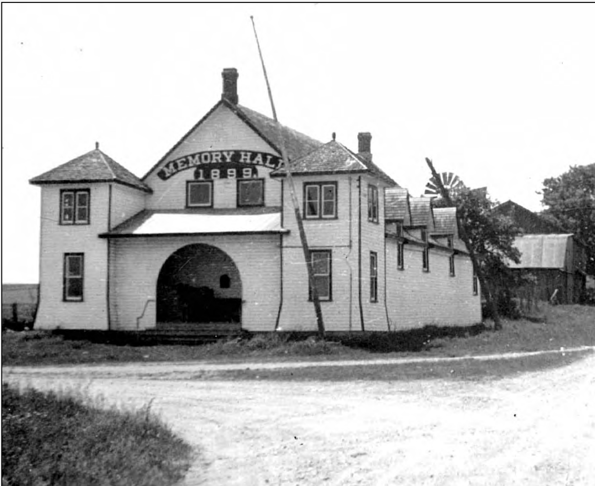
The Utica Hall was built by Thomas Horn as a gift to the people of his home town. It was officially opened on December 1, 1899.
