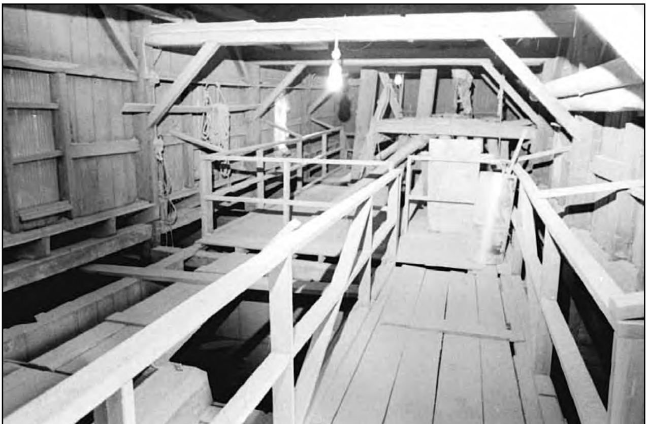
The headhouse (cupola) at the top of the elevator stretched over a series of about 18 grain bins, which were 30 feet deep. Upper picture shows an elevated view looking down through the beams to the "bin deck" walkways which are the same level as the top of the bins. Bottom picture shows the walkways and handrails in the "bin deck" which allowed access to equipment located over top of the bins.
