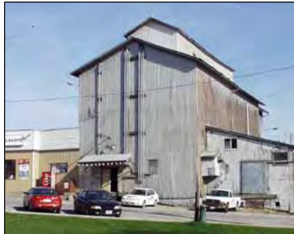
Elevator looking north from Palmer Park.
