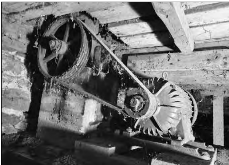
This heavy motor powered the auger which raised grain from the main floor to the turnheads in the cupola at the top of the elevator.
