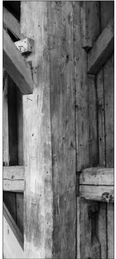
Huge posts and beams, some as large as 10"x 10" in size, helped provide the strength of the structure.
