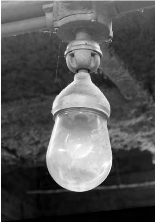
One of the many old light fixtures found throughout the elevator.
