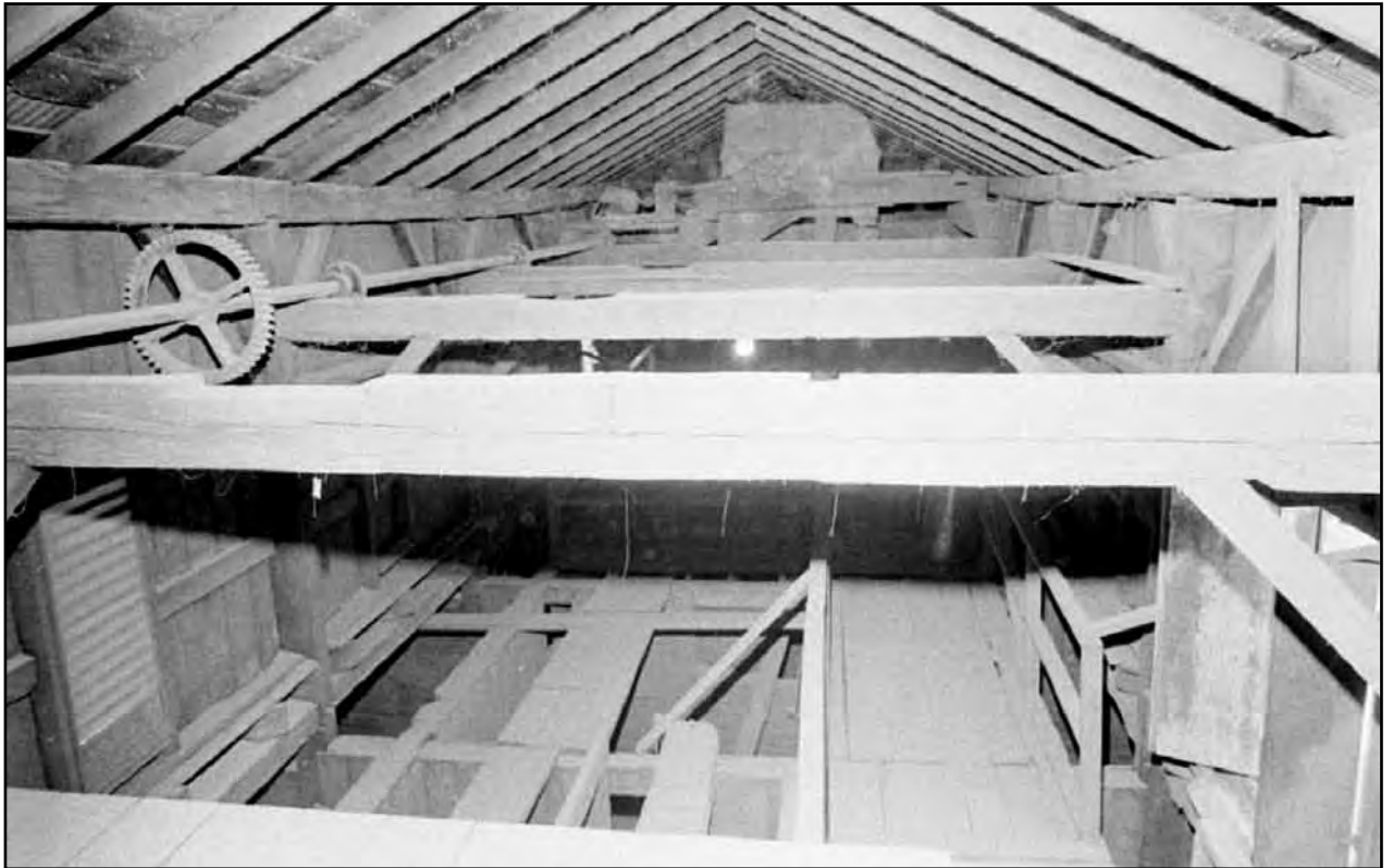
The headhouse (cupola) at the top of the elevator stretched over a series of about 18 grain bins, which were 30 feet deep. Upper picture shows an elevated view looking down through the beams to the "bin deck" walkways which are the same level as the top of the bins. Bottom picture shows the walkways and handrails in the "bin deck" which allowed access to equipment located over top of the bins.
