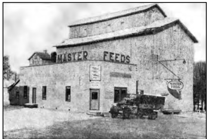
Master Feed's grain elevator June 1949
