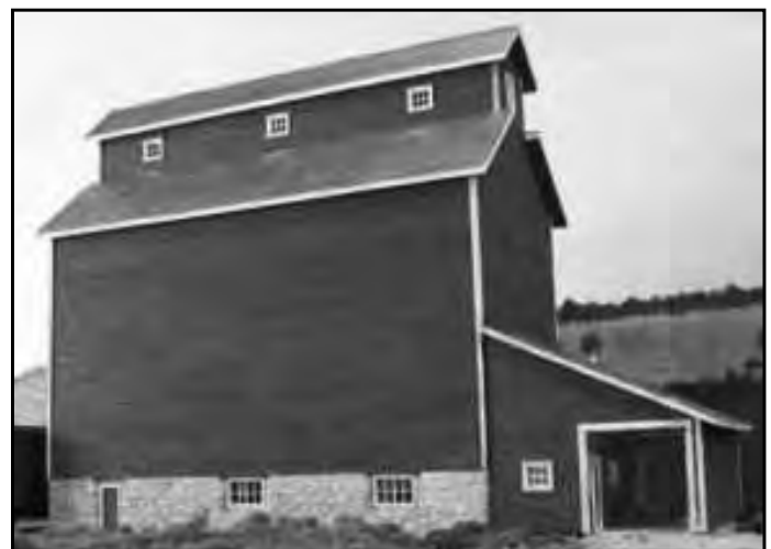
Eastern Grain Elevators were constructed in a more rectangular in shape.
