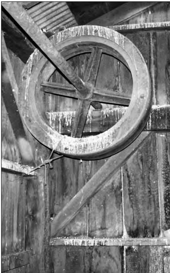
This large wooden pulley, left, and cogged wheel, above, have been standing idle for almost a century. They were used during the early days of the elevators operation to bring grain to the top of the elevator.
