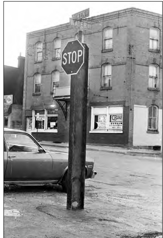
In May 1976, fed up with continually having to replace the "stop sign" at the corner of Queen and Water St., a new sign was erected, mounted on a steel "I-Beam" imbedded in solid concrete. Roads superintendant Ron MacDonald smiled, saying, "at least this way if they hit it, they'll stick around long enough for us to talk to them".
