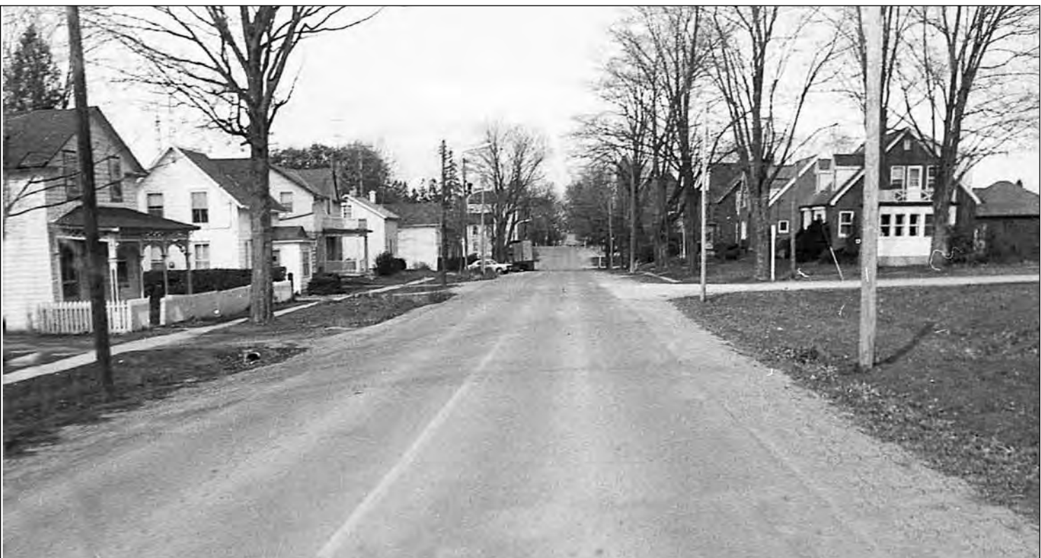
Lilla Street (now Simcoe Street), looking towards Queen Street from just north of 7A Hwy. This stretch of road was two-lanes, lined by open ditches in October 1974. The street, despite much controversy and objections, was widened to three lanes the following year.
