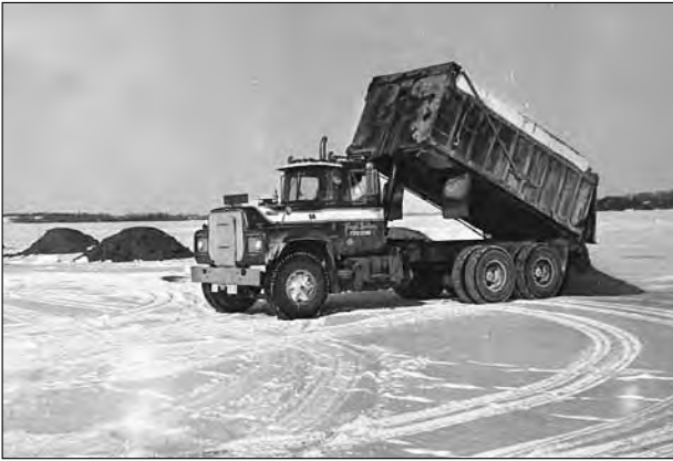
Trucks dumped more than 500 cubic yards of sand on the ice at Port Perry's waterfront in February 1979. The sand would become the base for the new Kinsmen Beach and swimming area after the ice melts and the sand settles to the bottom. The beach is a project of the Port Perry Kinsmen Club.
