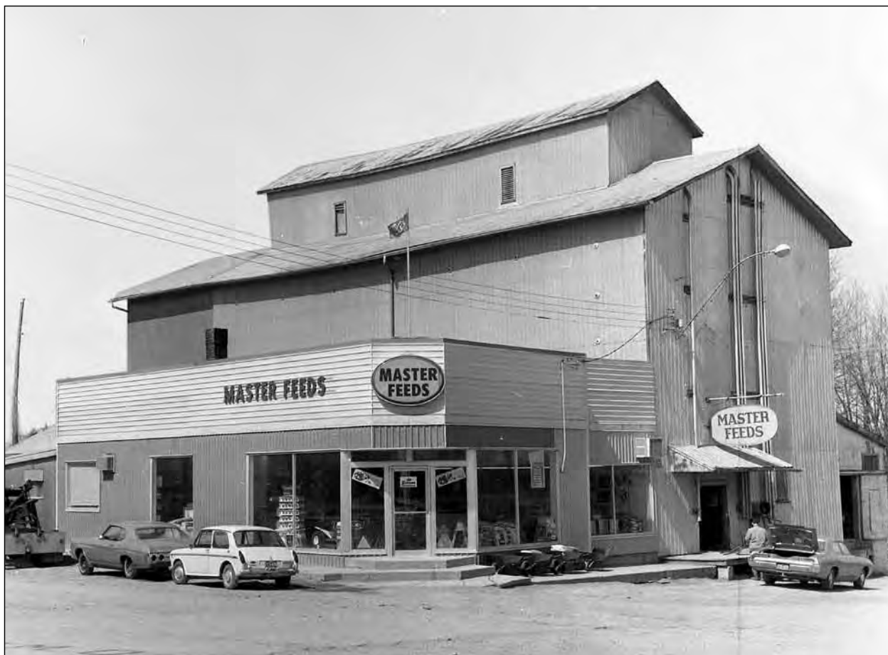
The former Currie Grain Elevator was the home of Master Feeds at the time this picture was taken in the summer of 1971.
