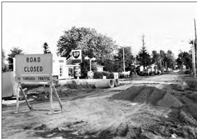
North end of Lilla Street, while under construction during summer of 1976.
