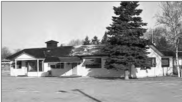
Conway Gardens restaurant, located on Hwy. 7A near the causeway, opened in July 1970 under the management of Jack Brickstock. The restaurant featured a dining room, meeting room and coffee shop.
