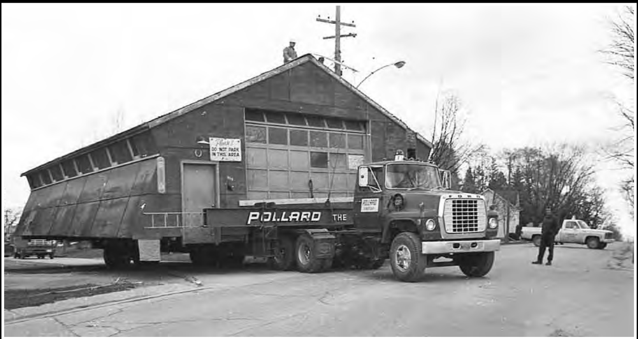
Van Camp Construction moved its 34' x 50' garage from its former location at the north end of Bigelow Street, to its new location on Vaneward Drive, just off of the Oshawa Rd, south of town in November 1974. It took 3 hours to move the garage, which they felt was worth saving.
