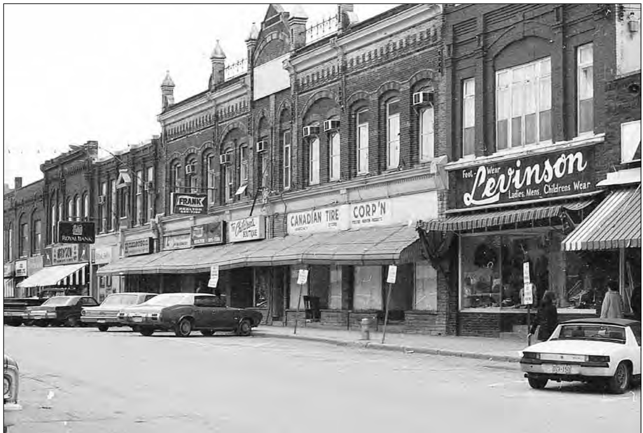
The above photograph, taken in March 1976, shows that almost every store had changed, except Levinson clothing store. Operating businesses along this stretch 16 years later included, from left, Mersco 5¢ to $1 store, the Royal Bank, Emmerson Insurance, Frank Realtor, The Children's Boutique, two stores left vacant by Canadian Tire when they moved to the Port Perry Plaza, and Levinson's store.
