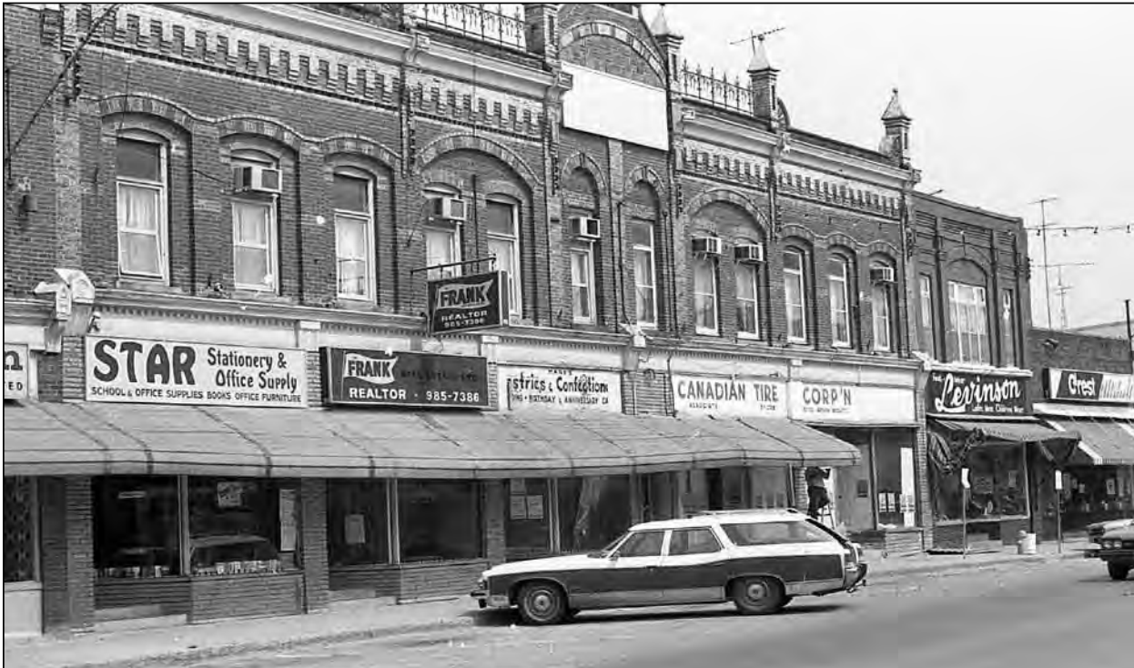
The dirty, faded yellow fibreglass awning, strung across this section of town, was just being removed in August 1976 after Canadian Tire had moved to its new location in the Port Perry Plaza. Businesses along this strip at that time included Star Stationery and Office Supply, Frank Realtor, Levinson's Dry Goods and Crest Hardware. Hank's Pastries had already moved across the street.
