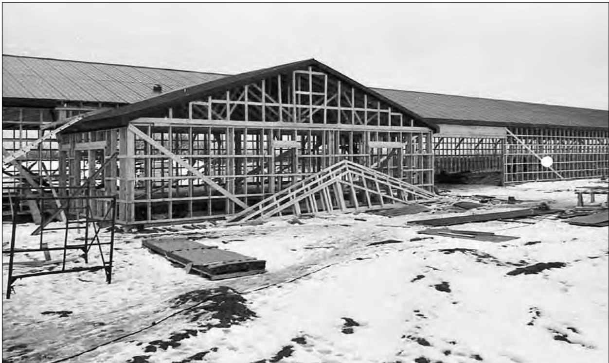
Construction was well underway in January 1975 for the new home of Lake Scugog Lumber. When finished the site will contain a 220'x50' truss plant, three storage sheds, a 6,000 sq. ft. showroom and warehouse area.
