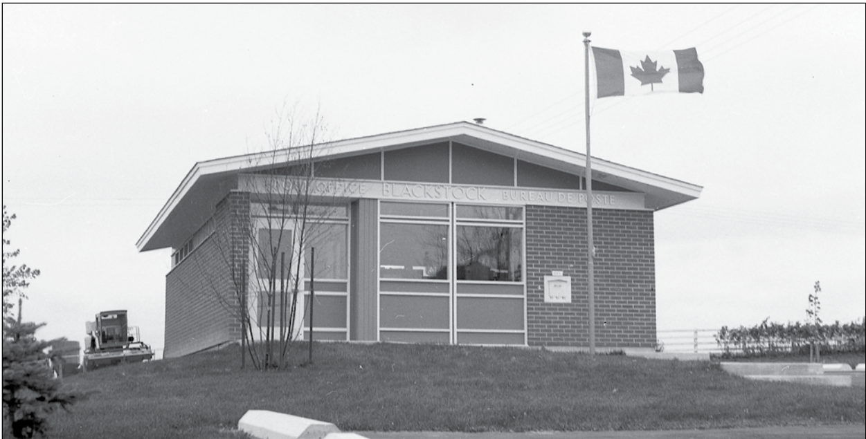
The new Blackstock Post Office building was opened in October 1968. Mrs. C. G. Venning was the postmaster .
