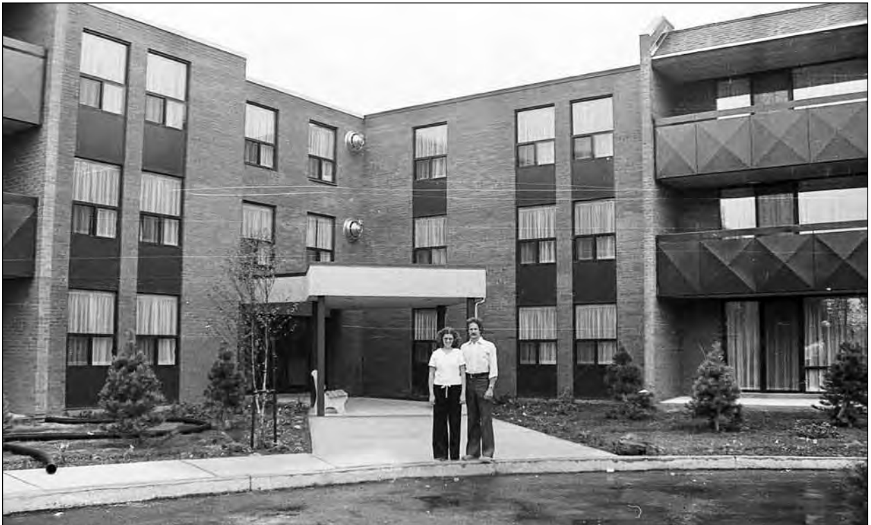
Building superintendents, Dennis and Cheryl Romeril, are seen standing in front of the entrance of the new 60 suite Carlan Apartment building, which officially opened in June 1978.
