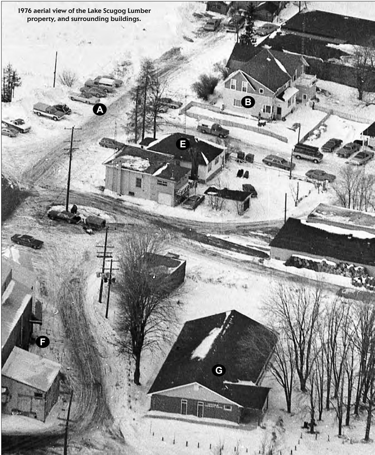
A - Water Street; B - Griffen home; C - Lake Scugog Lumber sheds; D - Lake Scugog Lumber showrooms; E - private homes; F - grain elevator;
