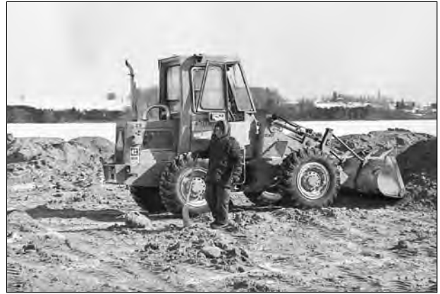
Trucks dumped more than 500 cubic yards of sand on the ice at Port Perry's waterfront in February 1979. The sand would become the base for the new Kinsmen Beach and swimming area after the ice melts and the sand settles to the bottom. The beach is a project of the Port Perry Kinsmen Club.
