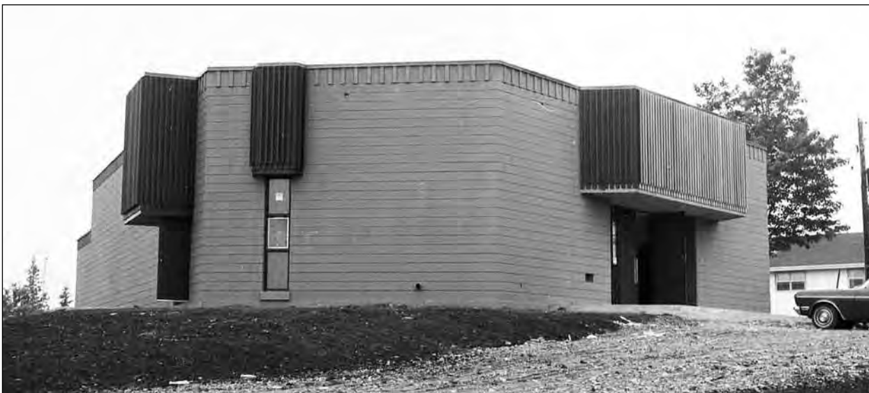
The new Roman Catholic Immaculate Conception Church under construction in June 1968.
