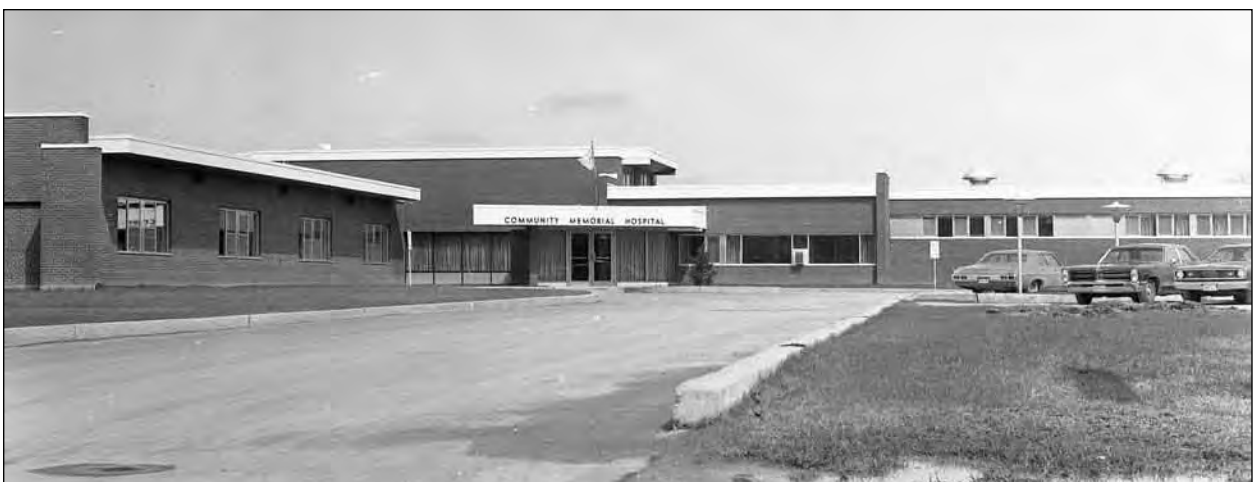
Entrance to Port Perry Community Memorial Hospital in June 1972.
