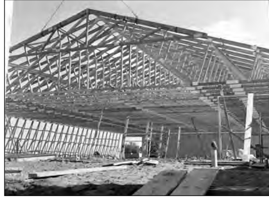
Construction was well underway on Peel's Poultry Farm's new hatchery in September 1966. The building is 190' x 94' and the trusses for the roof system are 94' long and weight approximately one ton each. Each truss was built in three sections at the Lake Scugog Lumber plant and assembled on site before being lifted into place by a large crane.
