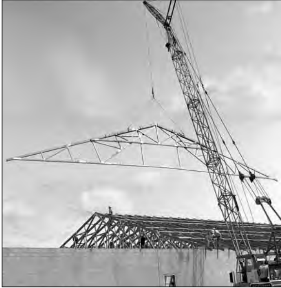
Construction was well underway on Peel's Poultry Farm's new hatchery in September 1966. The building is 190' x 94' and the trusses for the roof system are 94' long and weight approximately one ton each. Each truss was built in three sections at the Lake Scugog Lumber plant and assembled on site before being lifted into place by a large crane.
