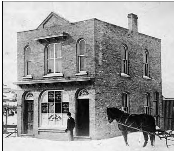
Port Perry Post Office, Queen and John Street.
