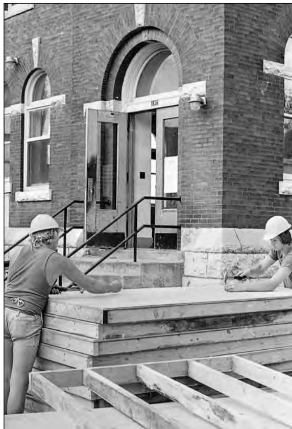
Construction underway on post office in November 1974.
