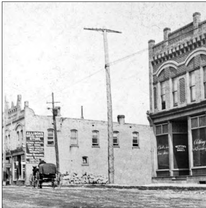
The wooden fence had been removed when this picture was taken on Queen Street, about 1911, before post office construction got underway.
