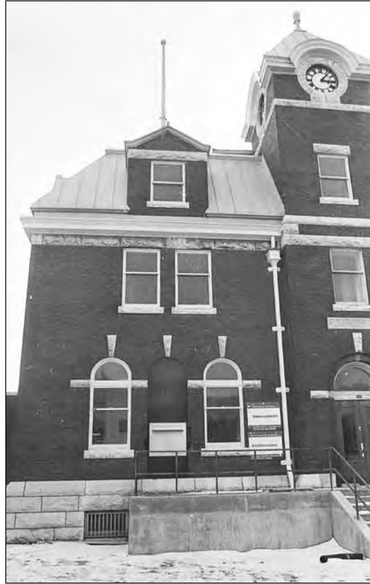
During renovations, the platform was extended over to the letters box between to the windows, eliminating the steps
